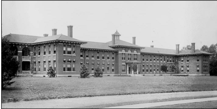
Figure 6.22. Building Q circa 1910. (Library of Congress National Photo Company Collection)
