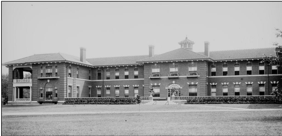
Figure 6.12. Either Building B or Building C circa 1910. Buildings B and C were largely identical buildings that flanked either side of Building A. (Library of Congress National Photo Company Collection)
