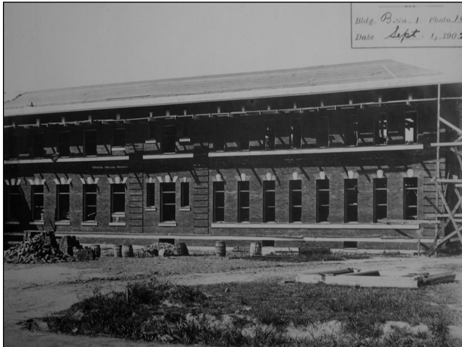
Figure 6.8. Building B under construction, September 1902. (National Archives RG 48 Entry 300 Box 6)
