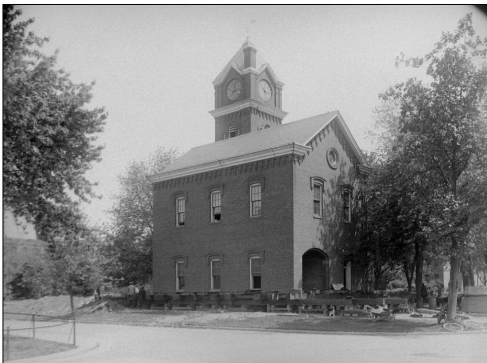
Figure 7.7. The firehouse in 1905 being prepared to be moved. (See also Figure 7.5) (National Archives RG 418-G-110)
