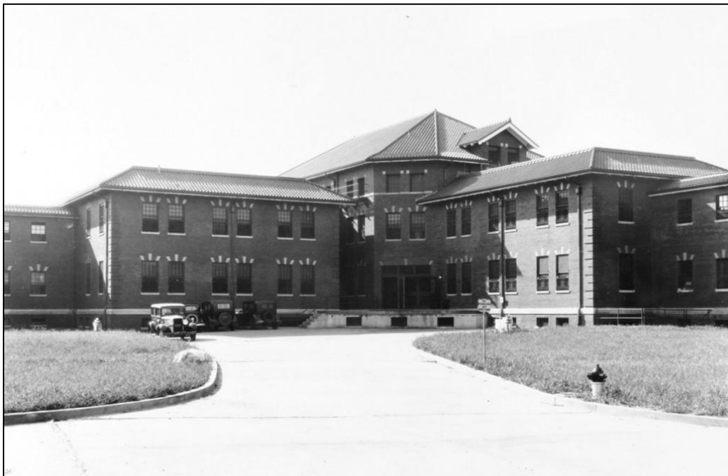
Figure 8.3. The central kitchen for the CT building complex flanked by two dining room wings and connecting wings to patient wards. (National Archives RG 418-P-68)
