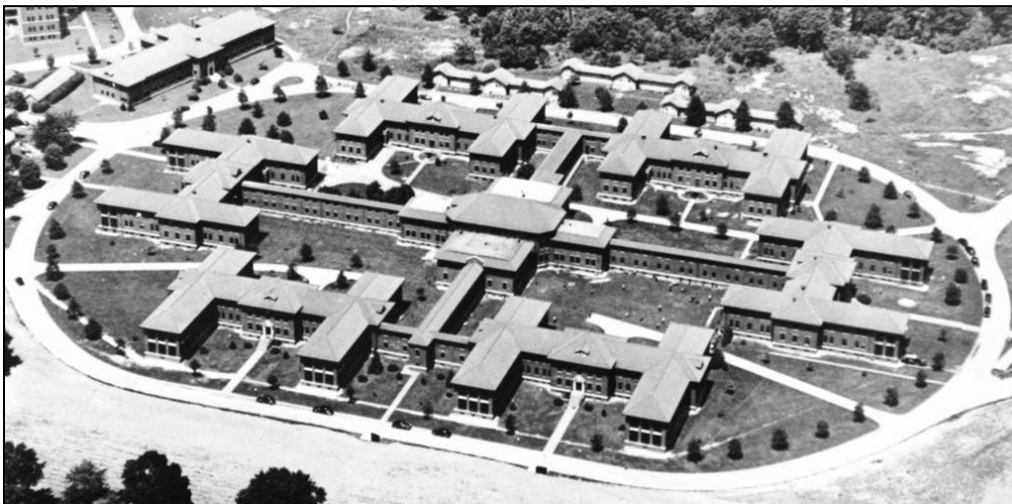
Figure 8.5. The completed CT building complex. Note the central kitchen and dining rooms at center. The Tuberculosis Building can be seen in the upper left and the three wooden temporary tuberculosis buildings can be seen at the top of the image. (National Archives RG 418-P)
