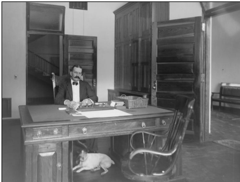
Figure 7.10. Supervisor's office in Building B in 1905. (National Archives RG 418-G-42)
