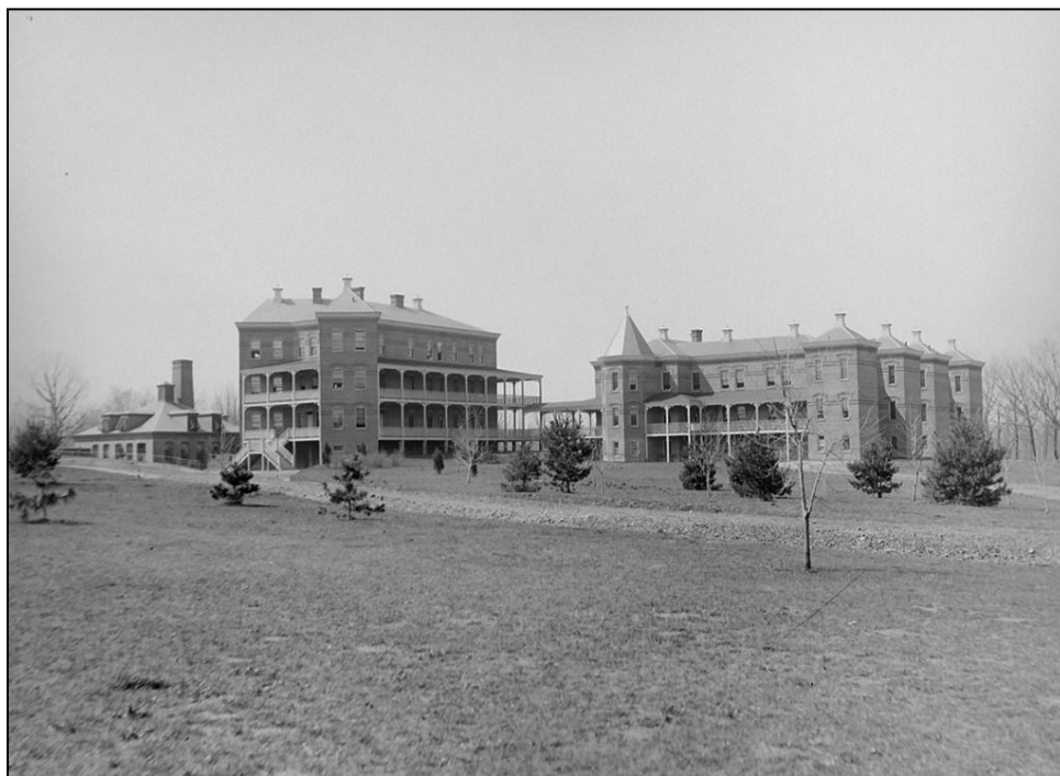
Figure 4.15. Oaks Buildings I and II built for white male epileptics. Note the detached kitchen for the Toner Building on the left of the image. (National Archives RG 418-G-200)
