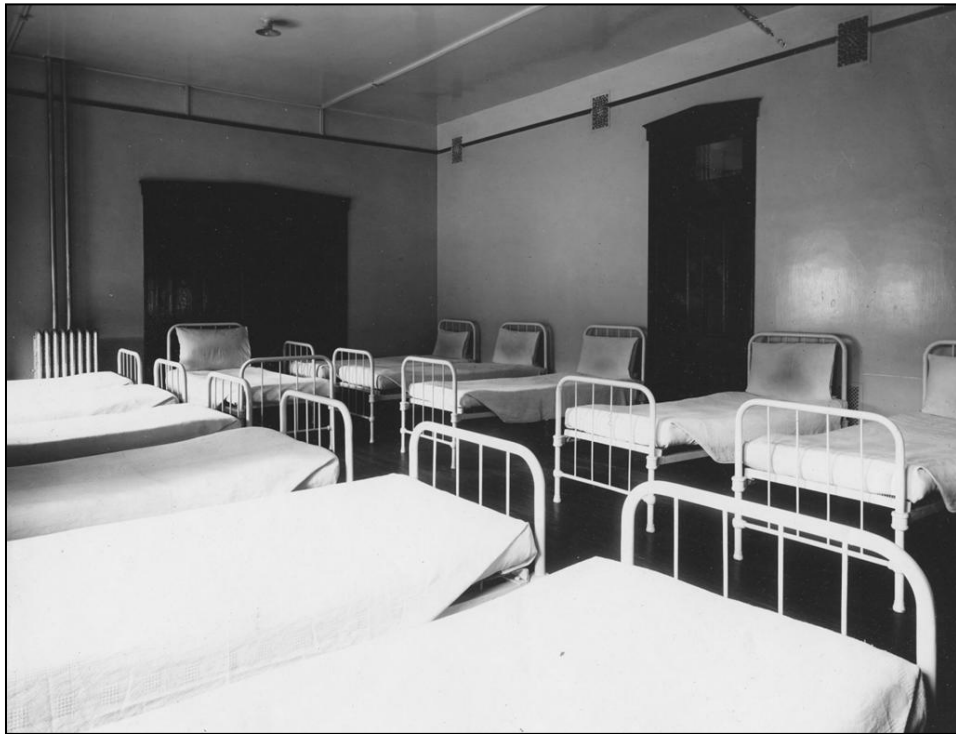
Figure 4.10. Typical dormitory room in Home Building. (National Archives RG 418-P-132)
