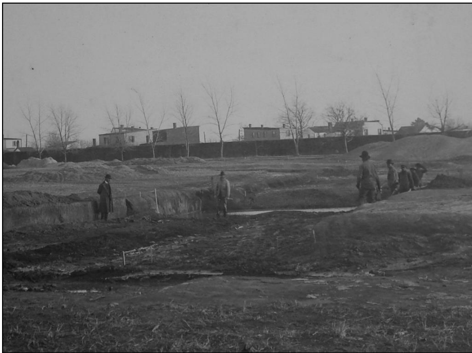
Figure 6.3. Patients digging foundations for the Shepley, Rutan & Coolidge buildings circa 1902. (National Archives RG 48 Entry 300 Box 6)
