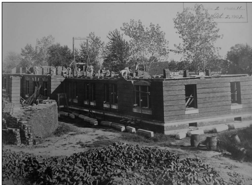
Figure 6.6. Building E under construction, October 1902. (National Archives RG 48 Entry 300 Box 6)
