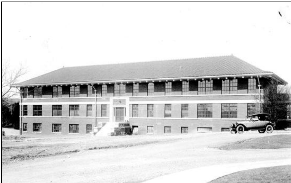
Figure 7.17. Blackburn Laboratory circa 1925. (National Archives RG 418-G-58) (See Figure 8.14 for site plan.)
