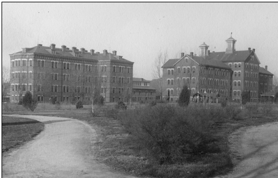
Figure 4.9. Looking from the southeast to the Home Building on the left and the Relief Building on the right circa 1897. Note the Detached Dining Hall in between the two buildings. (National Archives RG 418-P-550)
