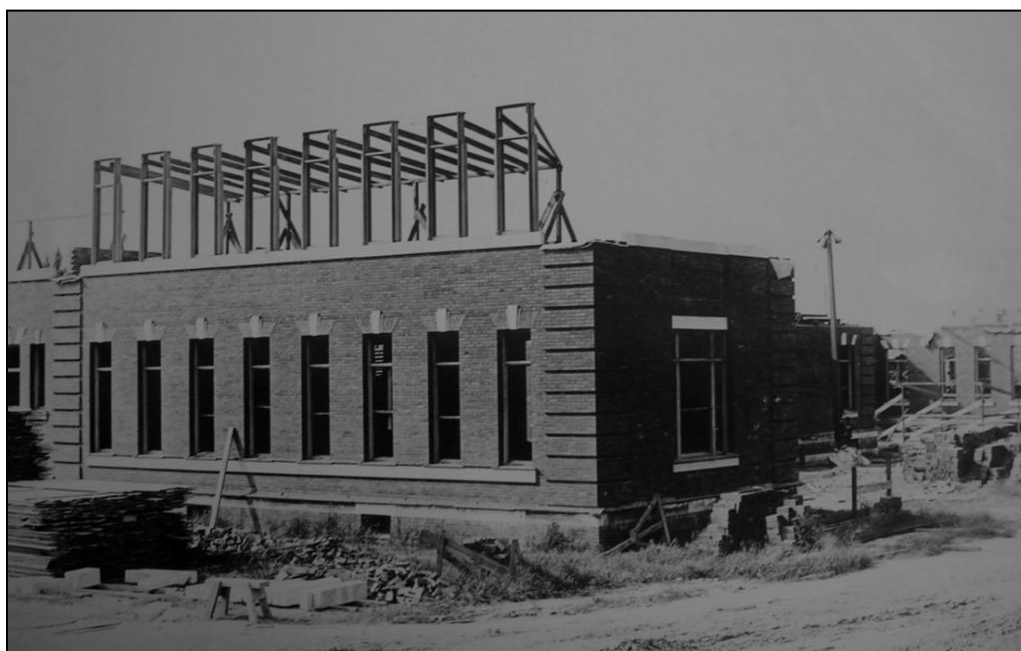
Figure 6.7. Building C under construction, September 1902. (National Archives RG 48 Entry 300 Box 6)
