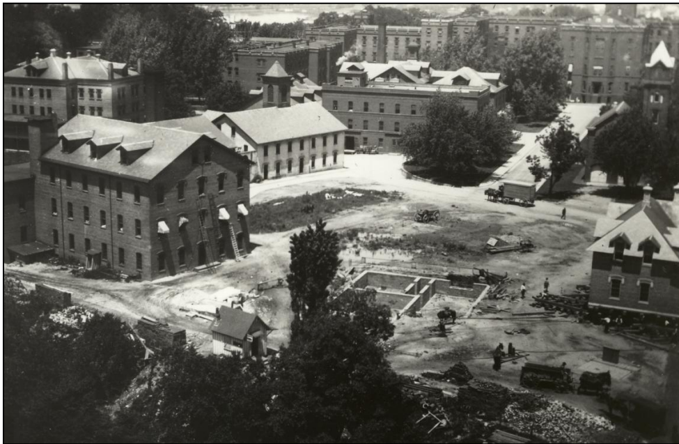
Figure 7.5. The Rest (at right) being moved toward its new foundation in 1905. The bell tower of the firehouse can be seen at the top right of the image prior to its move to a location just this side of the horse and wagon. (National Archives RG 418-P)
