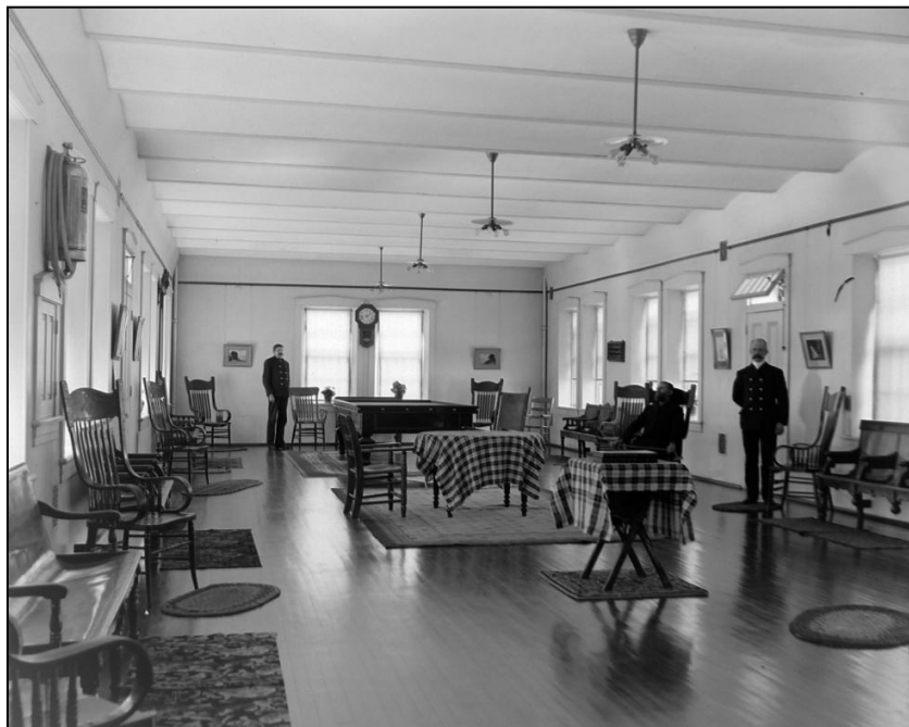
Figure 4.4. Day room on first floor of Atkins Hall after renovations circa 1900. (National Archives RG 418-G-27)
