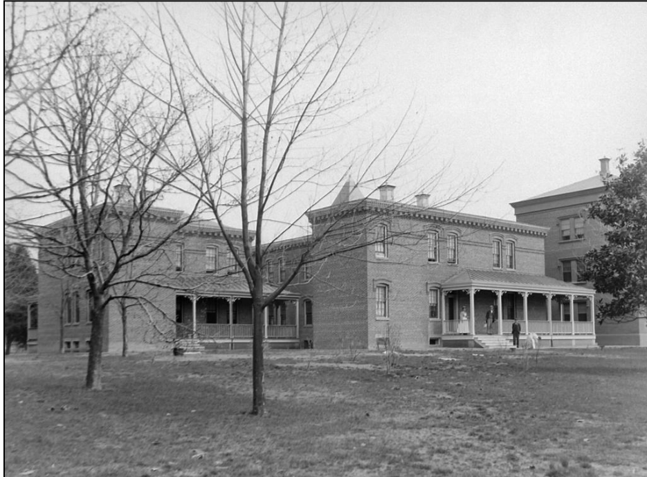
Figure 4.13. Looking southeast toward Dix 2 (later Linden ward) on the far left, Dix 1 (later Holly ward) in the middle, and the East Lodge at the far right. The Dix buildings were built in 1893 for white female epileptics. (National Archives RG 418-G-109)
