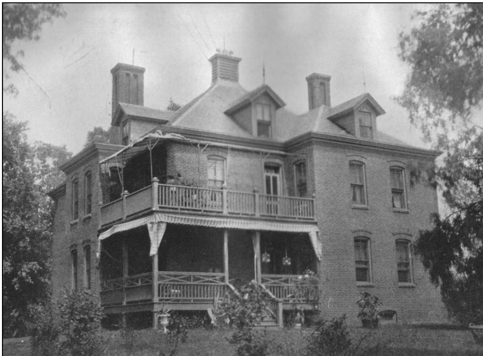
Figure 5.22. Borrows Cottage, completed in 1881, as shown in the 1898 Annual Report. 105
