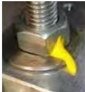
Marked nut and washer for torque audit
