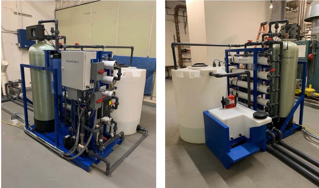
Figure 2: BDR system installed at the Lloyd D. George U.S. Courthouse
