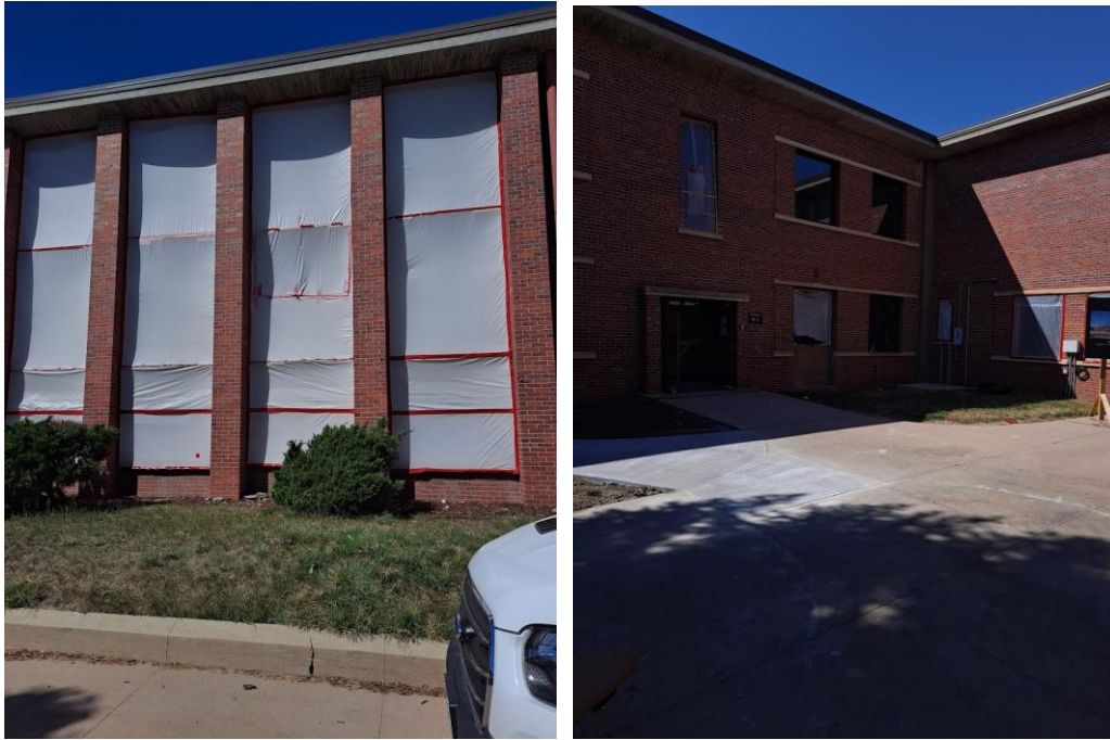
Figure 2. Denver Federal Center Building 40.
