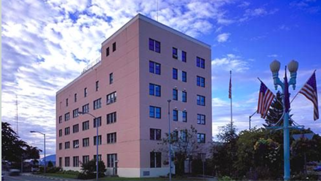
NREL assessed a biomass boiler at the Federal Building, Ketchikan, AK
