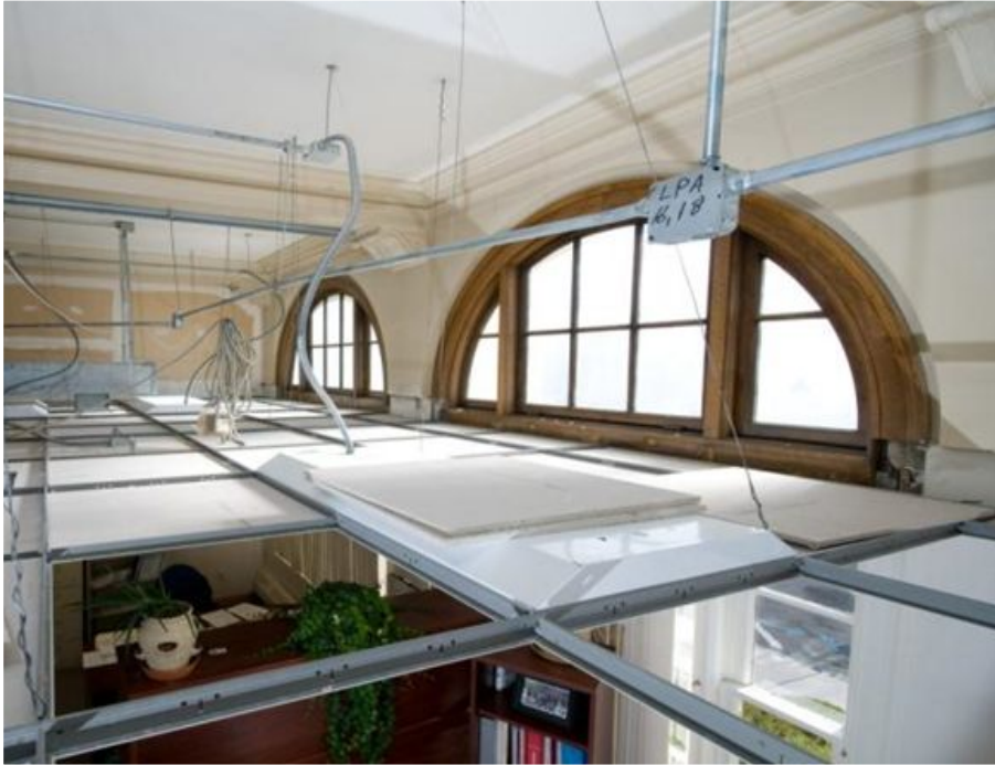
Dropped ceilings & ductwork in old postal lobby of Wayne Aspinall FB
