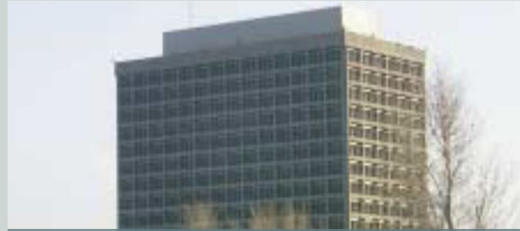
Building 67 Domestic Hot Water Recirculation Pumps
