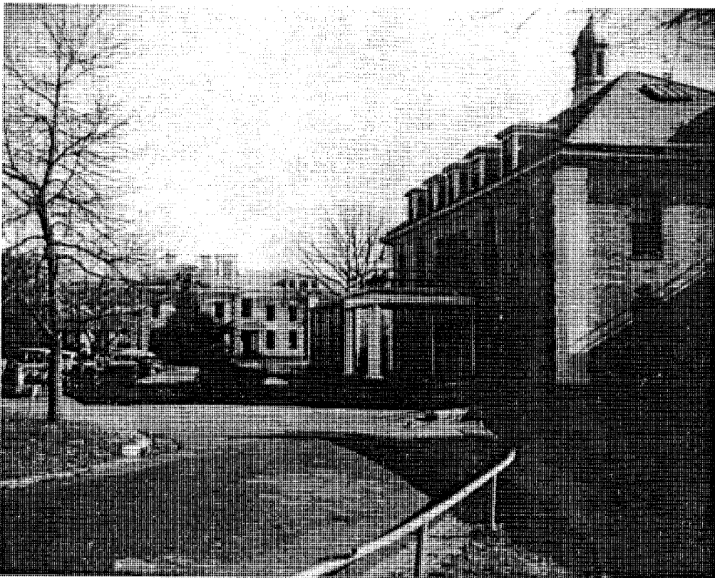
Figure 2-3 HOSPITAL (BUILDING 3) North and west elevations of administrative building, ca., early 1940's BUMED Archives
