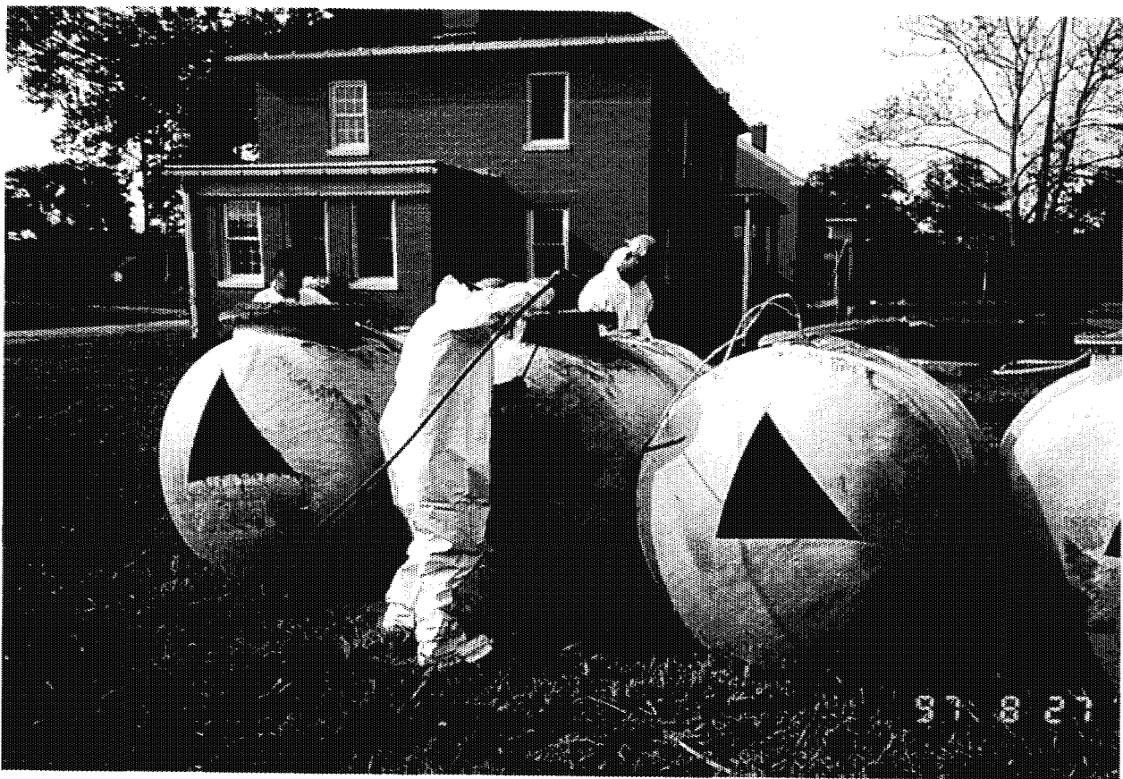
Photograph No.: 5 Contract No.: DACW31-95-D-0097 Location: Pedricktown U.S. Army Reserve Center (Bldg 276N) Photographer: B. Rayfield Description: Tanks cleaned using pressure washer.
