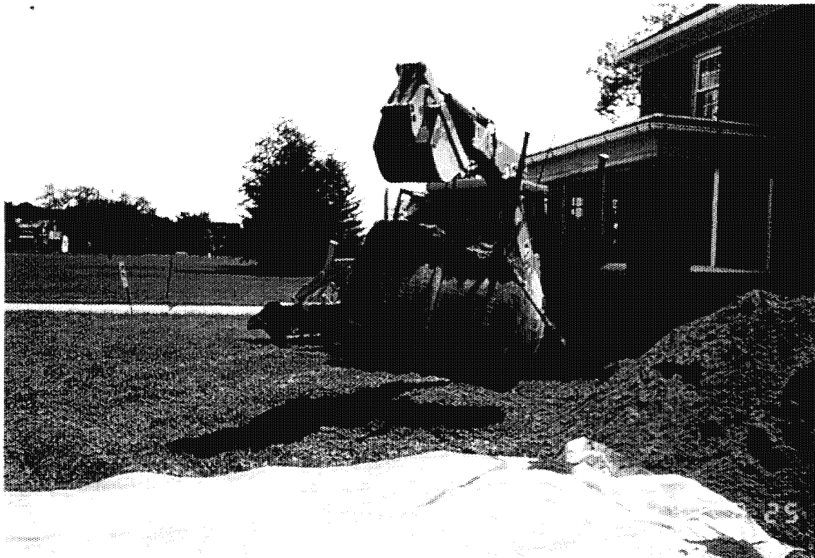
Photograph No.: 2 Contract No.: DACW31-95-D-0097 Location: Pedricktown U.S. Army Reserve Center (Bldg 276N) Photographer: B. Rayfield Description: 550-gallon UST being removed from ground.
