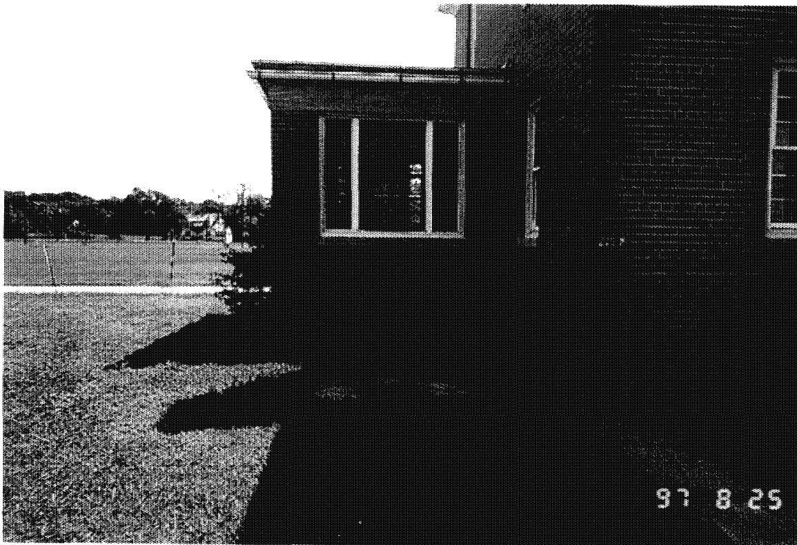
Photograph No.: 1 Contract No.: DACW31-95-D-0097 Location: Pedricktown U.S. Army Reserve Center (Bldg 276N) Photographer: B. Rayfield Description: Building 276N before tank removal activities.
