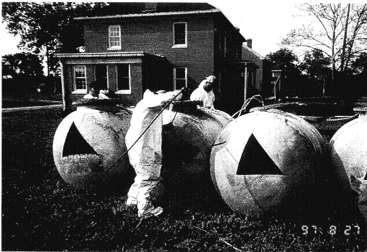
Photograph No.: 3 Contract No.: DACW31-95-D-0097 Location: Pedricktown U.S. Army Reserve Center (Bldg 277N) Photographer: B. Rayfield Description: Tanks cleaned using pressure washer.
