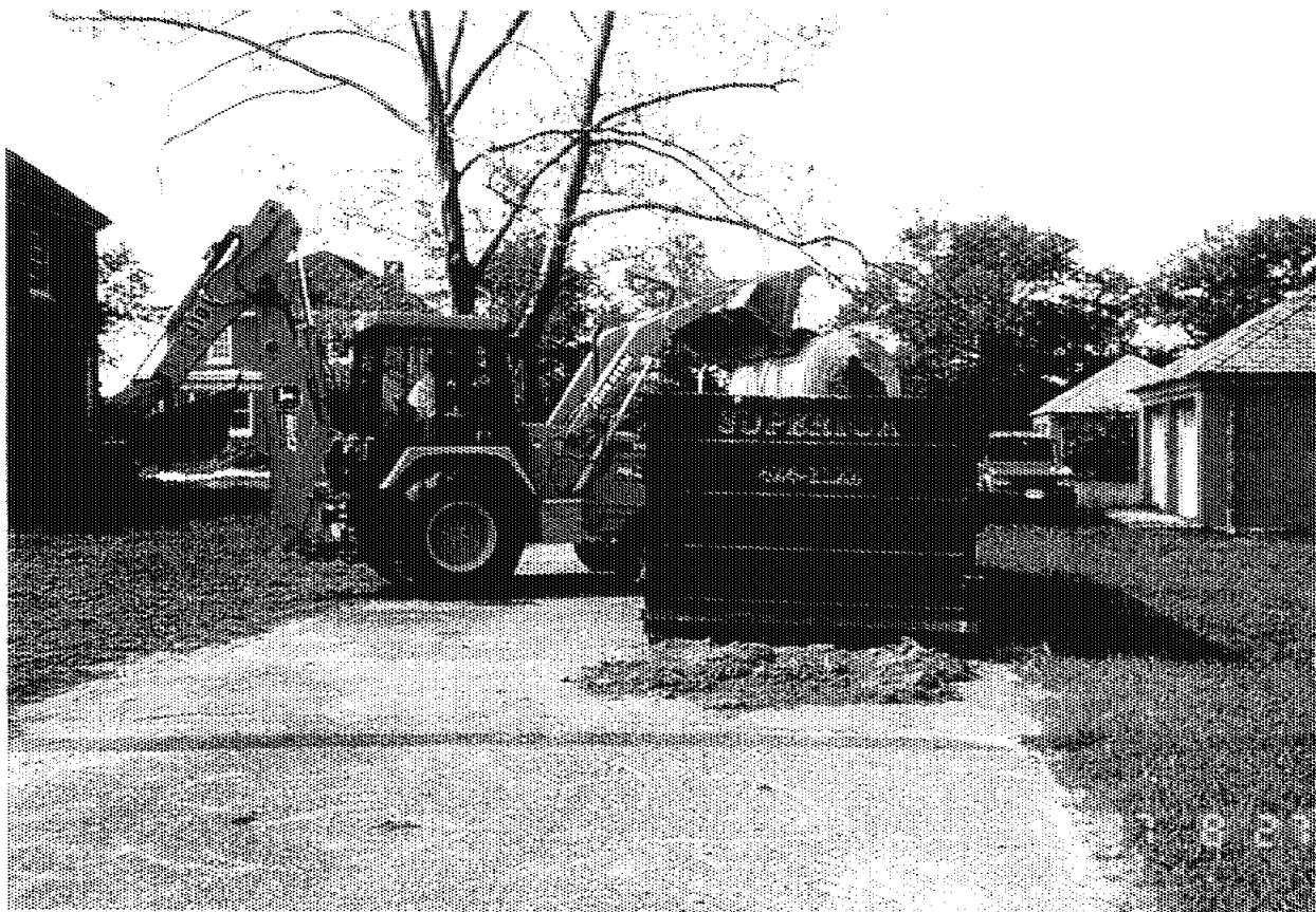
Photograph No.: 5 Contract No.: DACW31-95-D-0097 Location: Pedricktown U.S. Army Reserve Center (Bldg 277N) Photographer: B. Rayfield Description: Tank was loaded into rolloff box for disposal.
