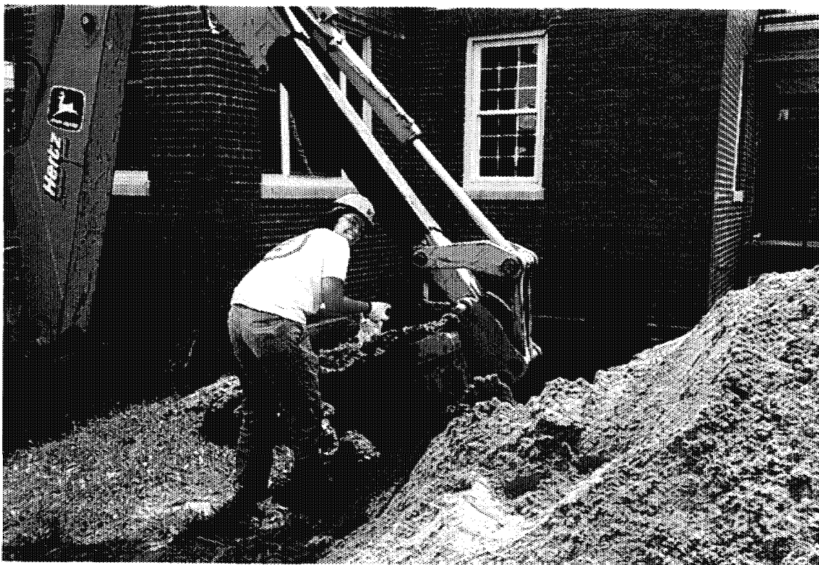
Photograph No.: 4 Contract No.: DACW31-95-D-0097 Location: Pedricktown U.S. Army Reserve Center (Bldg 276N) Photographer: B. Rayfield Description: Four ventilation soil samples were collected from tank excavation. View: Detail.
