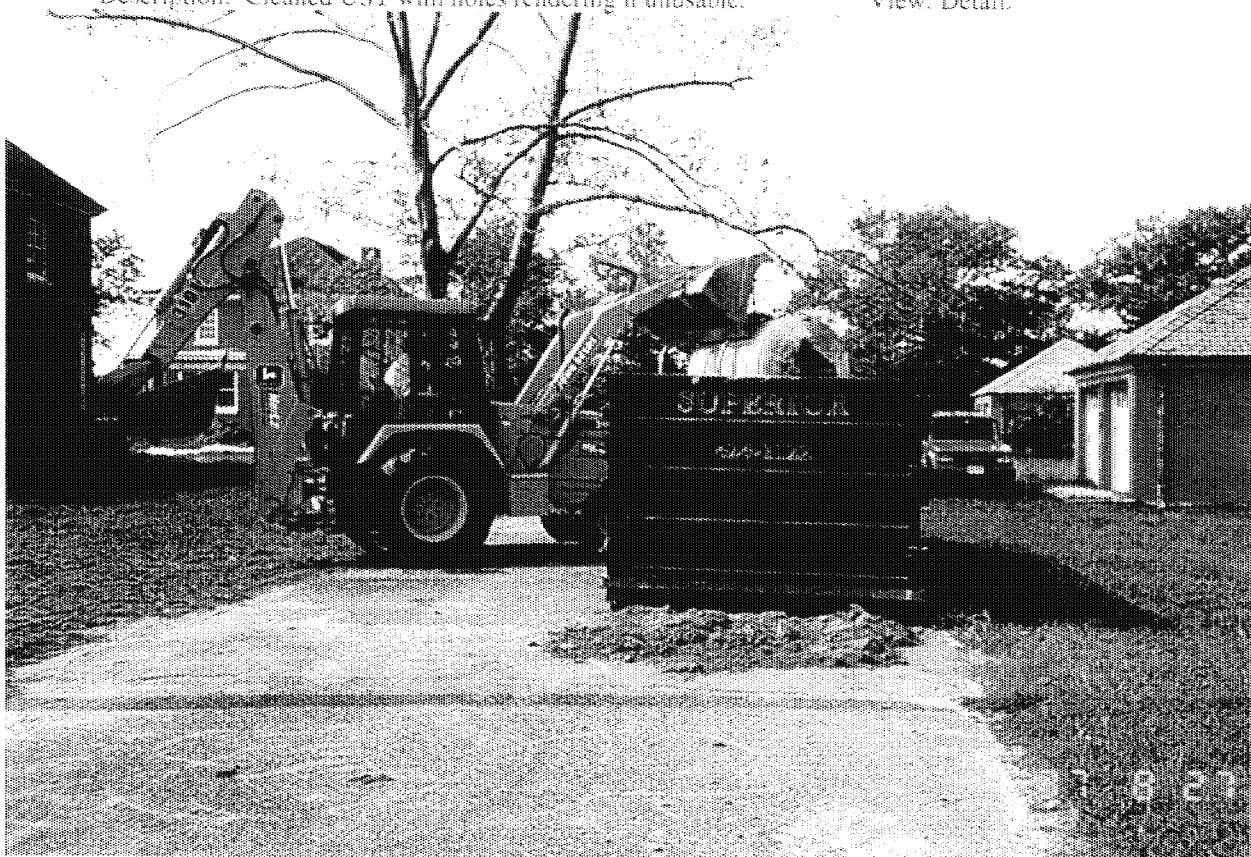
Photograph No.: 6 Contract No.: DACW31-95-D-0097 Location: Pedricktown U.S. Army Reserve Center (Bldg 276S) Photographer: B. Rayfield Description: Tank was loaded into rolloff box for disposal.
