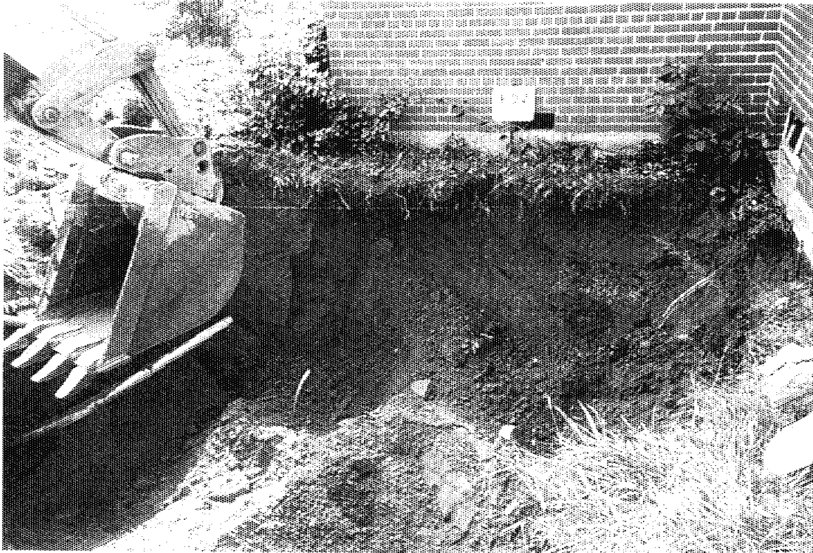
Photograph No.: 2 Contract No.: DACW31-95-D-0097 Location: Pedricktown U.S. Army Reserve Center (Bldg 277N) Photographer: B. Rayfield Description: Excavation after tank removal.
