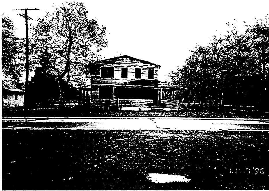
Figure 10. Section C of the Project Area. View facing east.
