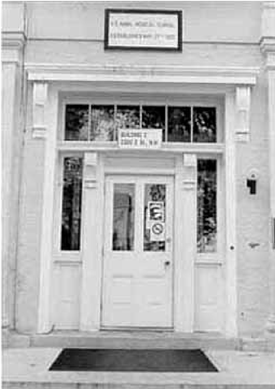
Figure 67 Old Naval Observatory (1844) North Elevation. Entry detail.
