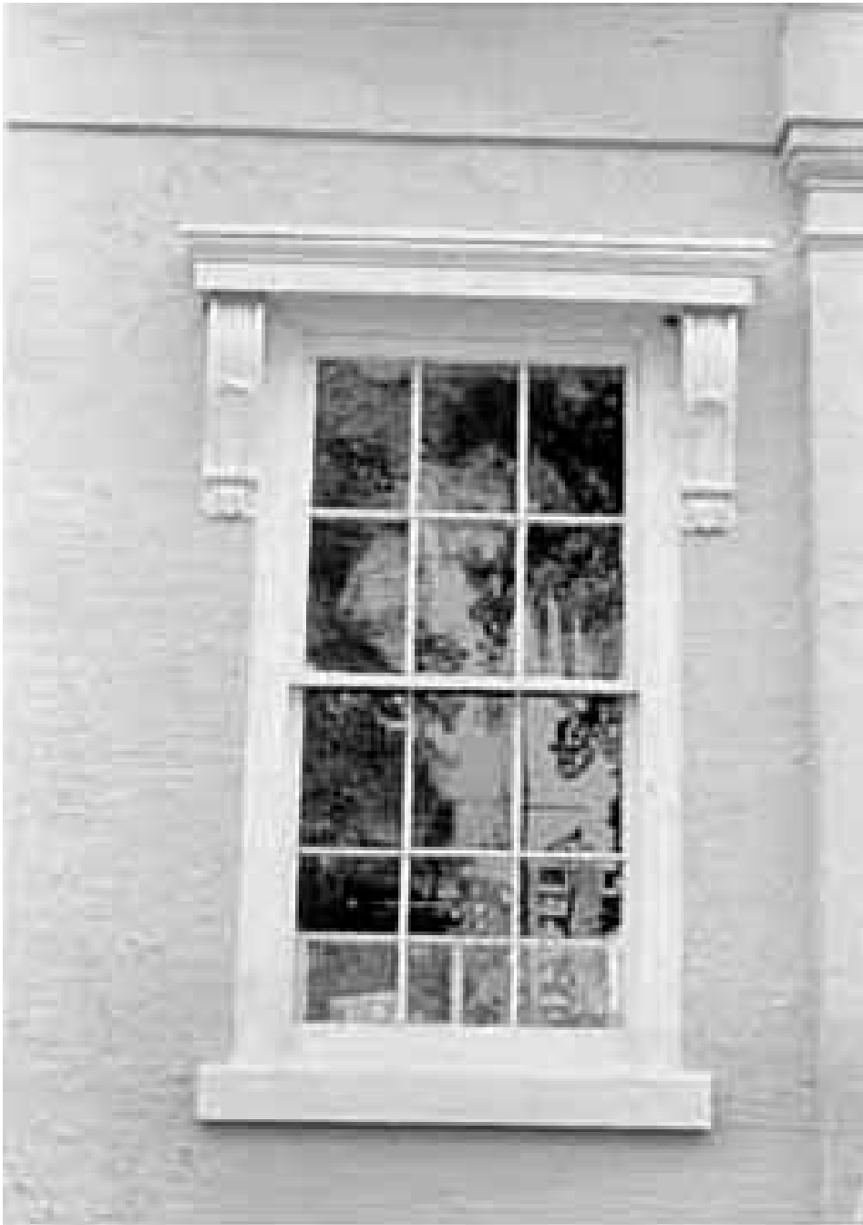
Figure 69 Old Naval Observatory (1844) Six-over-six windows with bracketed hoods are typical throughout the 1844 structure.
