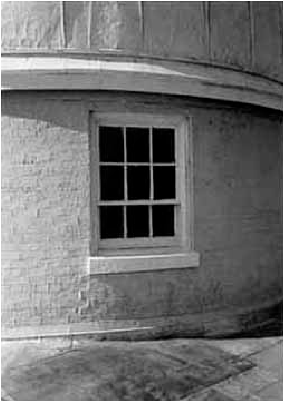
Figure 80 Old Naval Observatory (1844) Detail of drum showing window, which was originally a door to the roof.
