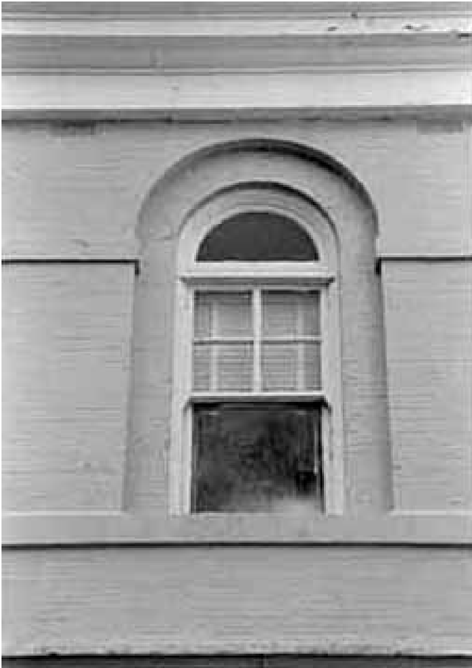
Figure 72 Old Naval Observatory (1844) Arched window typical of the second story additions.
