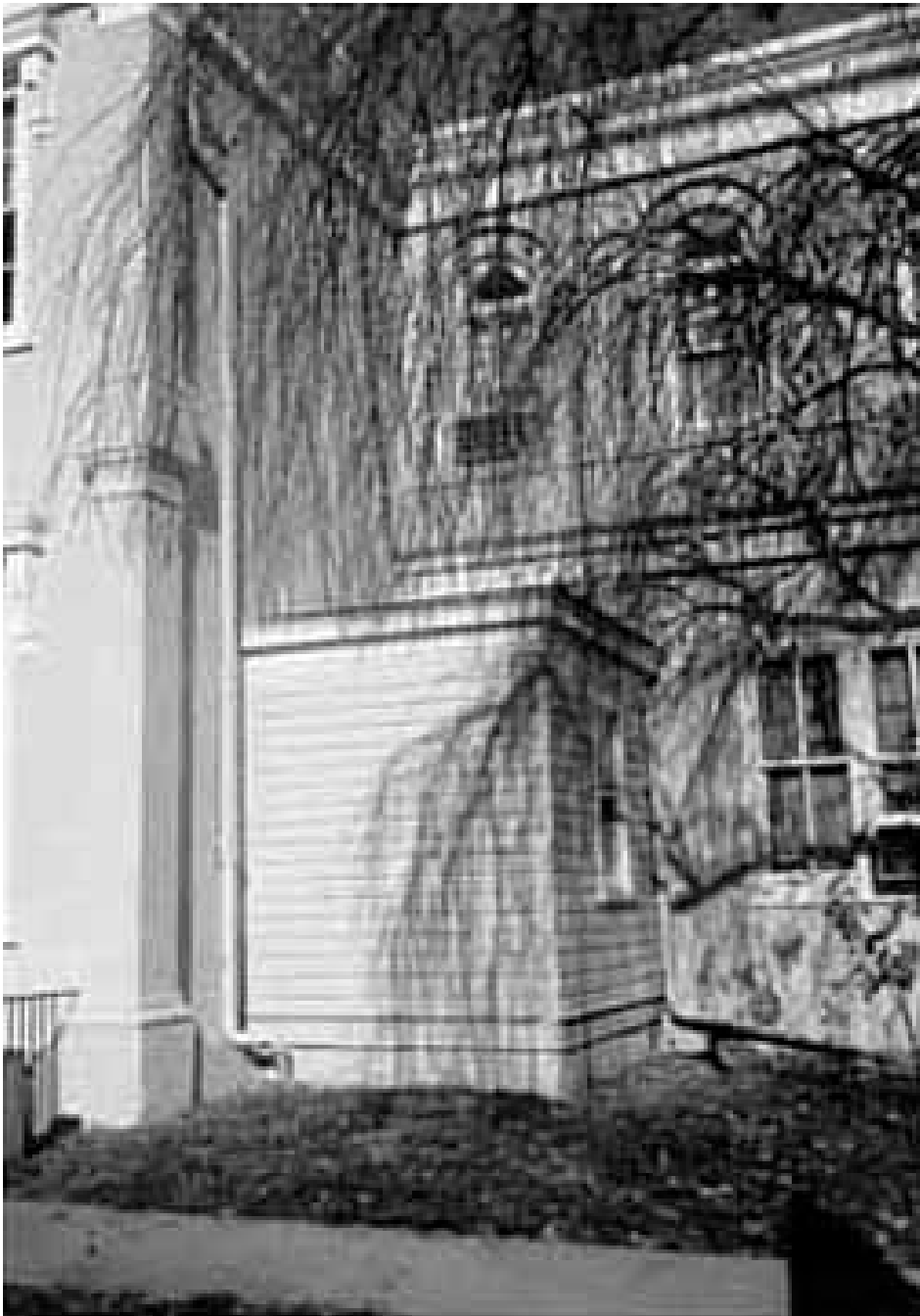
Figure 77 Old Naval Observatory (1844) South Elevation. Wood toilet addition ca. 1920.
