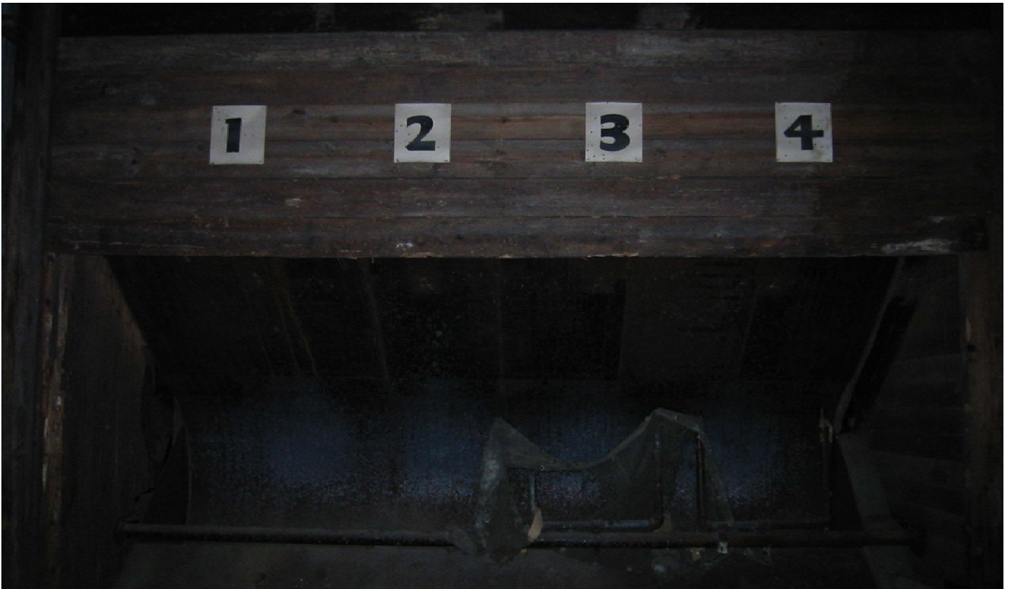
Photograph 2. Building 105 SAFR. Bullet Pit, September 2002.
