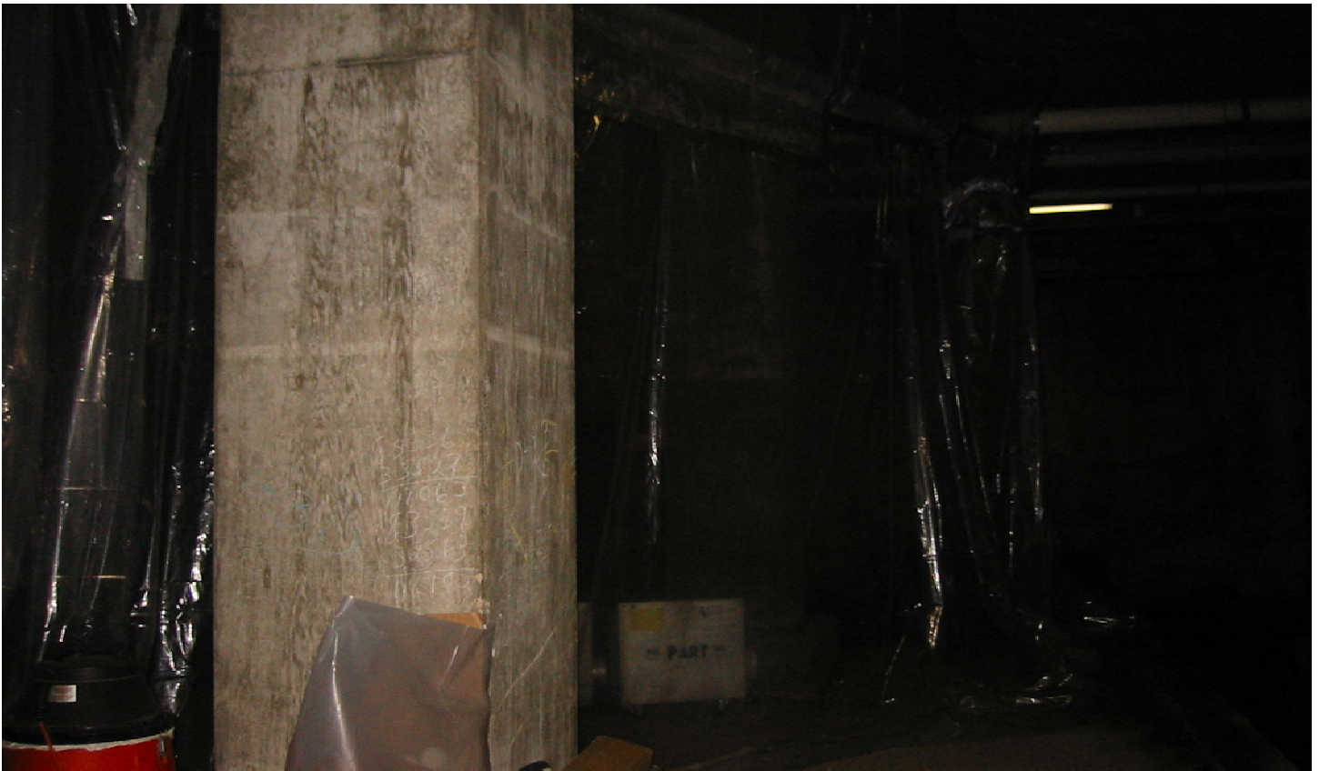
Photograph 7. Building 105 SAFR. Column at right hand (NE) corner of containment, September 2002.
