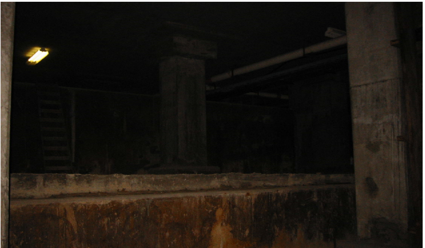
Photograph 4. Building 105 SAFR. Ledge above Bullet Pit to the left, September 2002.
