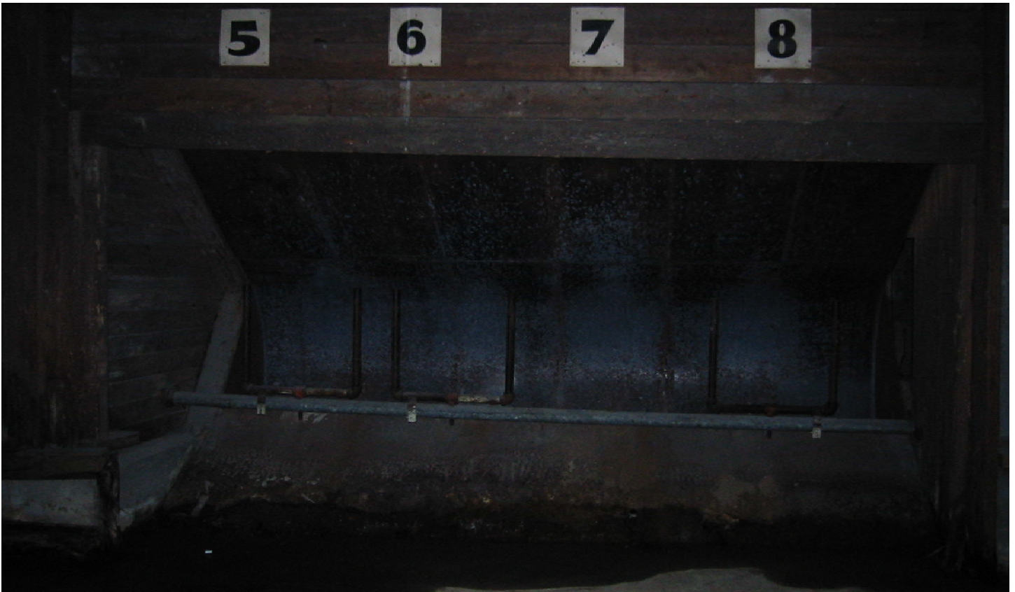
Photograph 1. Building 105 SAFR. Bullet Pit, September 2002.
