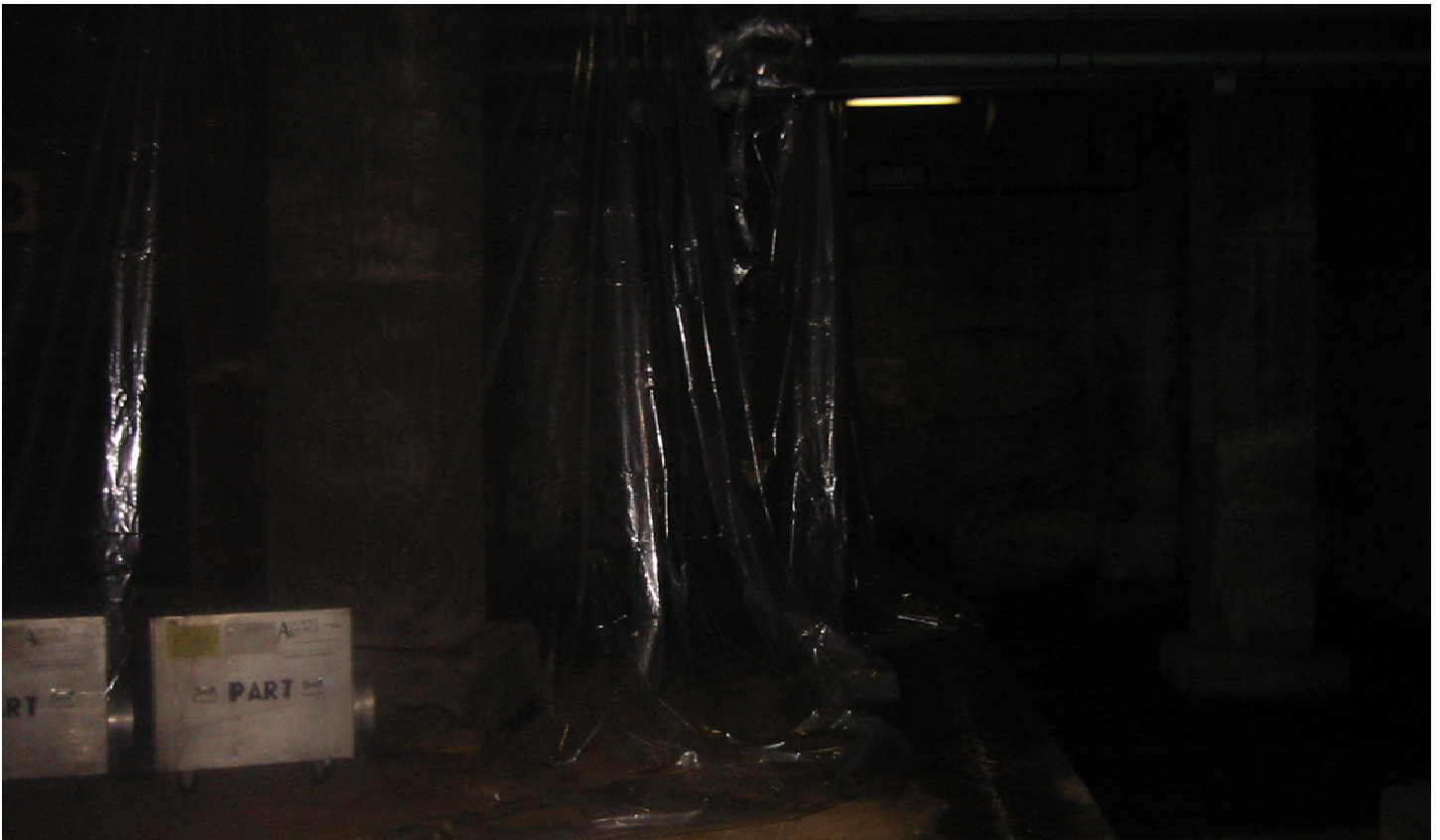
Photograph 6. Building 105 SAFR. Plastic sheeting containment with clean air HEPA filters at left, September 2002.
