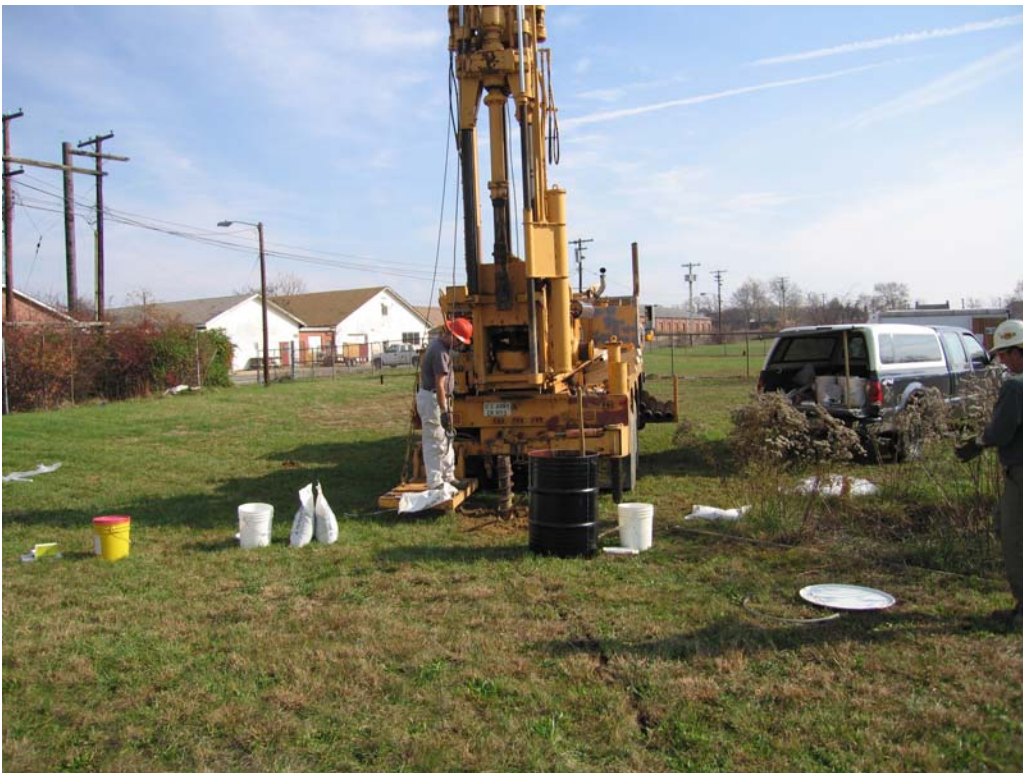
Photo G-6. Drilling at the 12-MW-03 location.
