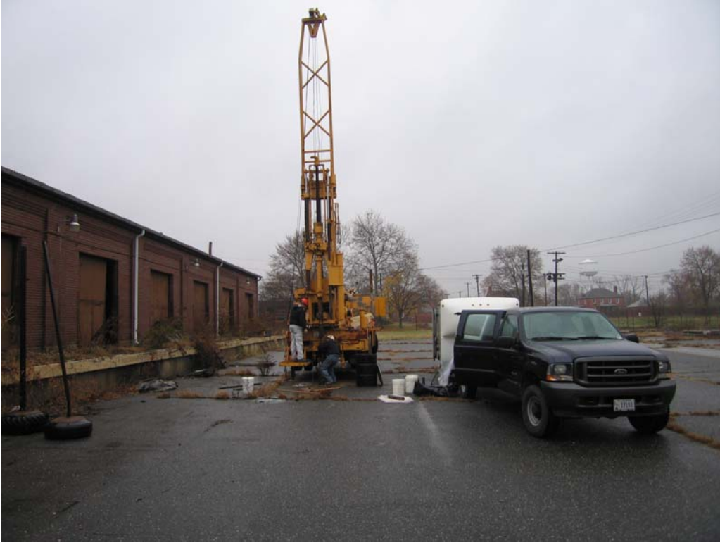
Photo G-1. Set up and drilling at monitoring well 434-MW-01 location.
