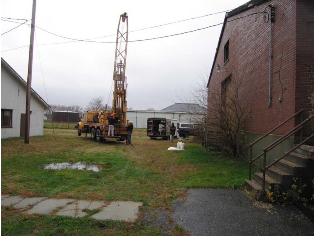
Photo G-3. Drilling at 434-MW-02 location.
