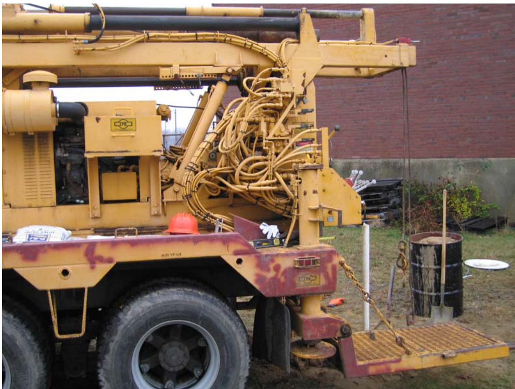
Photo G-4. Complete drilling and well installation at 434-MW-02 location.
