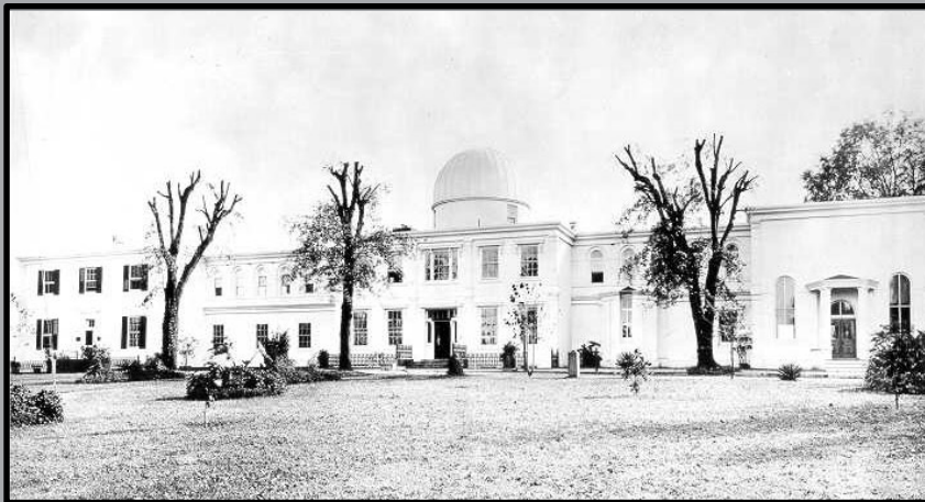
View of Building 2 and Maury Circle, 1935
