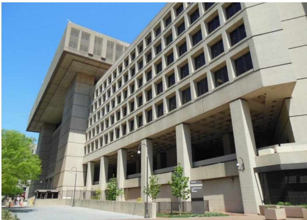
Figure 62 - West facade along 10th Street (Source: QEA, 2013)
