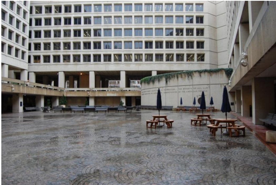
Figure 65 - Courtyard (Source: QEA, 2013)
