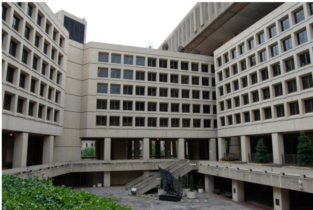
Figure 66 - Courtyard (Source: QEA, 2013)
