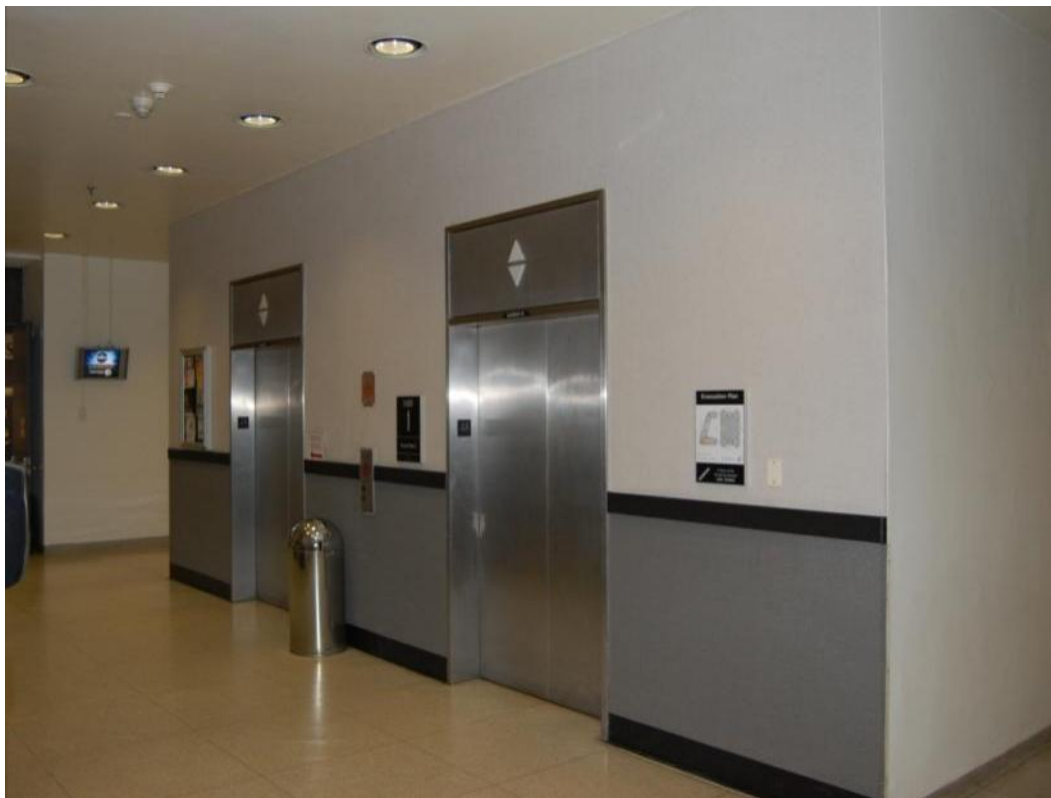
Figure 77 - Typical elevator lobby (Source: QEA, 2013)
