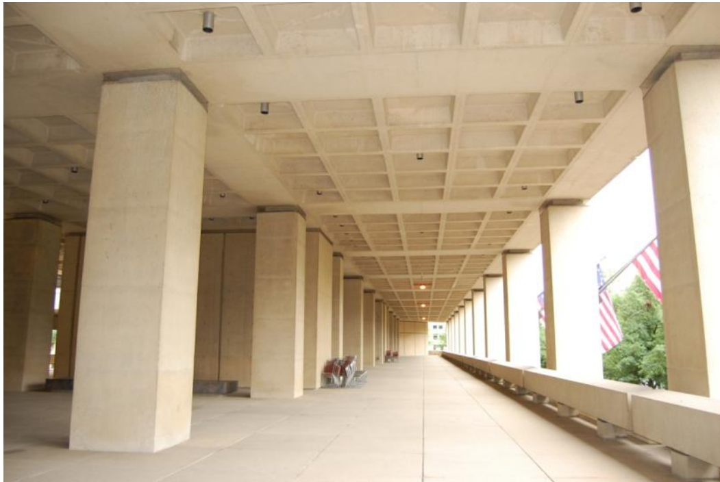
Figure 63 - Second floor terrace (Source: QEA, 2013)
