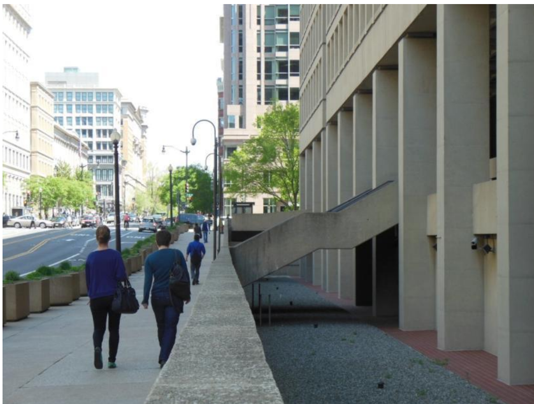
Figure 64 - East view along E Street (Source: QEA, 2013)
