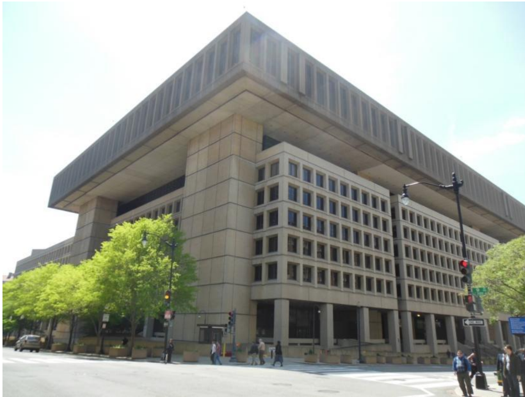
Figure 61 - Northwest corner of building at E and 9th Streets (Source: QEA, 2013)
