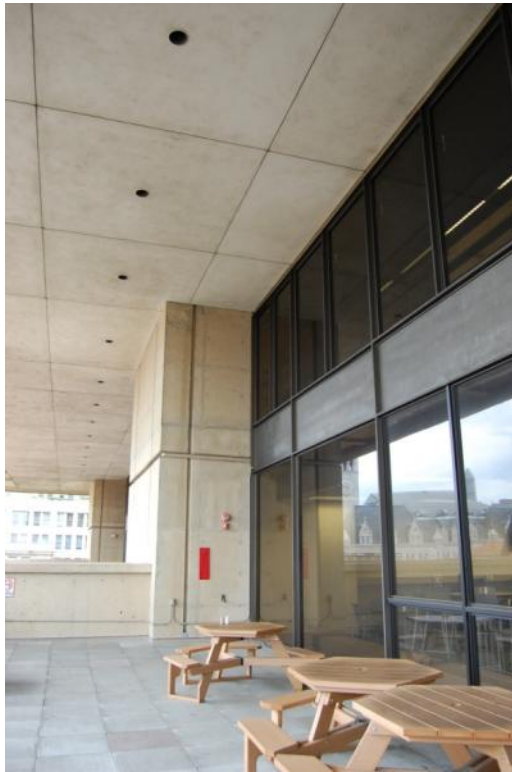
Figure 81 - Roof deck off of the cafeteria (Source: QEA, 2013)
