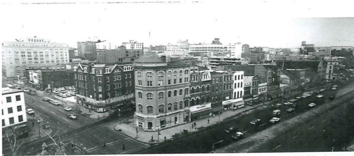
Figure 13 - View of the two blocks bounded by Pennsylvania Avenue, 9th and 10th Streets prior to demolition for the FBI Building (Source: GSA Regional Office Archives)
