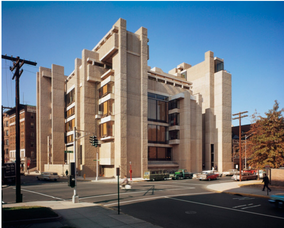
Figure 47 - Art and Architecture Building, Yale University, New Haven, Connecticut (Source: AIA.org)
