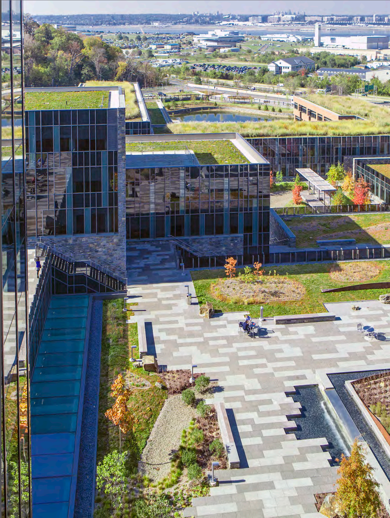
Figure 4: U.S. Coast Guard Headquarters Courtyard Washington, DC
