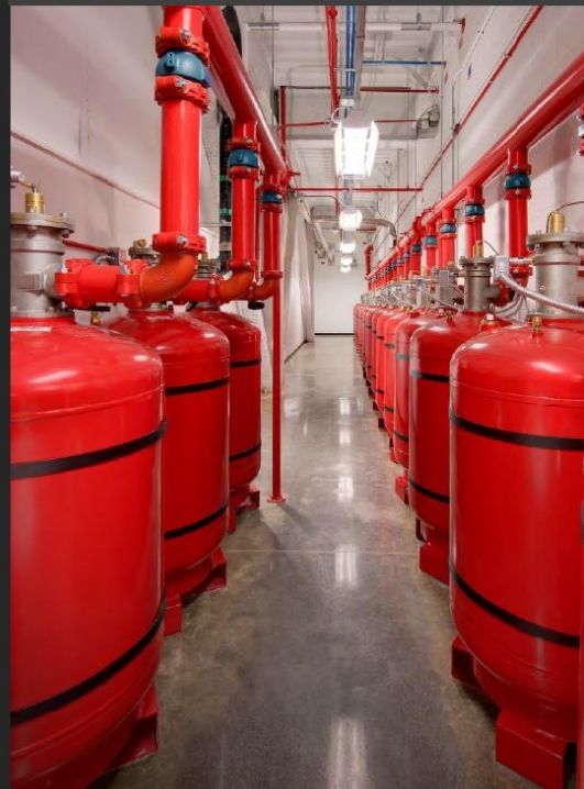
Figure 15: National Support Center Social Security Administration Frederick, MD
