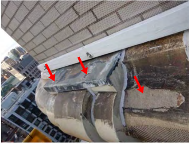
Photo 1: Seal cap anchors + seal terracotta + R/S
