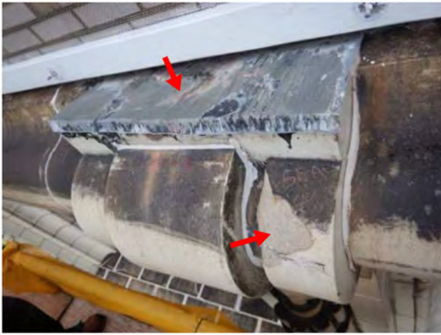
Photo 1: New tapcons to secure cap + seal terracotta
