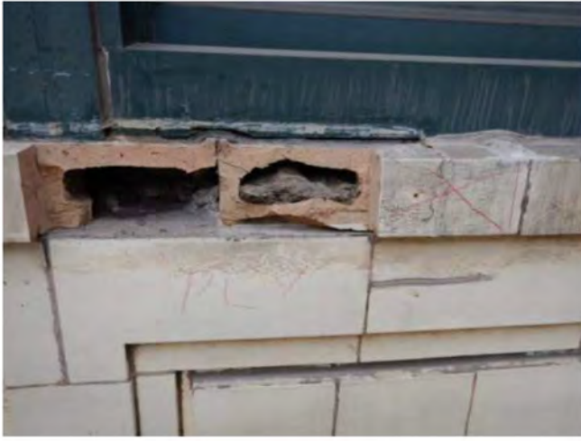
Photo 45: Remove loose & install plywood
