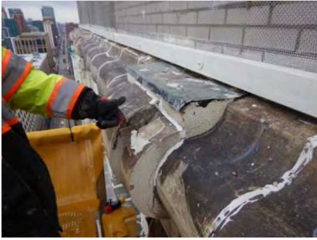
Photo 1: Install tapcons + seal terracotta
