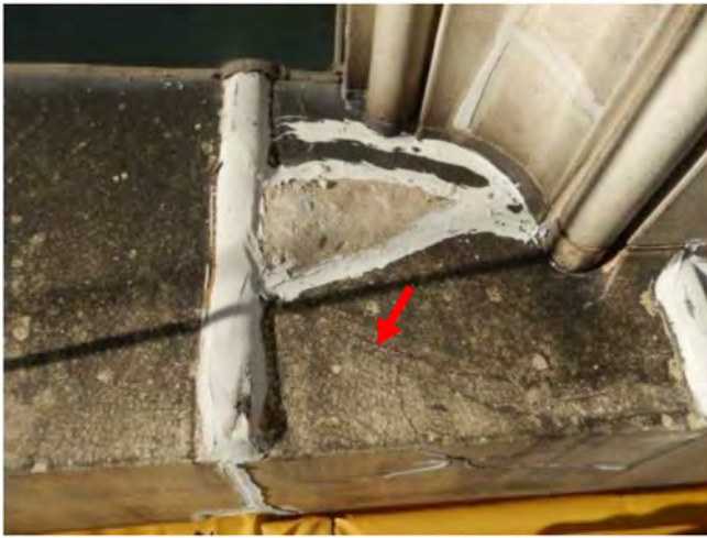
Photo 177: R/S cracks, failed sealant, remove loose + seal
