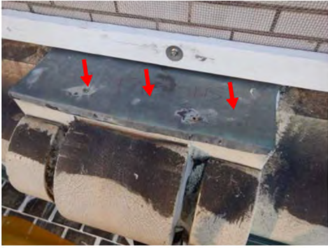
Photo 1: New tapcons to secure aluminum cap
