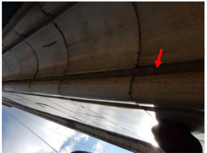
Photo 166: Seal joint
