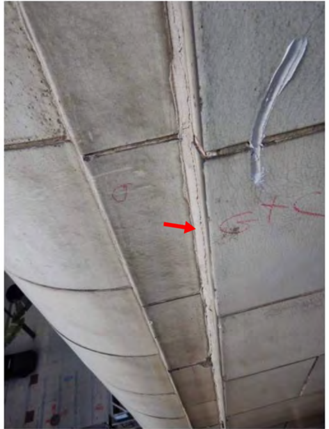
Photo 154: Seal joint
