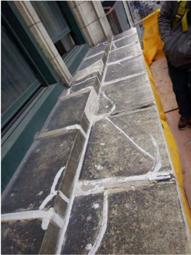
Photo 41: R/S cracks, failed sealant, remove loose material & seal
