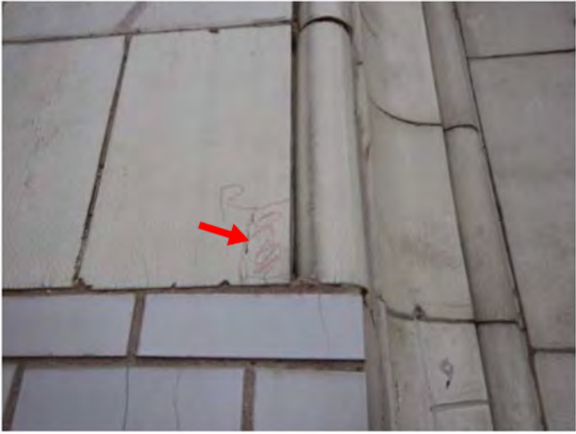
Photo 128: Remove loose + seal
