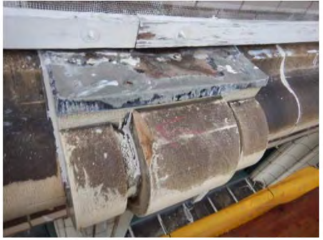
Photo 2: Install tapcons + seal terracotta
