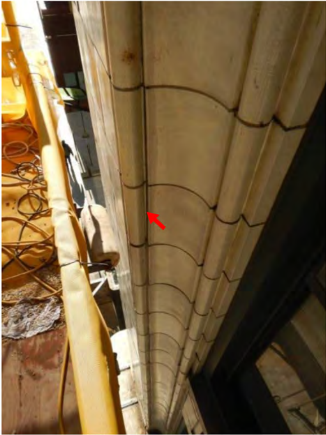
Photo 207: Seal joint
