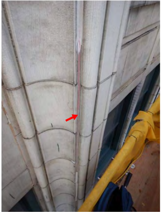
Photo 140: Seal joint
