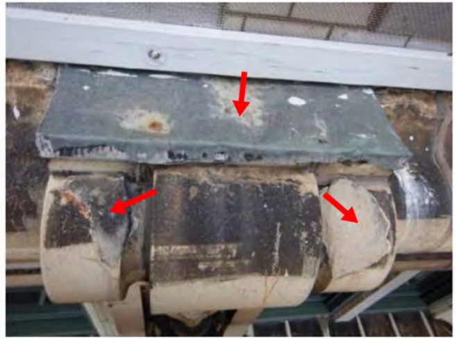
Photo 2: New tapcons to secure cap + seal terracotta
