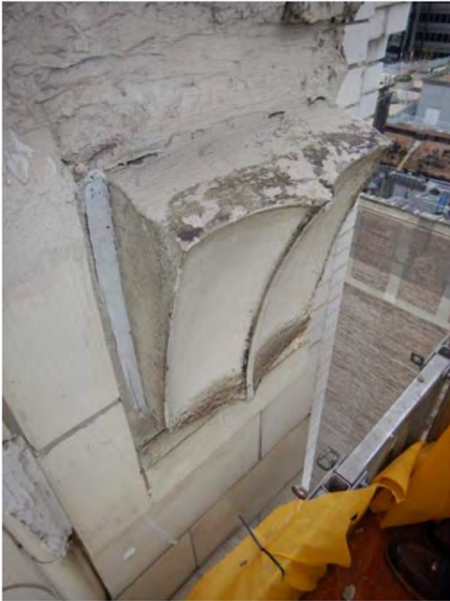
Photo 11: R/S left and top sides of shield
