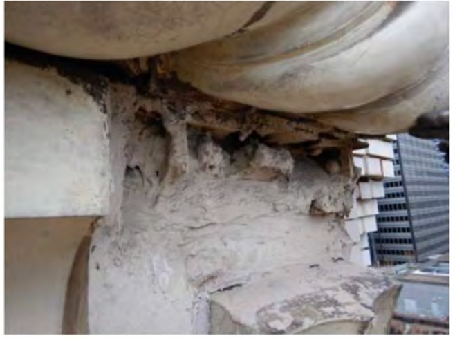
Photo 10: Wire brush + paint exposed steel
