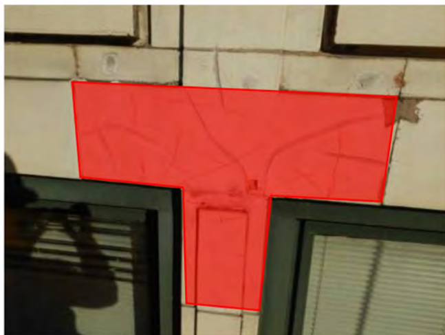
Photo 43: Remove & install plywood
