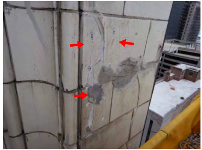
Photo 76: Remove loose + install plywood
