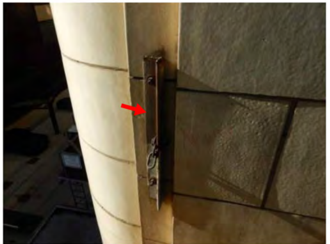
Photo 206: Remove existing angle
