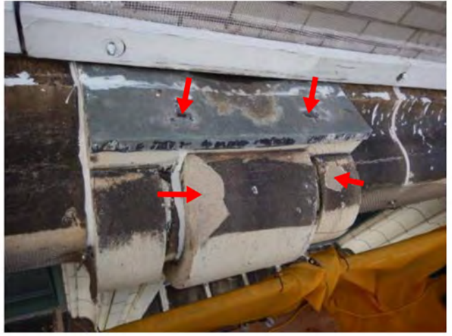
Photo 2: Seal cap anchors + seal terracotta
