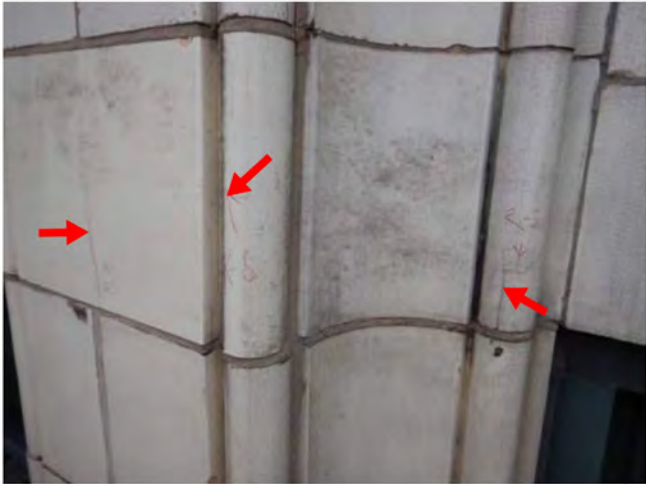
Photo 83: Remove loose + seal
