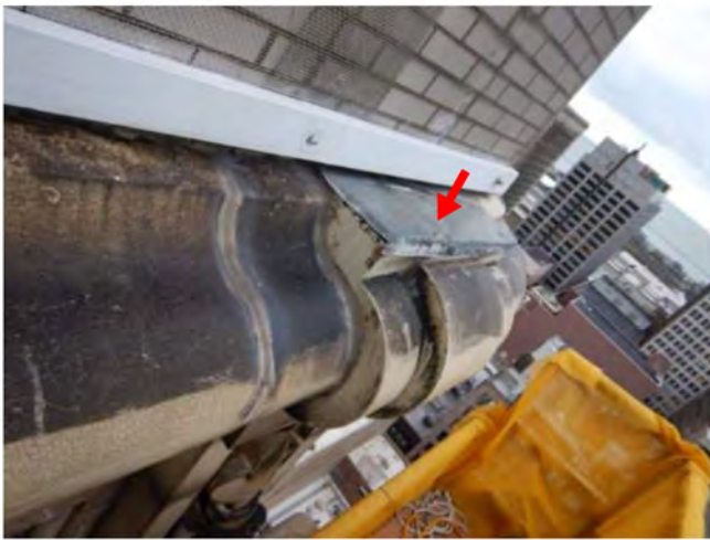
Photo 3: New tapcons to secure cap + seal terracotta
