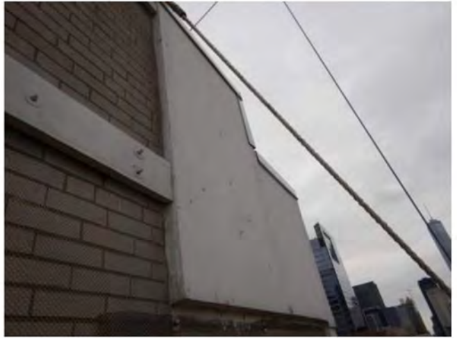
Photo 4: Replace existing wood
