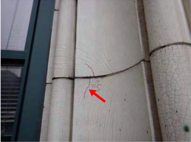
Photo 128: Remove loose + seal
