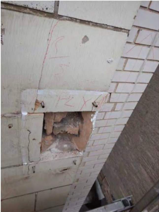
Photo 23: Install plywood & mesh
