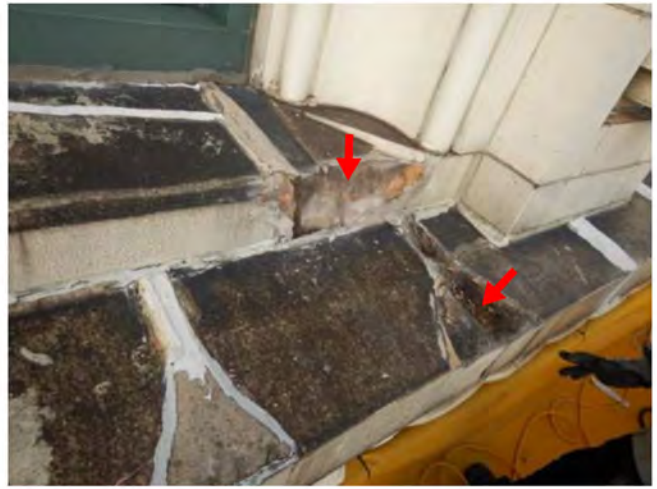
Photo 24: R/S cracks, failed sealant, remove loose + seal
