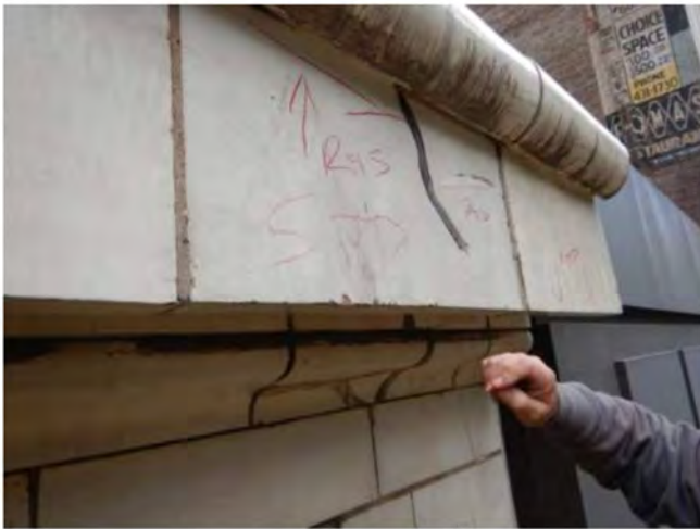
Photo 41: R/S cracks, failed sealant, remove loose material & seal
