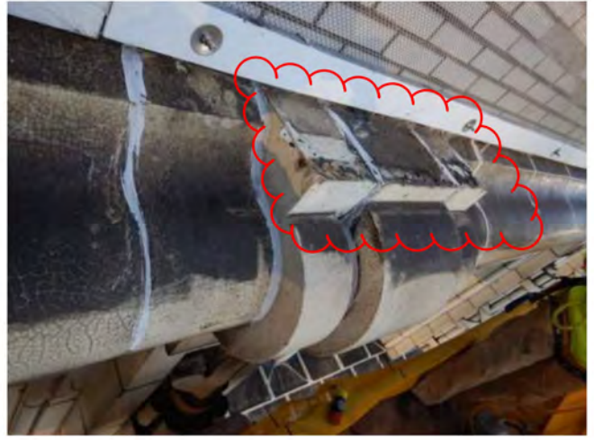
Photo 2: Install new aluminum cap
