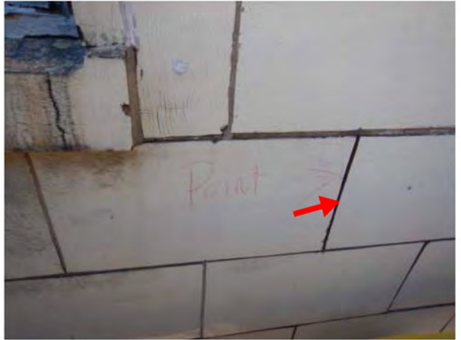
Photo 54: Remove loose + seal
