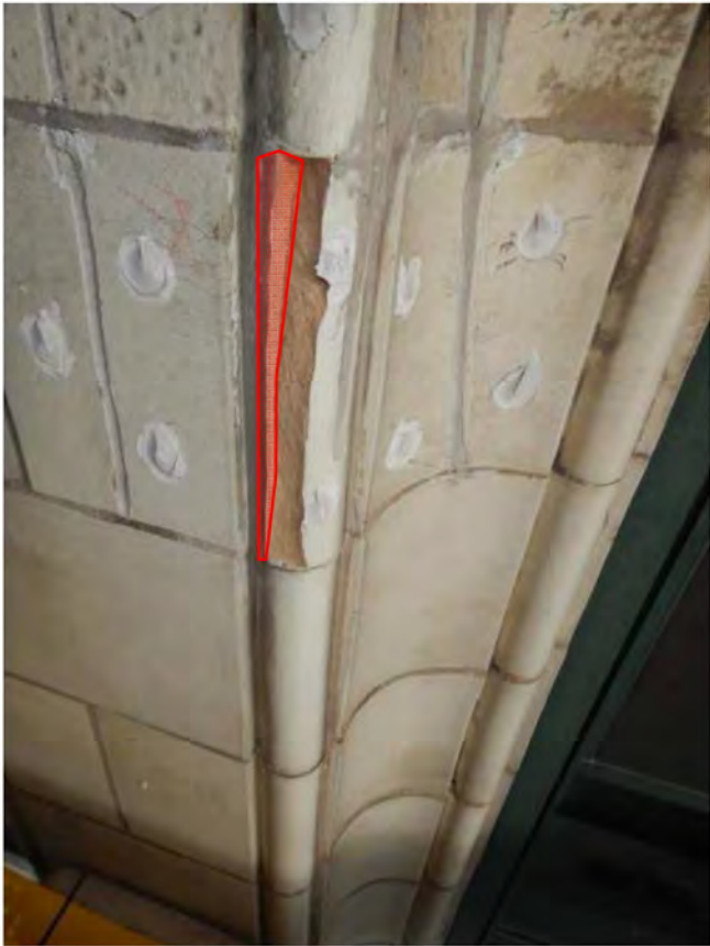
Photo 49: Remove loose
