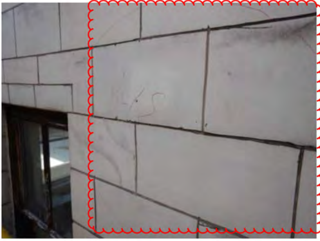
Photo 145: Remove loose + seal or install plywood
