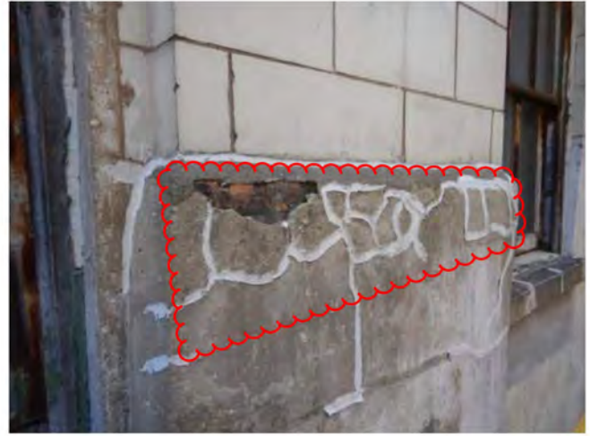
Photo 158: Remove unsound cementitious parge material, prepare substrate, install new coat
