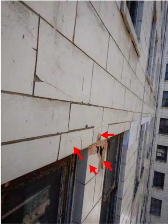
Photo 81: Remove loose + install plywood
