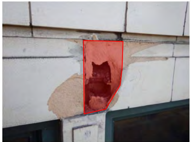
Photo 24: Remove loose & install plywood
