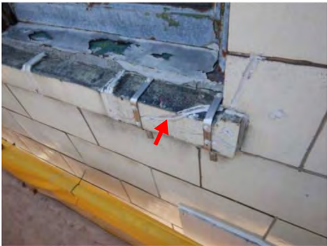
Photo 29: Seal & extend mesh
