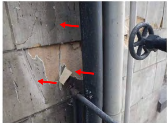
Photo 2: Remove loose + R/S cracks + install wood
