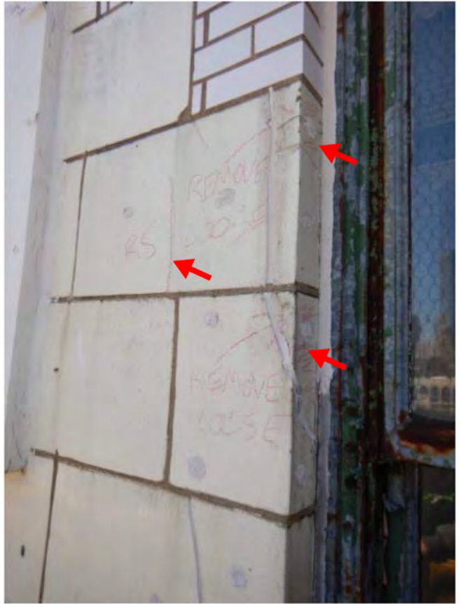
Photo 6: Remove loose + install plywood
