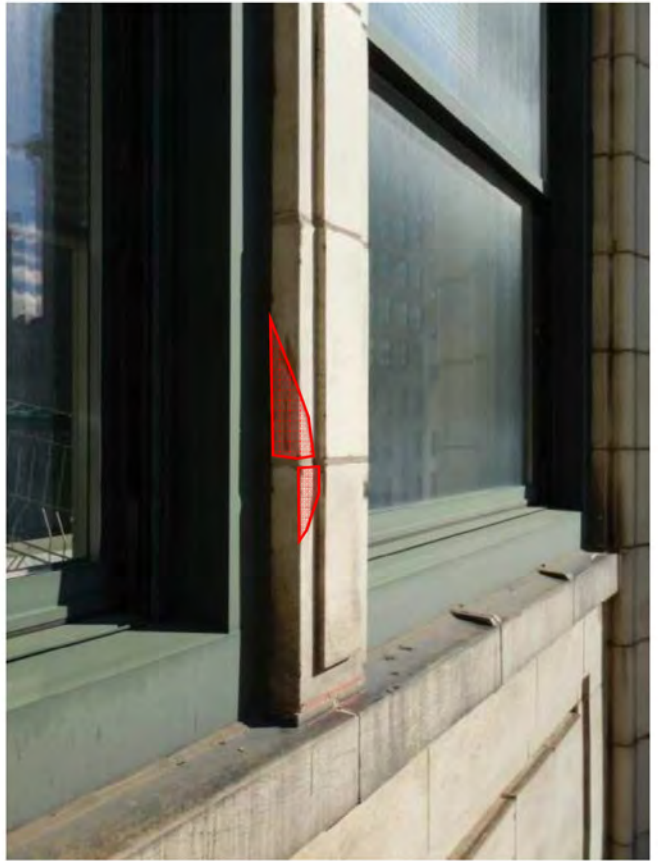
Photo 94: Remove loose
