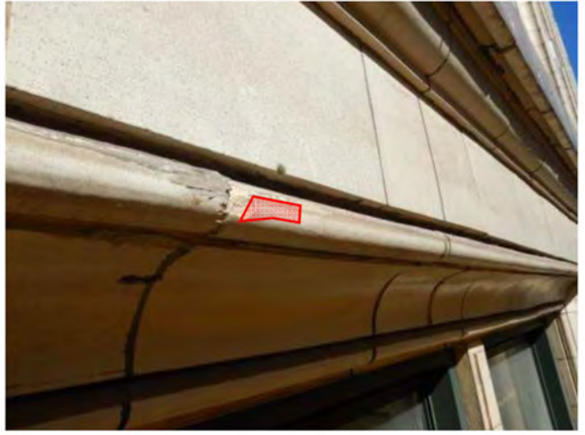
Photo 186: Remove loose
