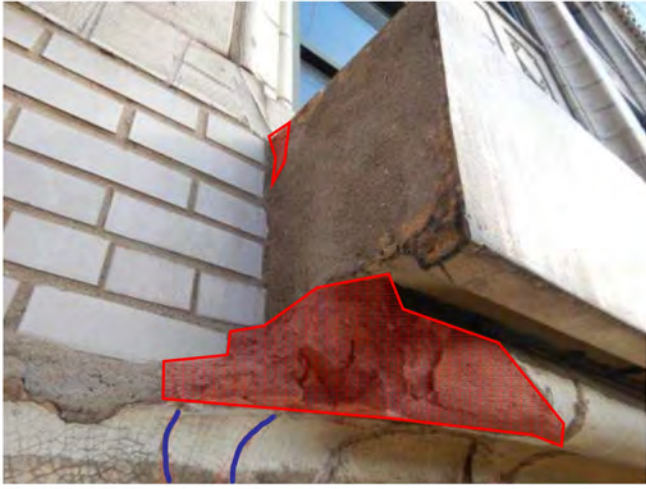
Photo 47: Remove loose, clean & seal
