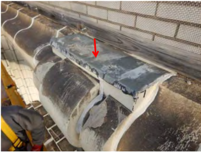
Photo 1: New tapcons to secure aluminum cap
