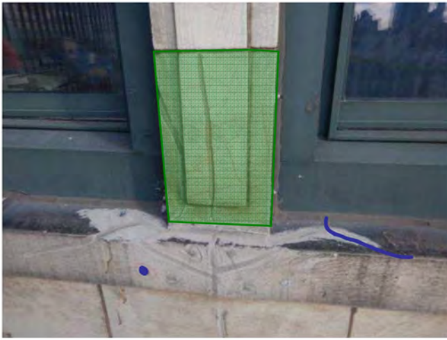
Photo 51: Remove loose, install plywood & R/S
