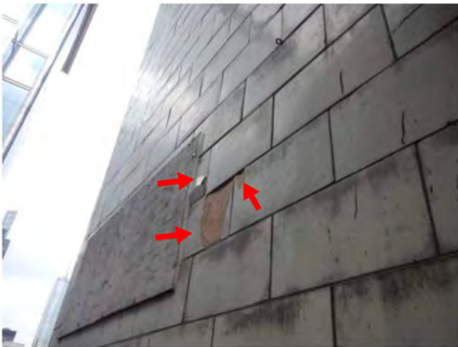
Photo 43: Remove loose + R/S cracks + install wood
