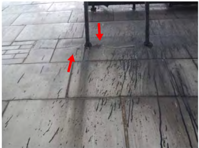
Photo 18: Remove loose + R/S cracks + install wood
