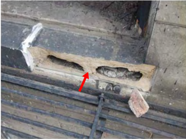
Photo 7: Remove loose + R/S cracks + install wood
