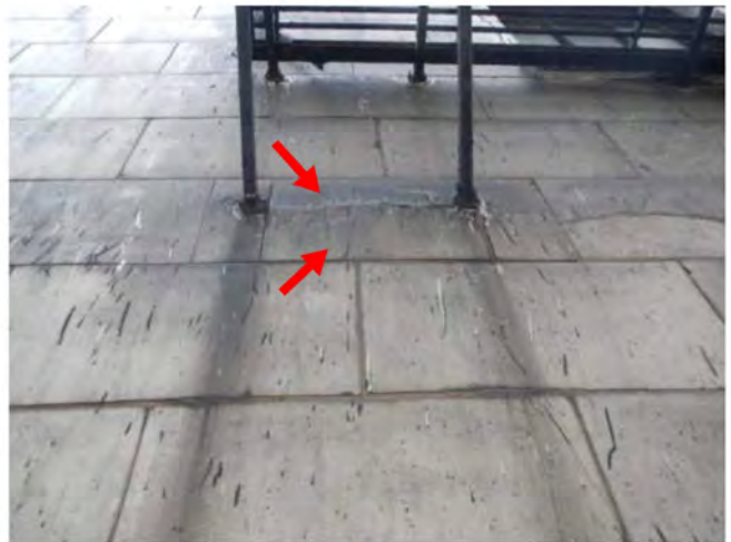
Photo 10: Remove loose + R/S cracks + install wood
