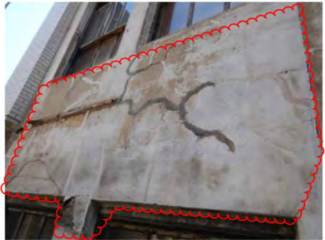
Photo 160: Remove unsound parge, prepare substrate, install new coat
