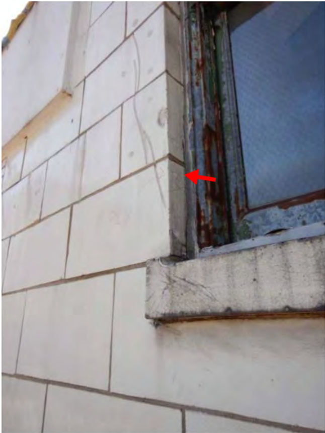
Photo 7: Remove loose + install plywood
