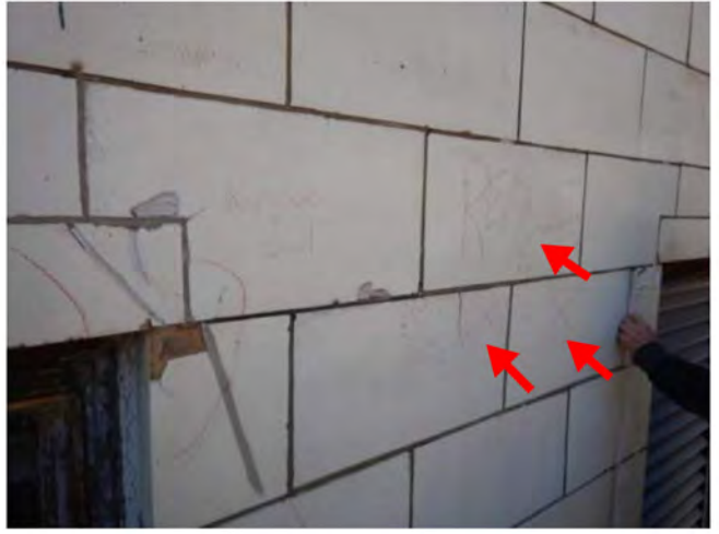
Photo 50: Remove loose + install plywood
