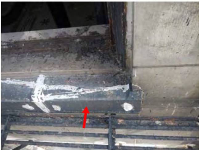
Photo 9: Remove loose + R/S cracks + install wood
