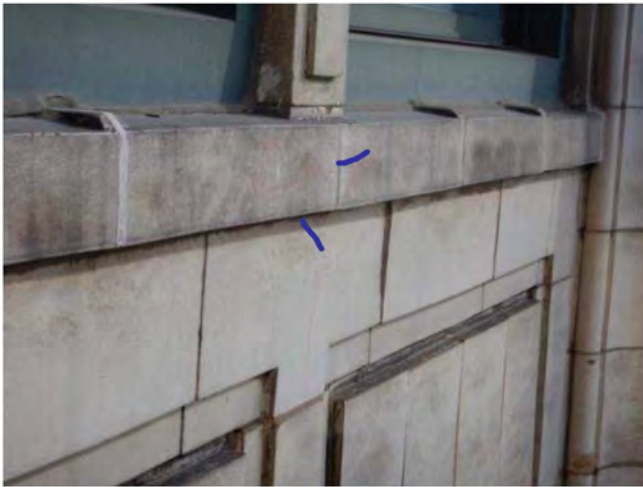
Photo 51: Remove loose, install plywood & R/S
