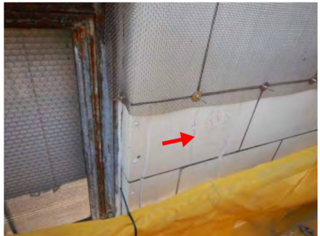
Photo 26: Remove loose + install plywood
