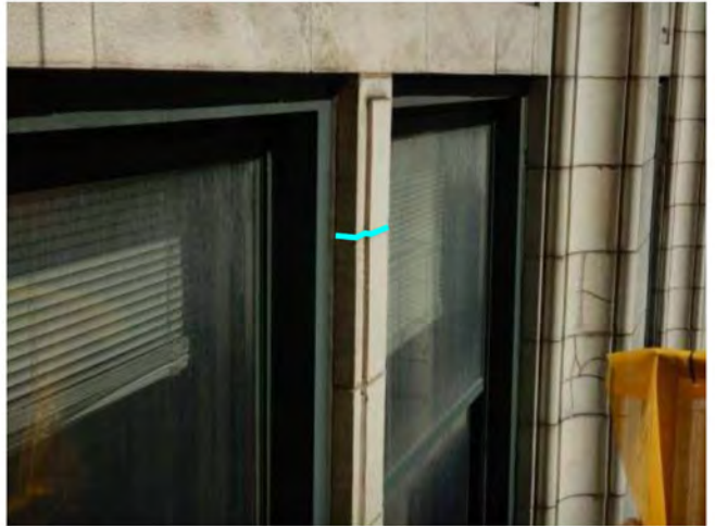
Photo 154: Remove loose + TP
