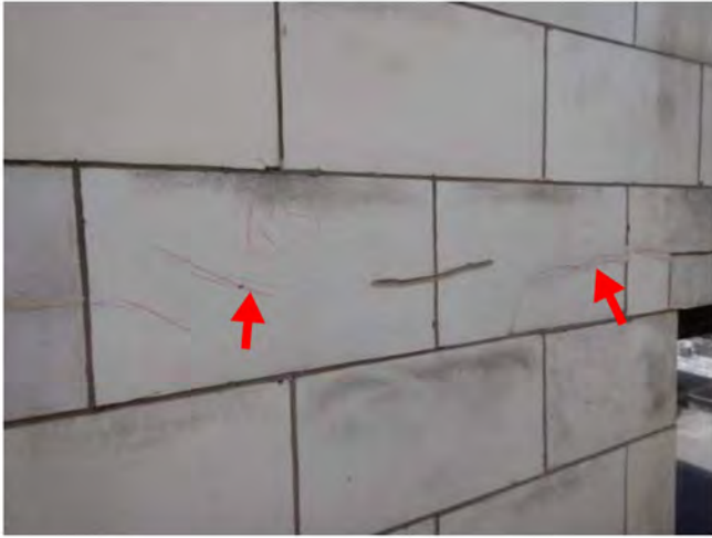
Photo 145: Remove loose + seal or install plywood
