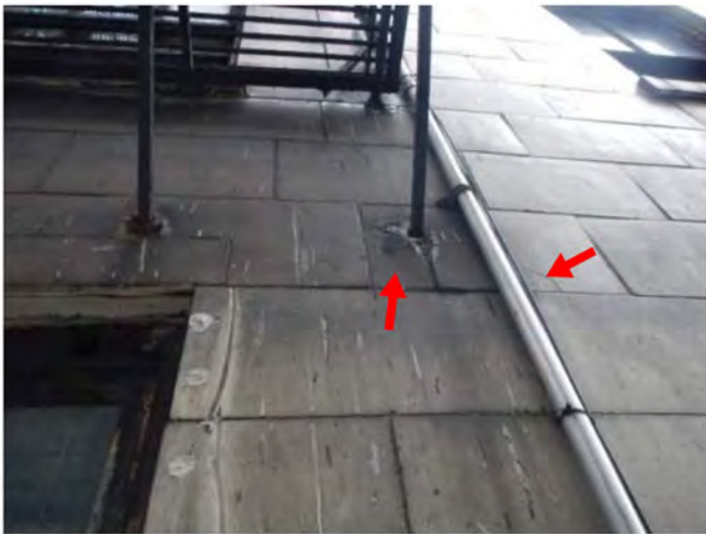
Photo 21: Remove loose + R/S cracks + install wood
