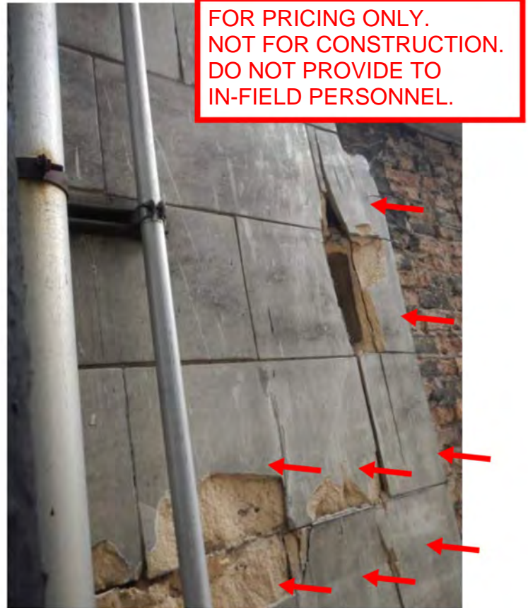
Photo 2: Remove loose + R/S cracks + install wood
