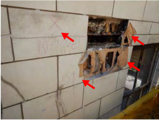
Photo 103: Remove loose + install plywood
