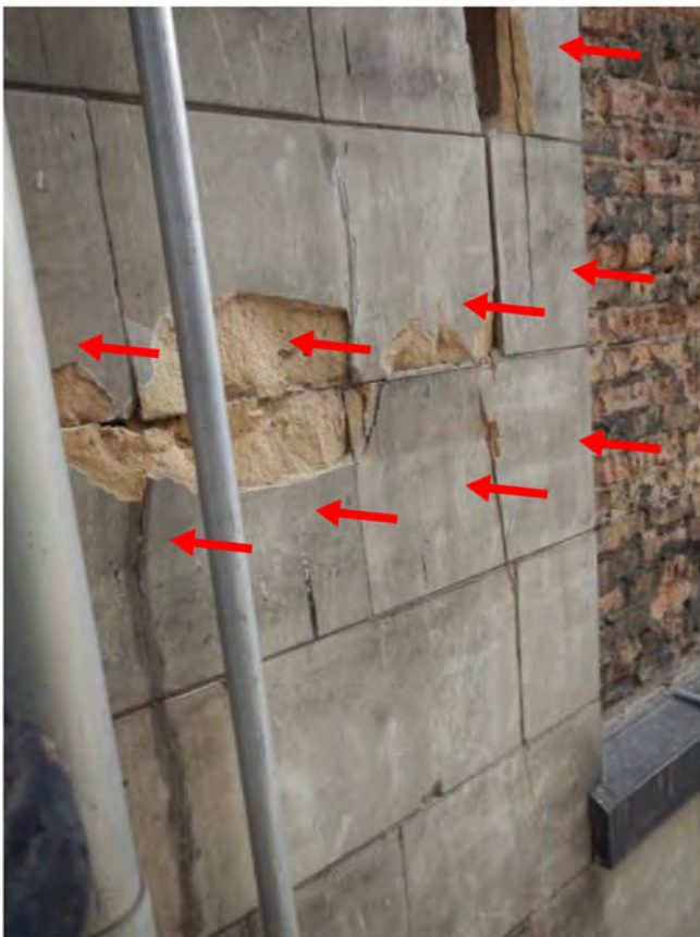
Photo 3: Remove loose + R/S cracks + install wood
