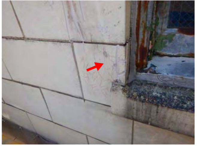
Photo 54: Remove loose + seal
