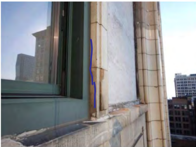
Photo 53: R/S or remove if material is loose
