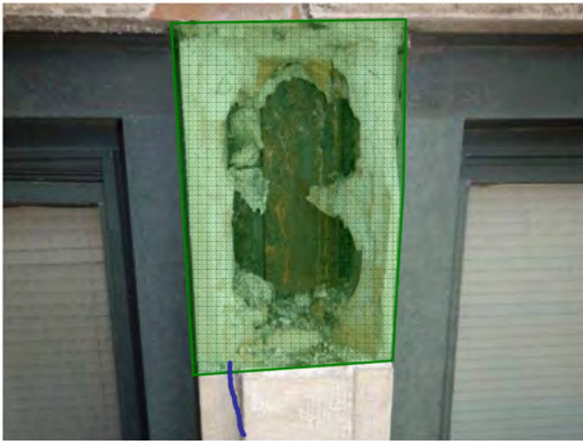
Photo 43: Remove loose, install plywood & R/S
