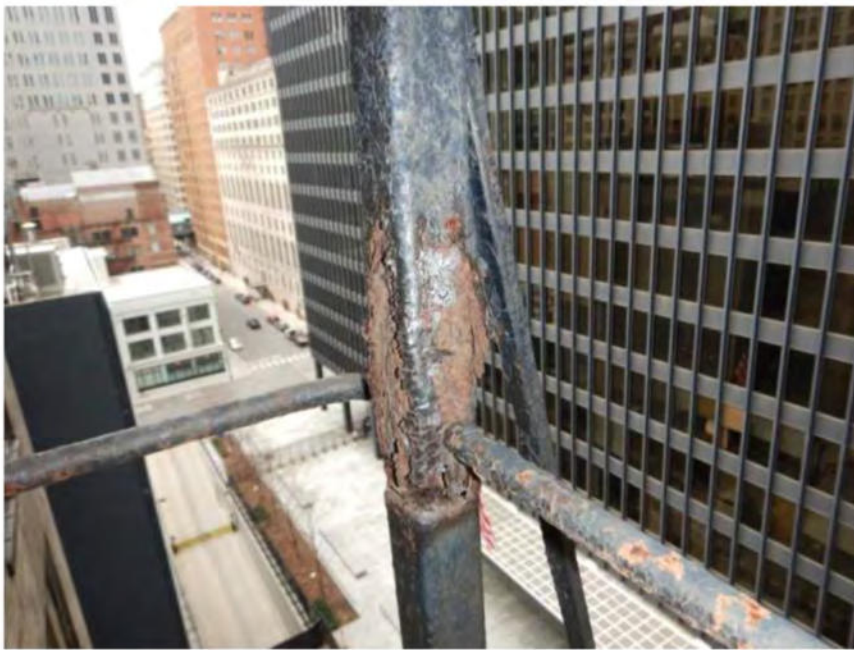
Photo 2: Item #2: Full replacement of handrail post
