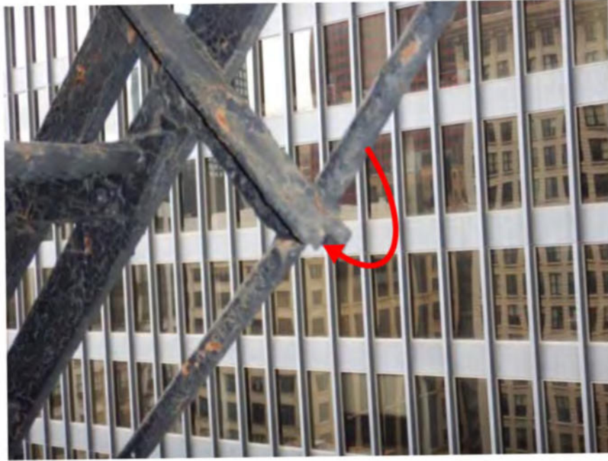
Photo 9: Item #9: Replacement of stringer bottom chord brace (angle) at Level 14
