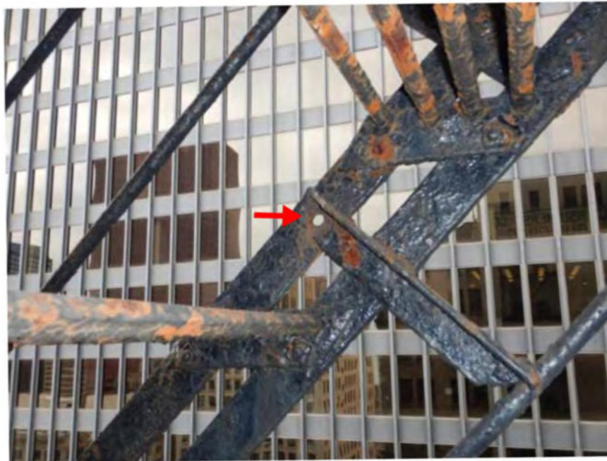
Photo 10: Item #9: Replacement of stringer bottom chord brace (angle) at Level 20
