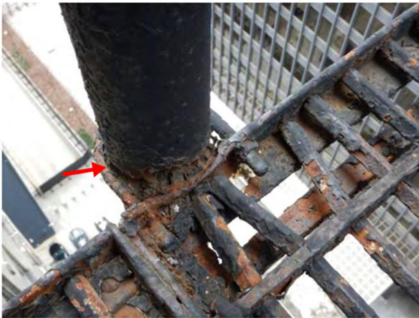
Photo 13: Item #12: Removal of existing stand pipe
