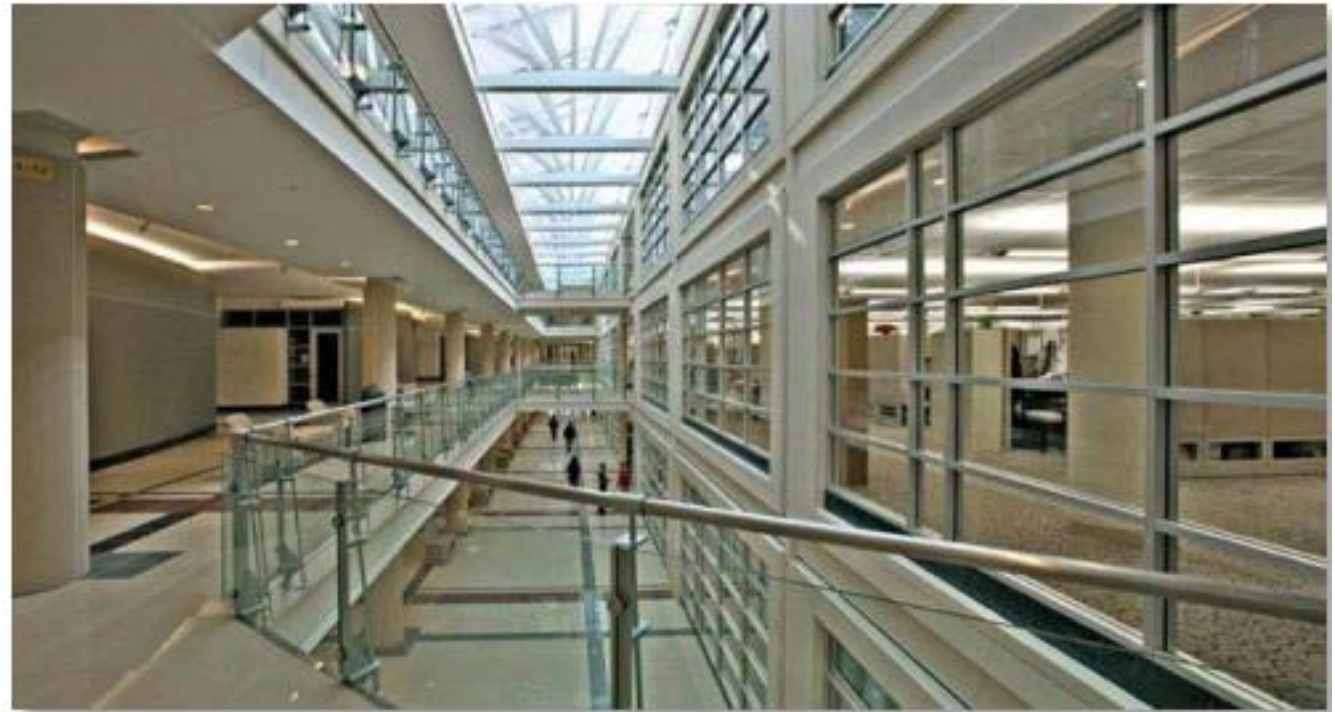
SSA Offices now Credit: Hensel Phelps
