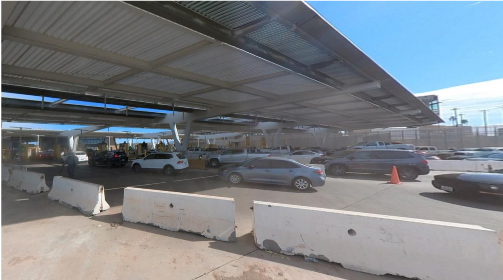
New Pre-Primary Canopy – View Looking towards East
