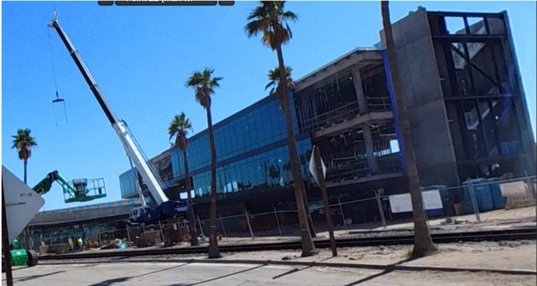
New Administration Building – Looking South towards Mexico
