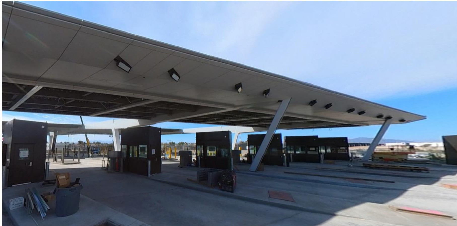
Primary Canopy Expansion – View looking towards West
