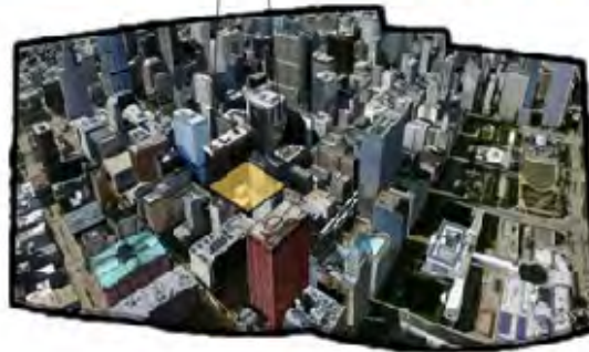
Site Aerial View
