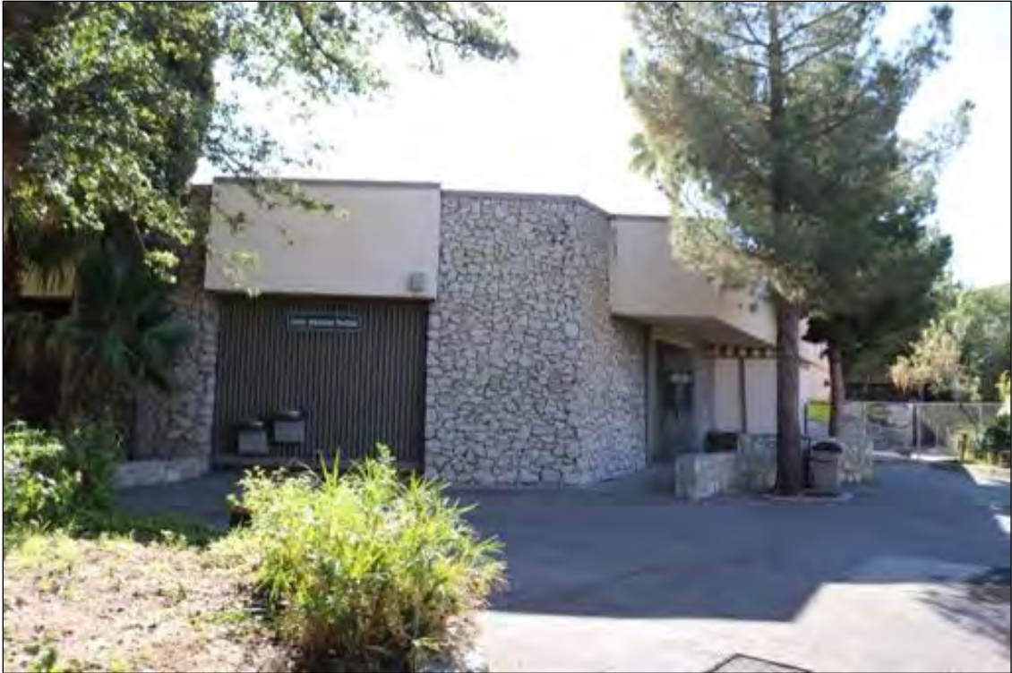
Figure 236. South American Pavilion, looking southeast.
