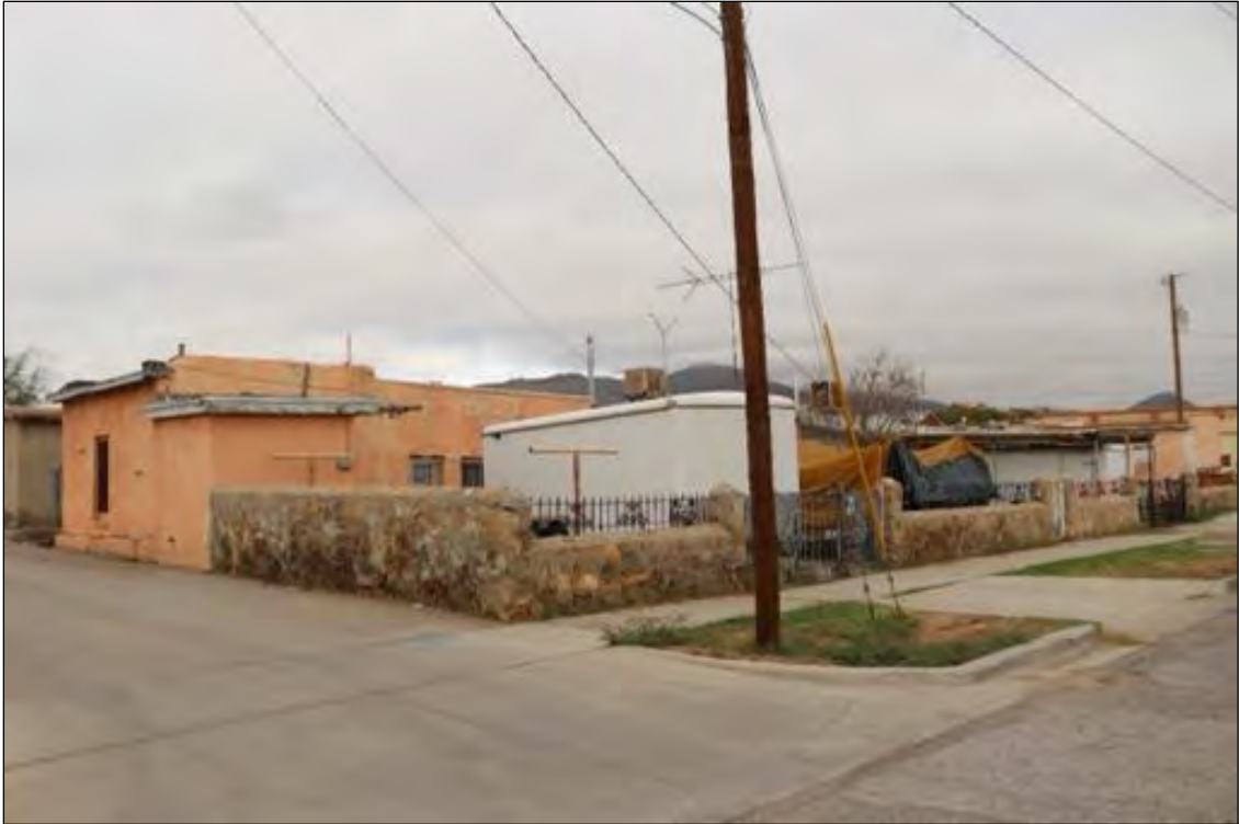
Figure 183. 3726 E San Antonio Avenue (Residence), looking northwest.
