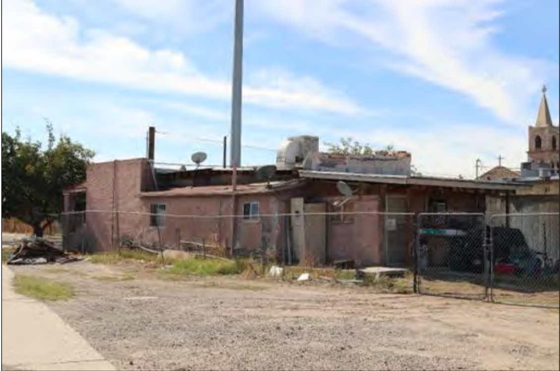
Figure 167. 3821 Findley Avenue (Residence) rear, looking southwest.
