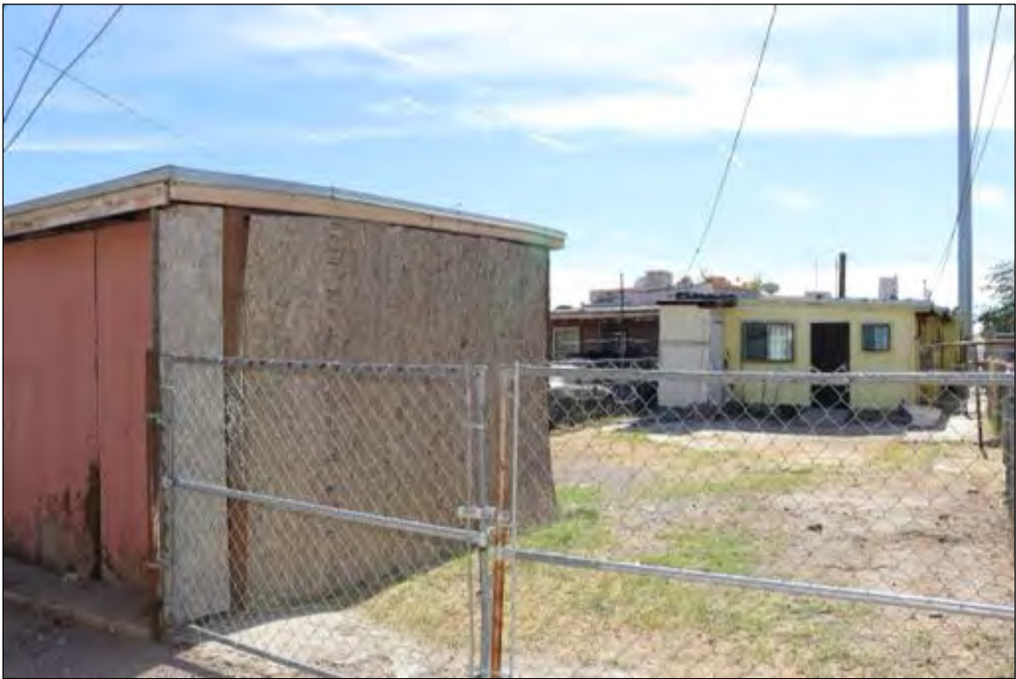
Figure 165. 3819 Findley Avenue (Residence) rear, looking southeast.
