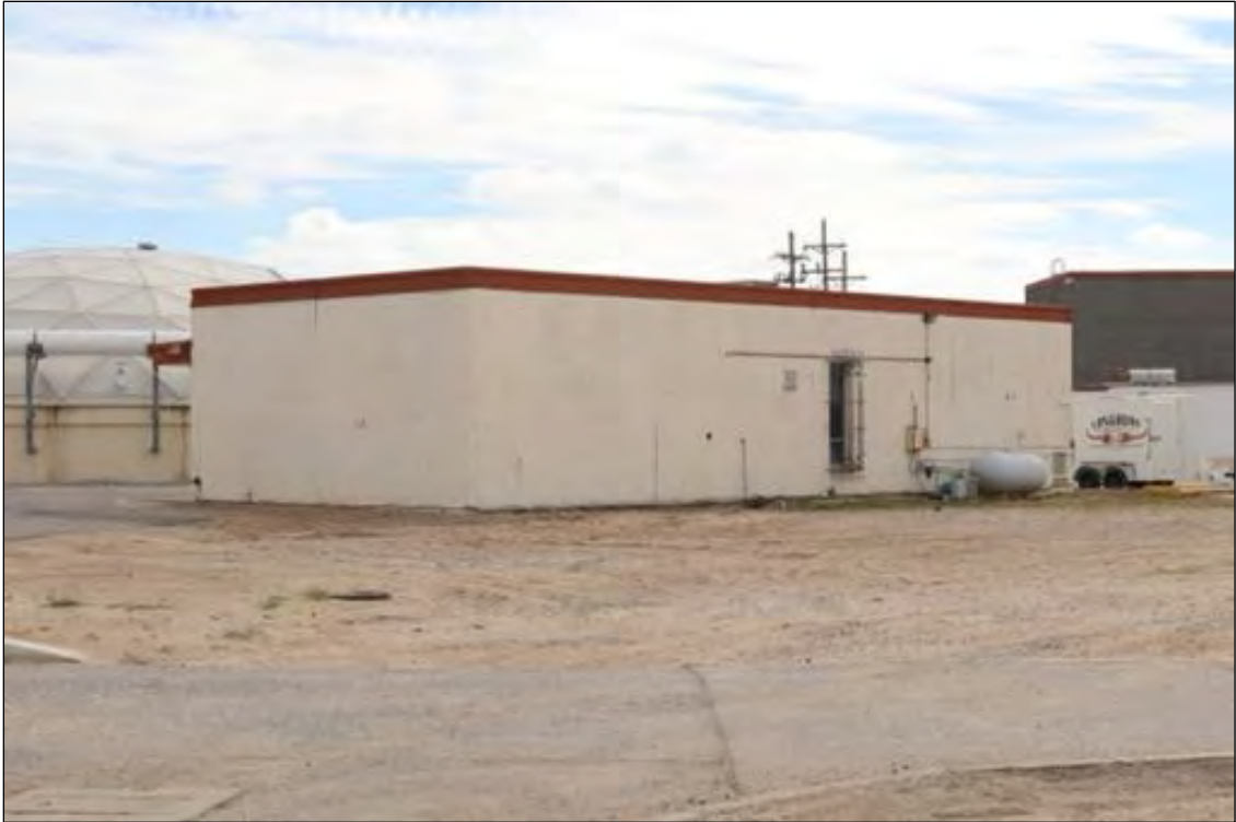
Figure 256. Building, looking southwest.
