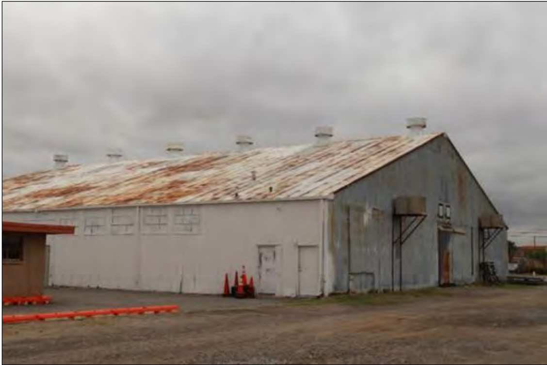
Figure 226. Holding Area Shelter, western wing, looking southeast.
