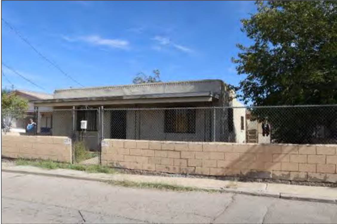
Figure 86. 204 Hardesty Place (Residence), looking northeast.
