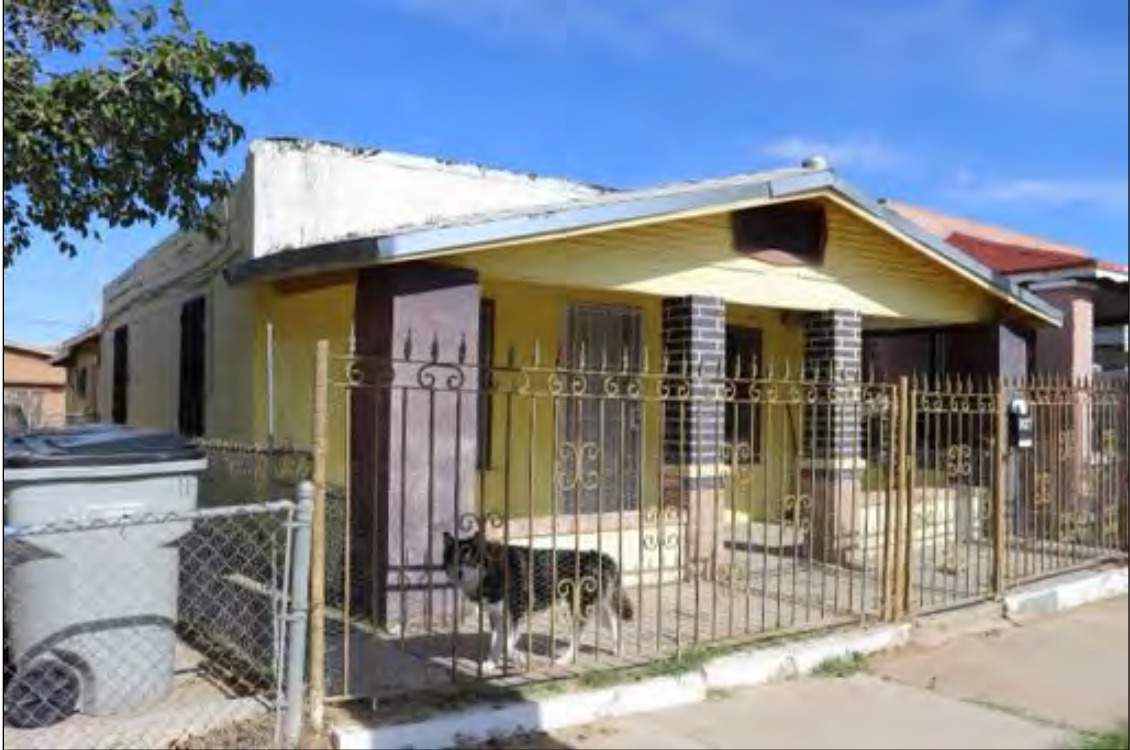
Figure 164. 3819 Findley Avenue (Residence), looking northeast.
