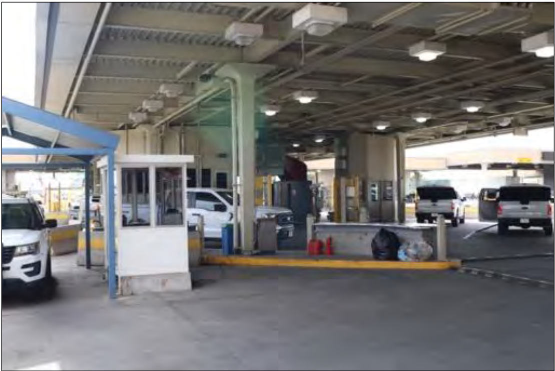
Figure 70. 3600 E Paisano Drive (Building K Primary/Secondary Inspection Canopy), Secondary Inspection Canopy.
