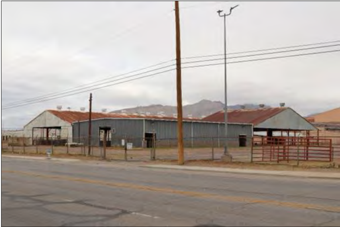
Figure 229. Holding Area Storage Building (right) and Holding Area Shelter (left and background), looking northwest.
