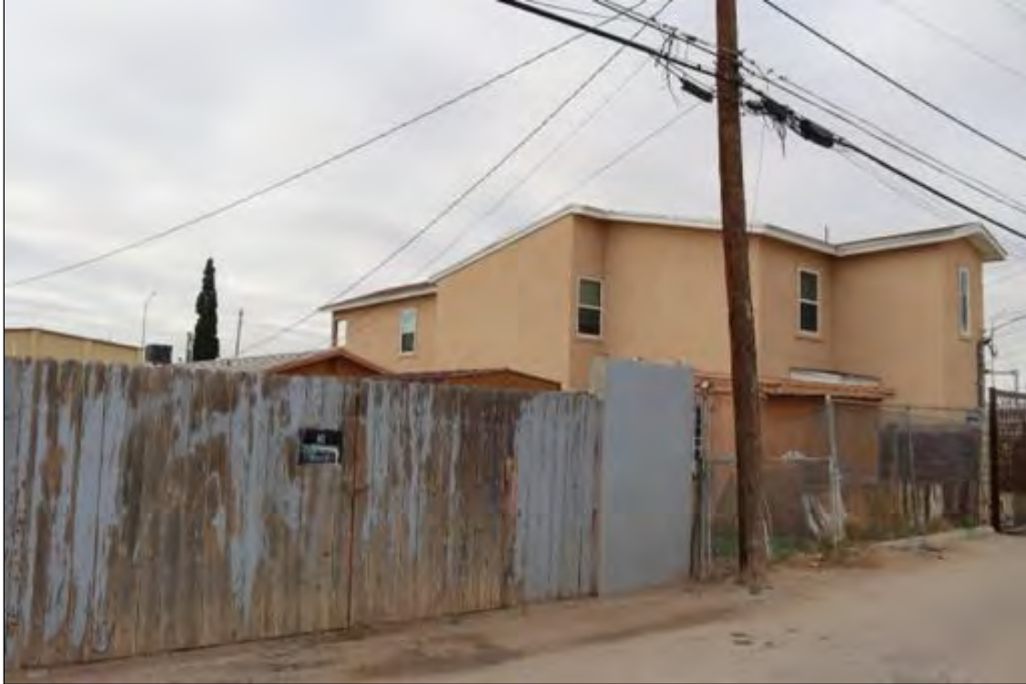
Figure 140. 3717 Findley Avenue (Residence) rear, looking southwest.
