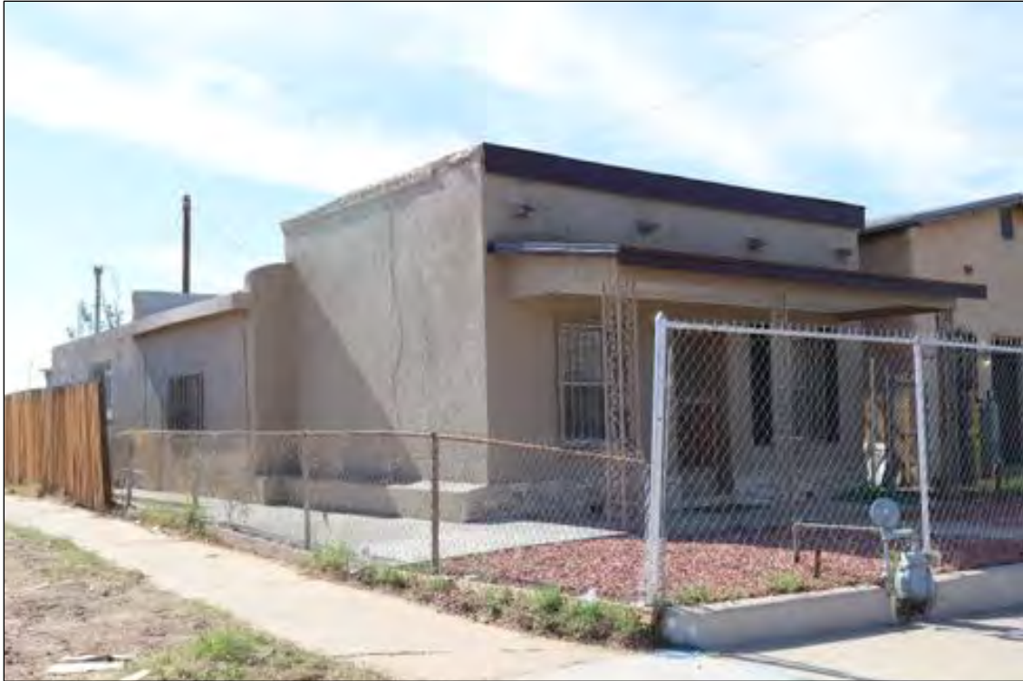
Figure 160. 3816 Findley Avenue (Residence), looking southwest.
