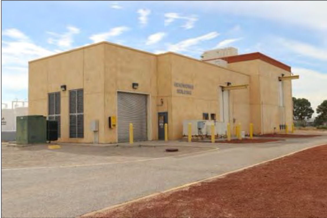
Figure 254. Headworks Building, looking southwest.
