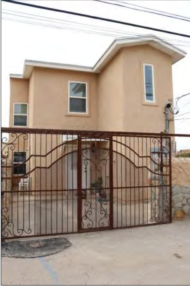
Figure 136. 3711 Findley Avenue (Residence) rear, looking south.
