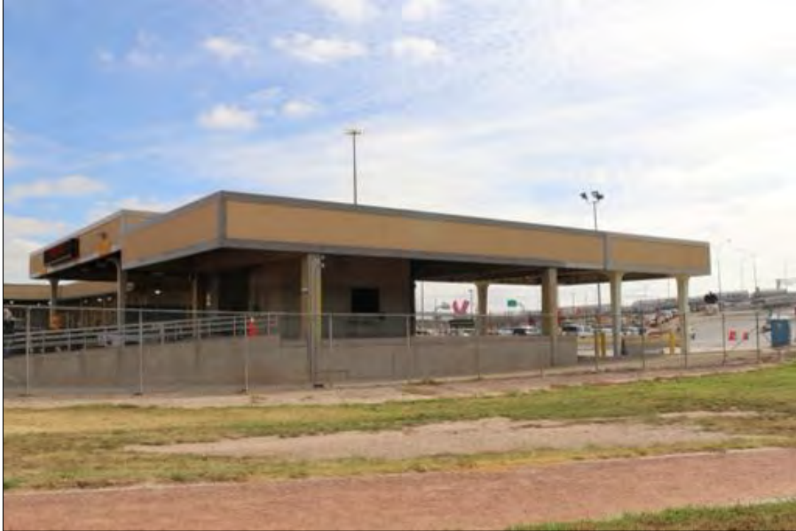
Figure 84. 3600 E Paisano Drive (Southbound Inspection Canopy), looking southeast.
