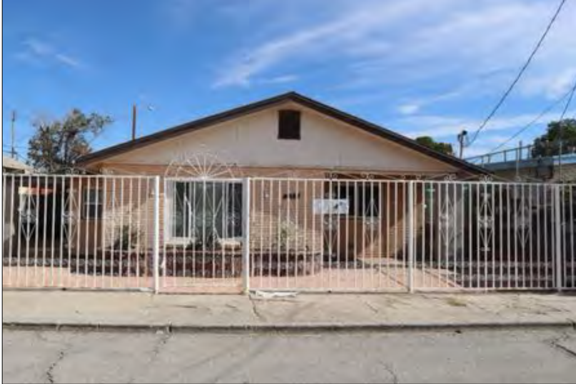
Figure 104. 220 Hardesty Place (Residence), looking east.
