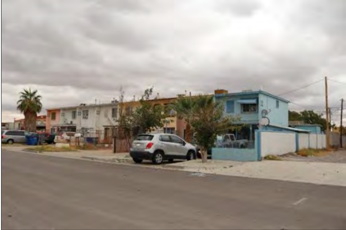
Figure 48. 700–714 S Martinez Street (Apartment Complex), looking northeast.
