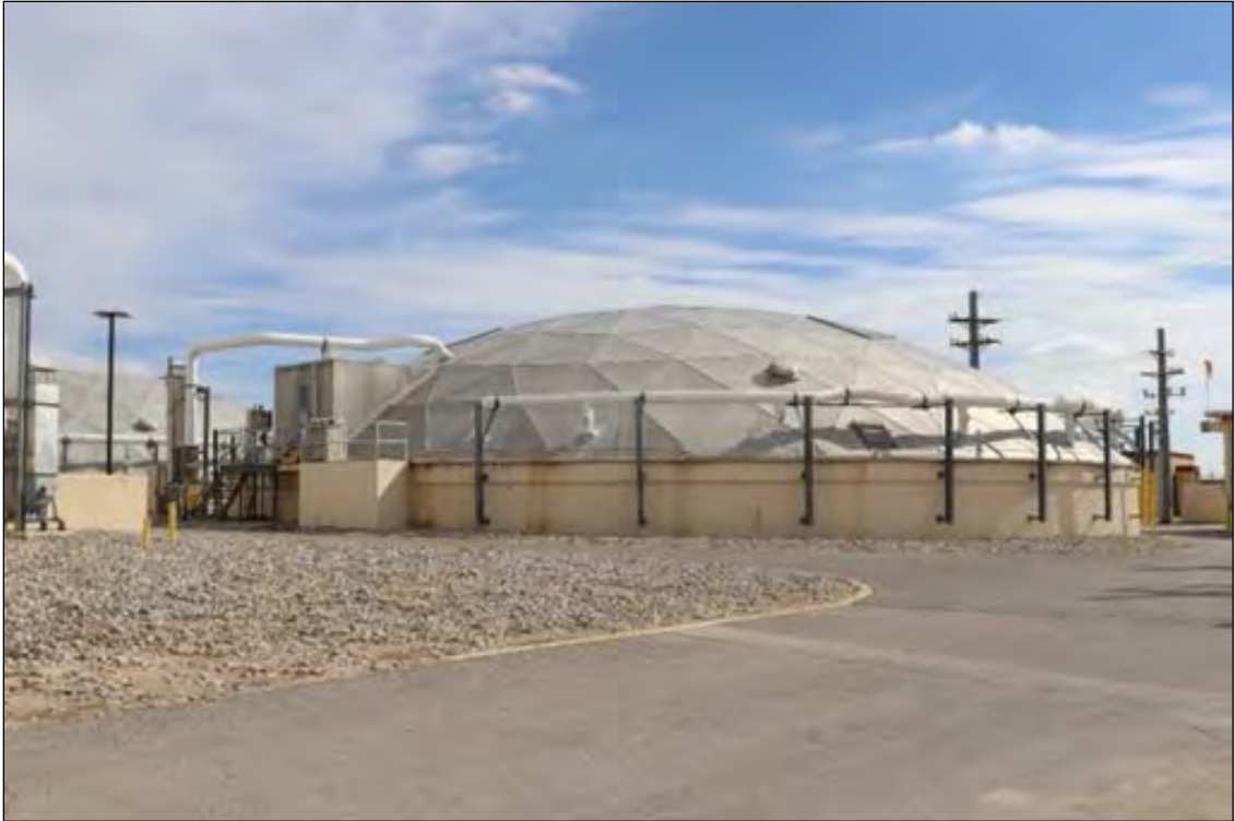
Figure 260. Digestion Tank, looking southeast.
