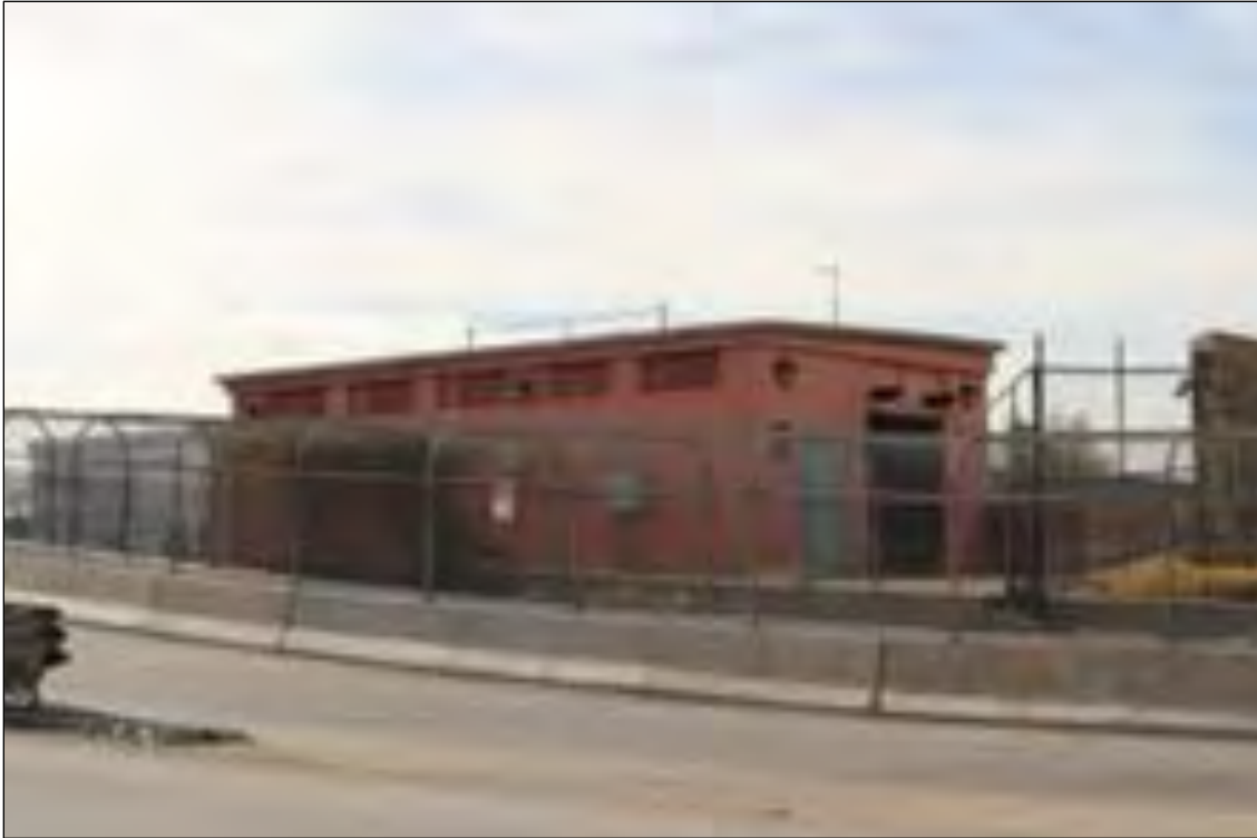
Figure 24. El Paso Water Support Building, looking southwest.
