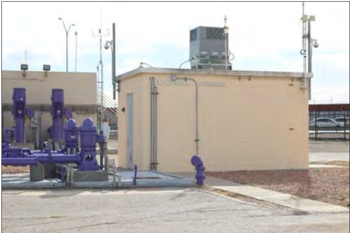
Figure 265. Electrical Building, looking south.
