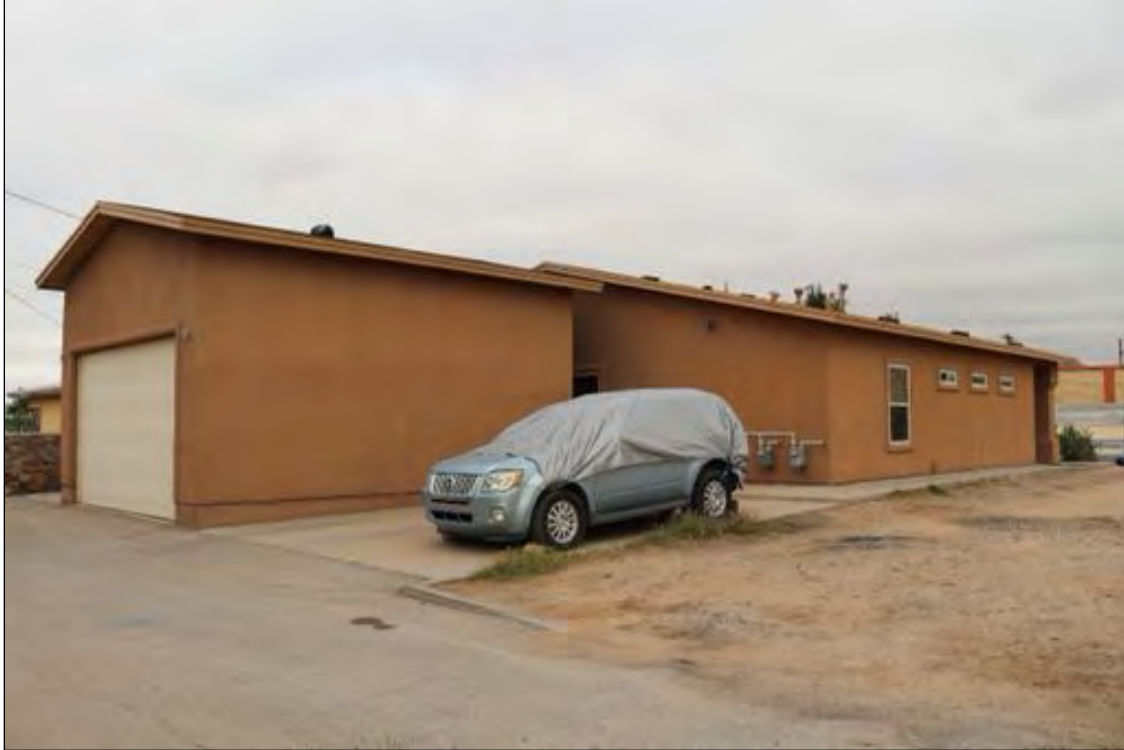
Figure 174. 3710 E San Antonio Avenue (Duplex) rear, looking northwest.
