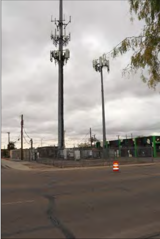
Figure 28. 3930 Delta Drive (Substation), looking southwest.
