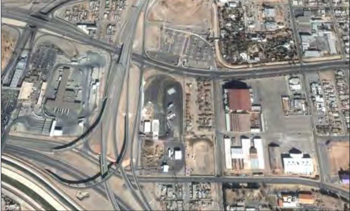
Figure 203. Aerial showing the location of the TxDOT Facility in December 2005 (courtesy of Google Earth).
