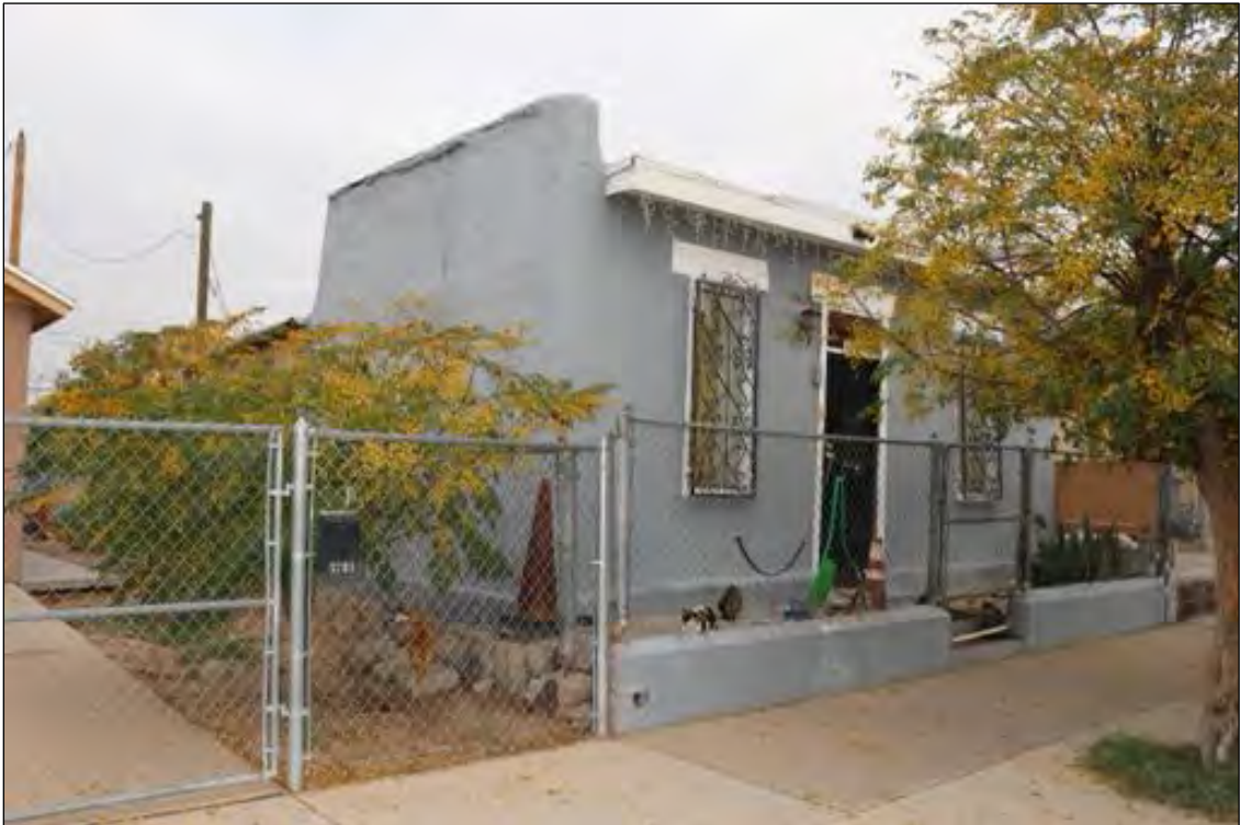
Figure 131. 3705 Findley Avenue (Residence), looking northeast.
