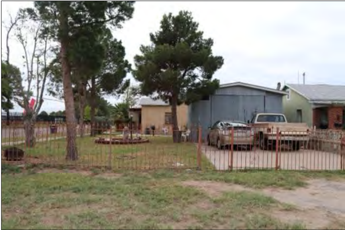
Figure 46. 4030 Laredo Avenue (Residence) rear, looking south.
