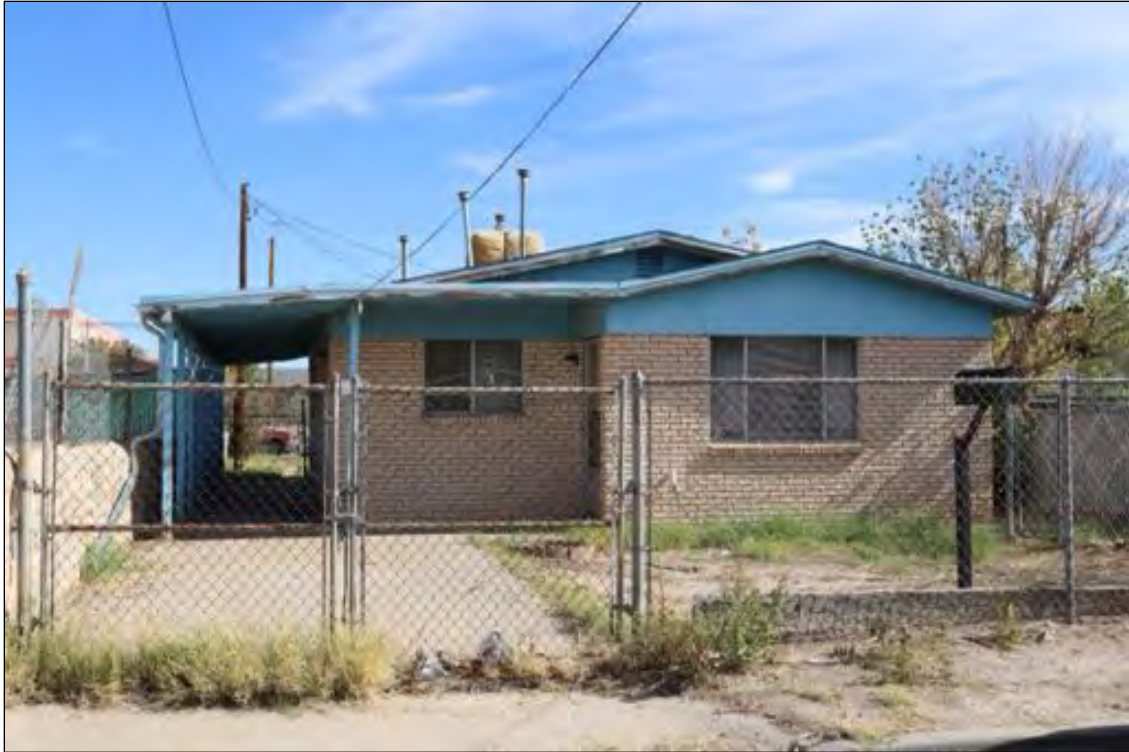
Figure 97. 214 Hardesty Place (Residence), looking east.
