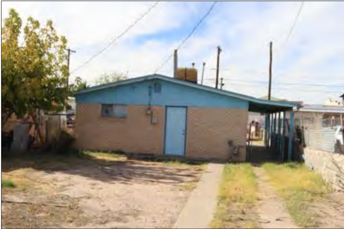
Figure 98. 214 Hardesty Place (Residence) rear, looking west.
