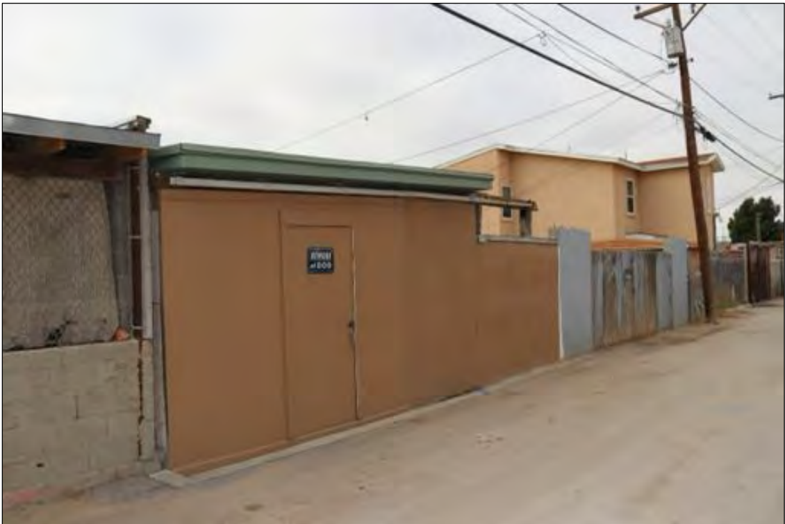
Figure 142. 3719 Findley Avenue (Residence) rear, looking southwest.
