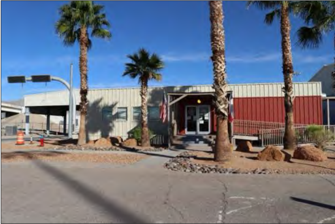
Figure 205. 4000 E Paisano Drive (Office), looking north.
