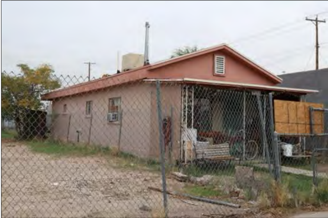
Figure 145. 3733 Findley Avenue (Residence), looking northeast.
