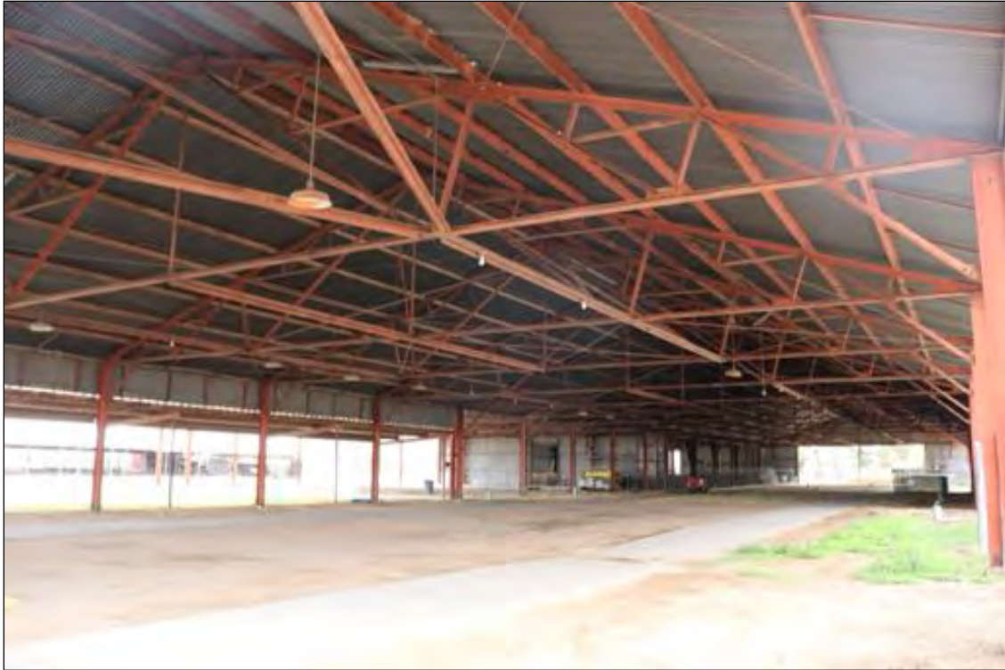
Figure 225. Holding Area Shelter metal frame, looking south.
