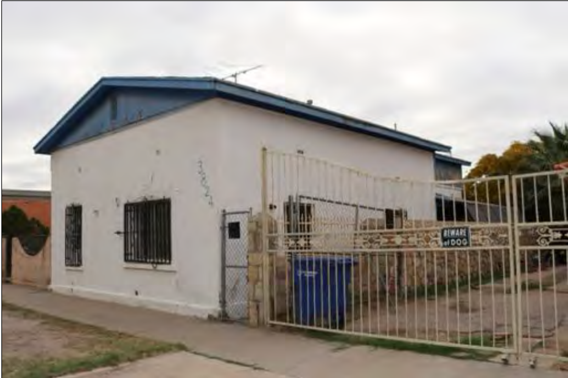
Figure 195. 3824 E San Antonio Avenue (Residence), looking southeast.
