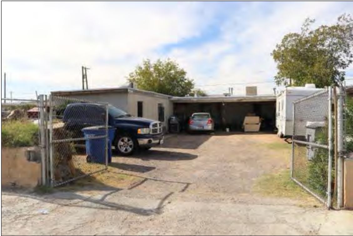
Figure 87. 204 Hardesty Place (Residence) rear, looking southwest.
