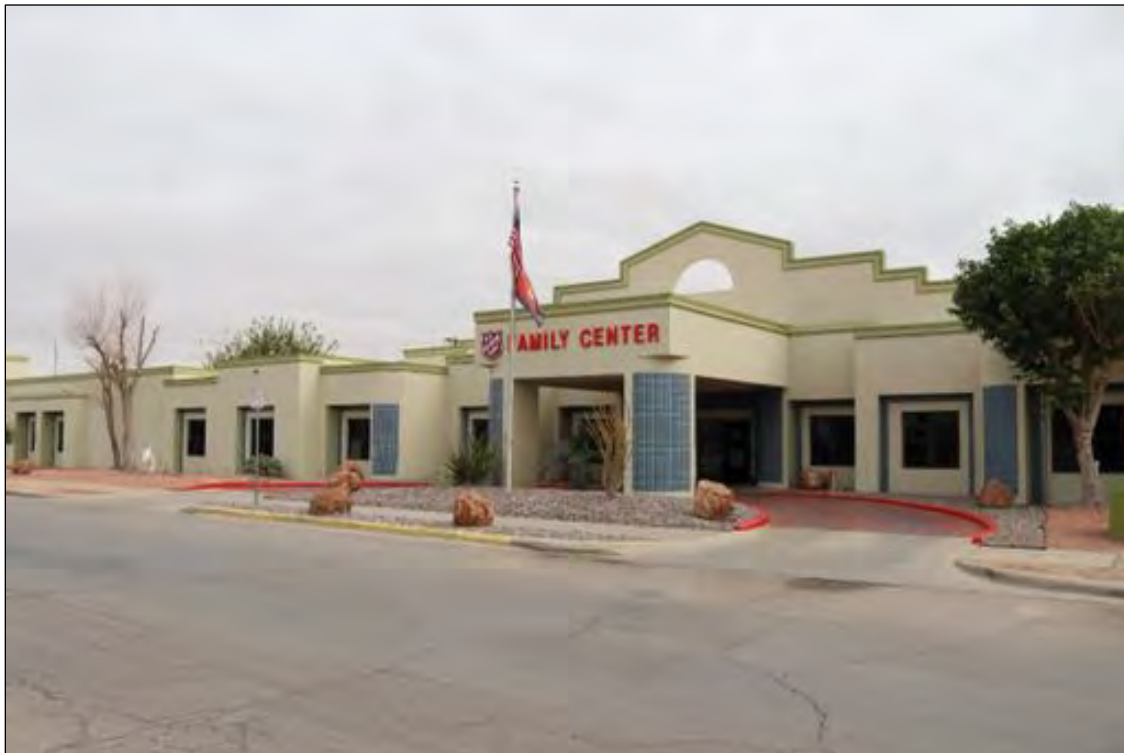
Figure 1115. 4300 E Paisano Drive (Salvation Army Family Center), looking west.
