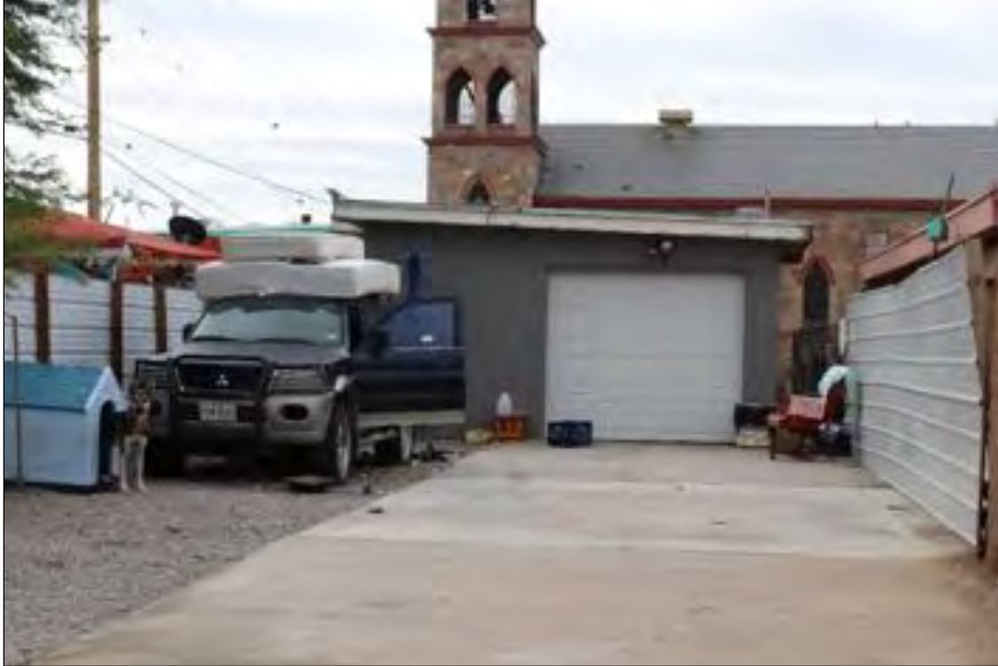
Figure 148. 3735 Findley Avenue (Residence) rear, looking south.
