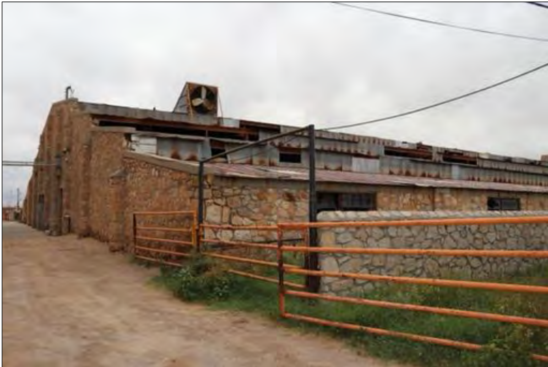
Figure 217. Coliseum Livestock barns, looking east.
