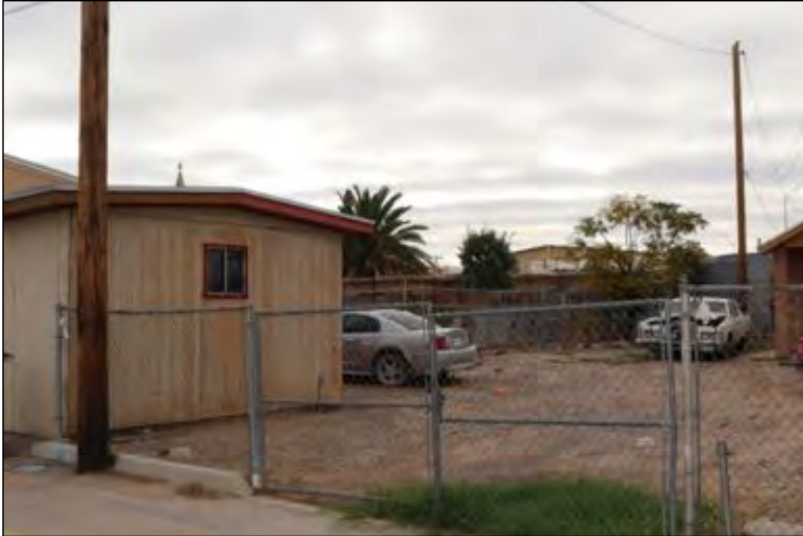
Figure 132. 3705 Findley Avenue (Residence) rear, looking southwest.
