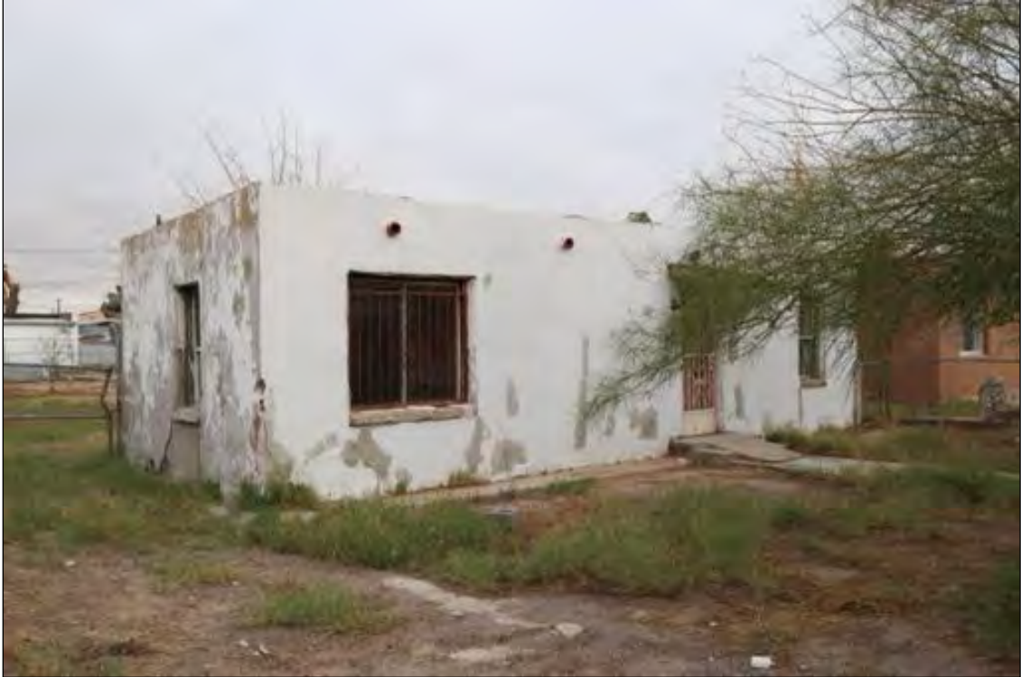
Figure 57. 4007 Oak Court (Residence), looking northeast.
