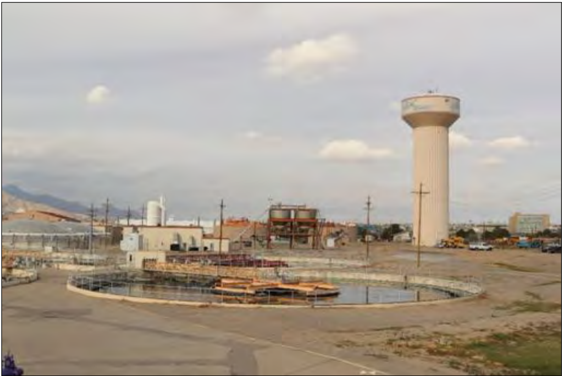
Figure 269. Basins and water tower, looking north.
