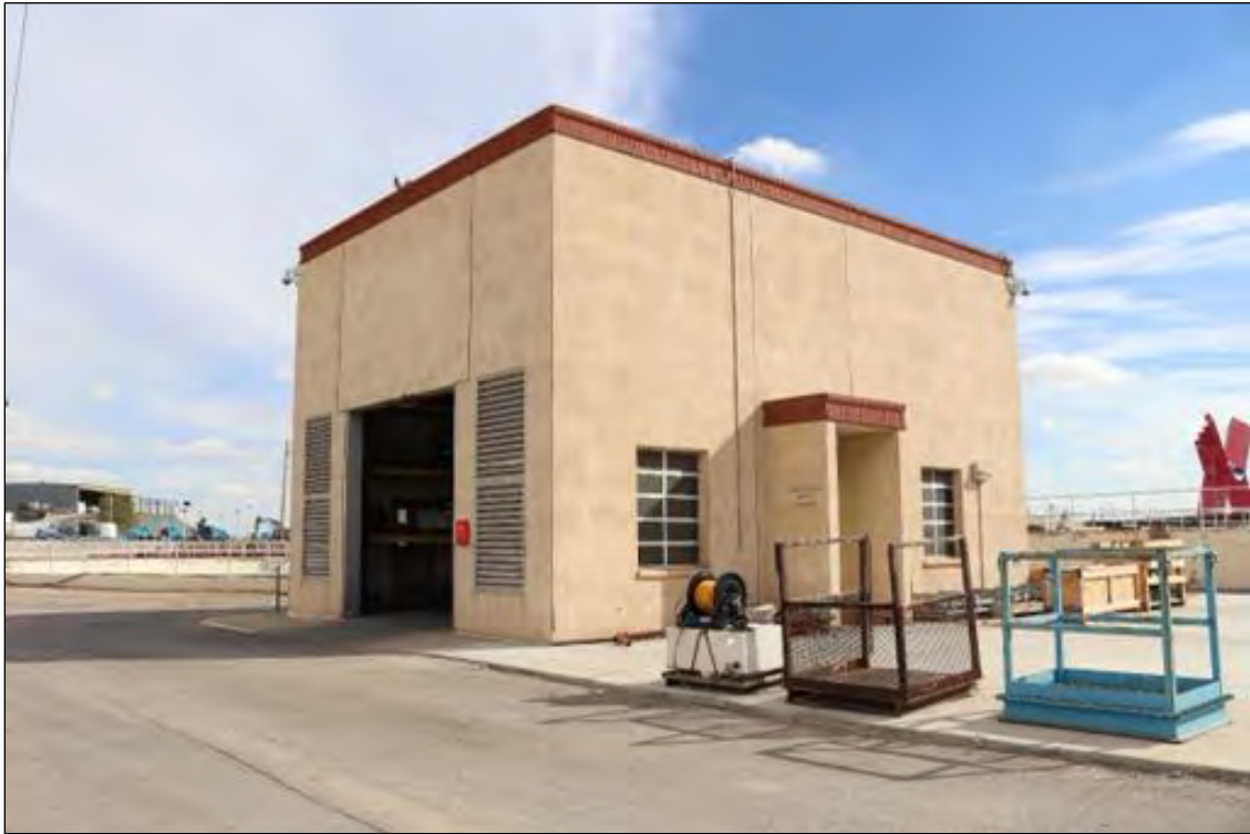
Figure 263. Oxygenation Supply System Building, looking southeast.
