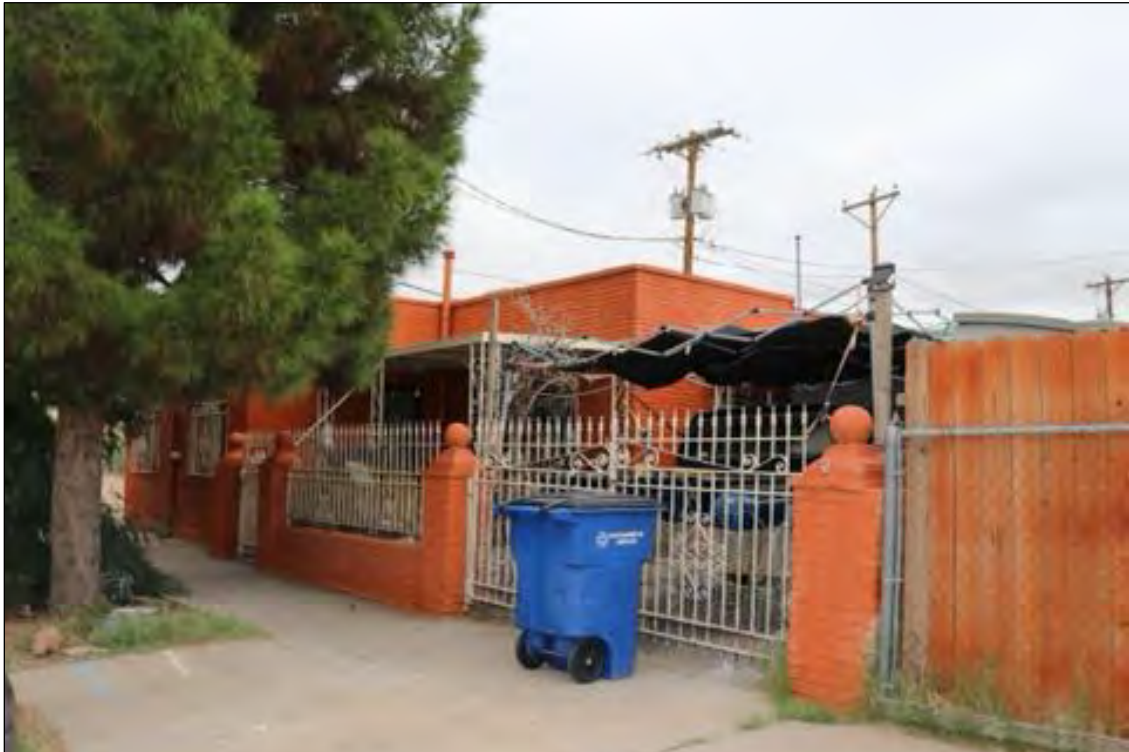
Figure 169. 418 Stevens Street (Residence) rear, looking east.
