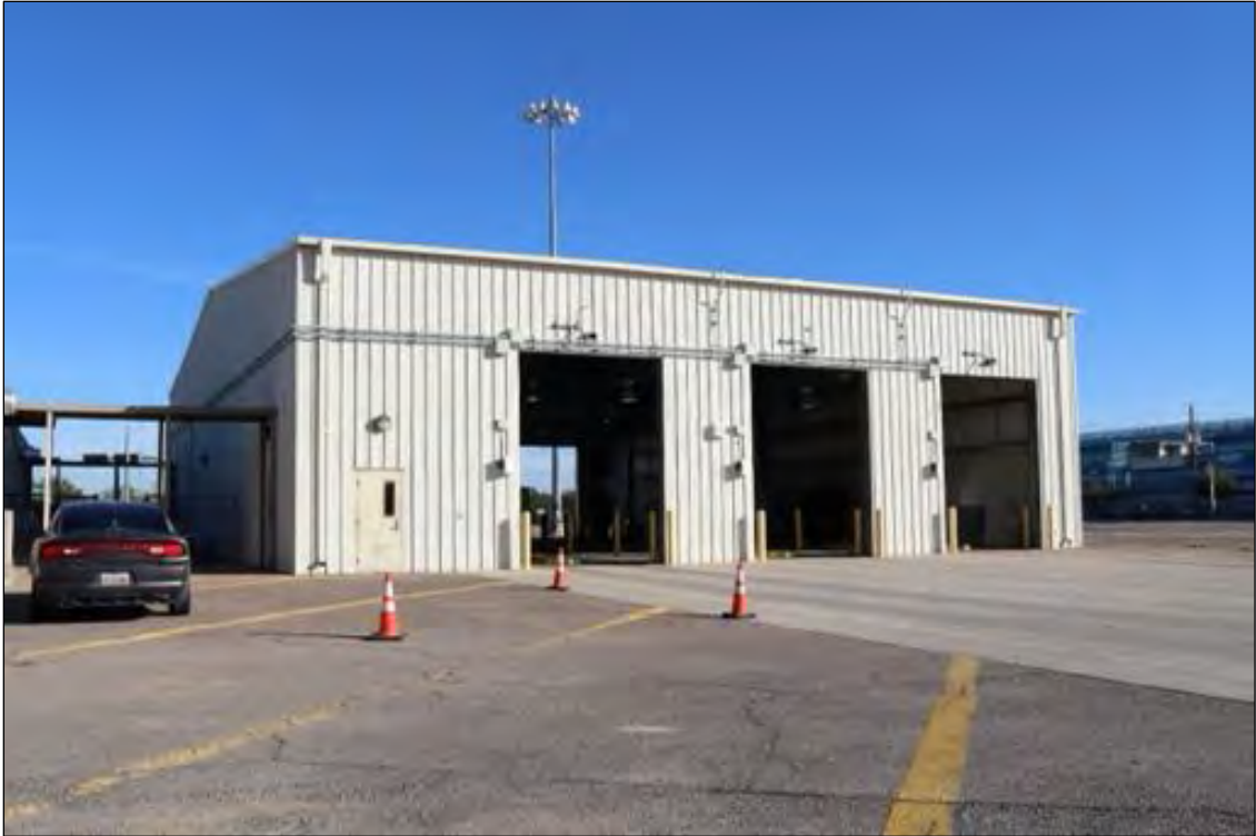
Figure 207. 4000 E Paisano Drive (Inspection Shed), looking northeast.
