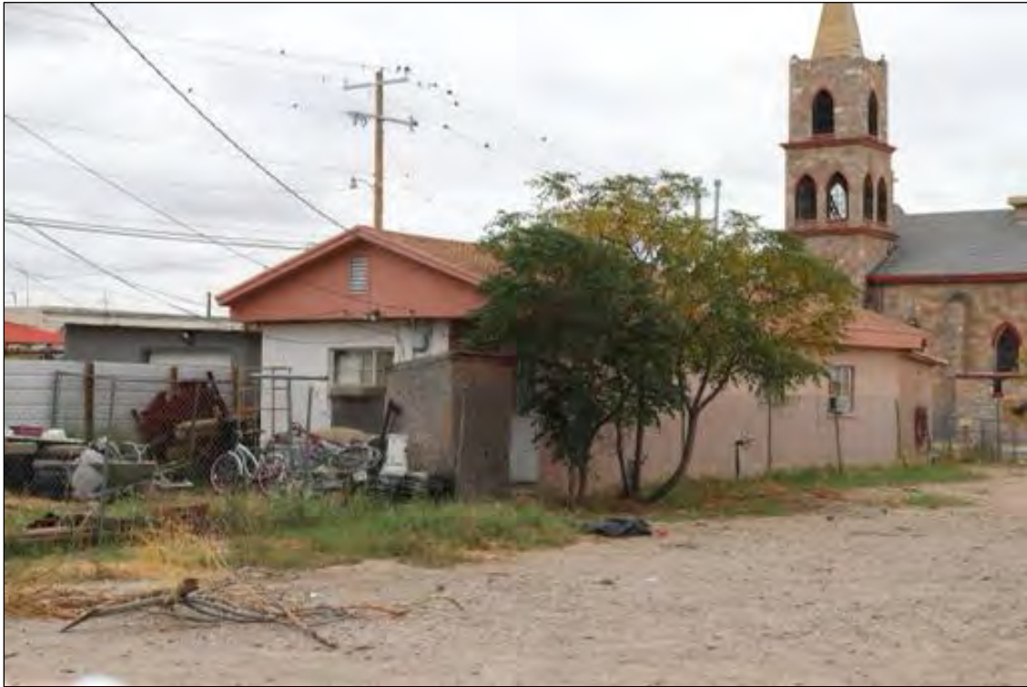
Figure 146. 3733 Findley Avenue (Residence) rear, looking southeast.
