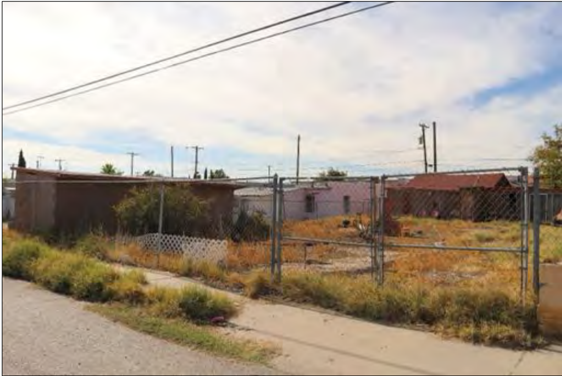
Figure 90. 208 Hardesty Place (Residence) rear, looking southwest.
