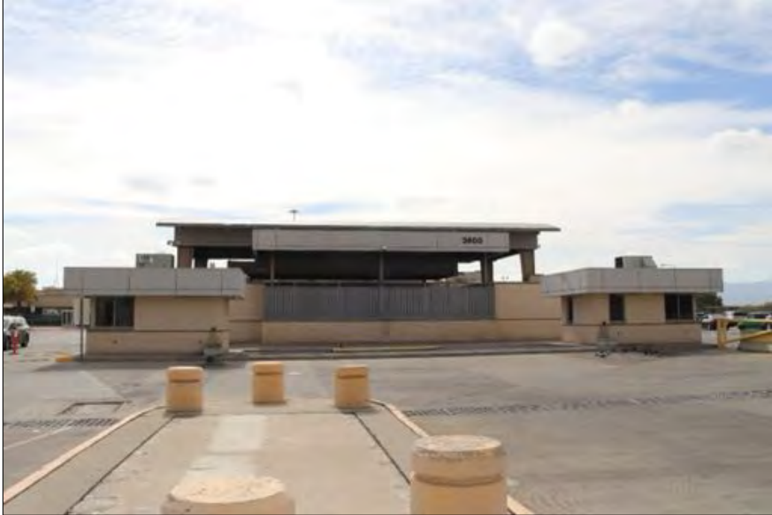
Figure 62. 3600 E Paisano Drive (Building C Head House and TAC Booths), looking southwest.
