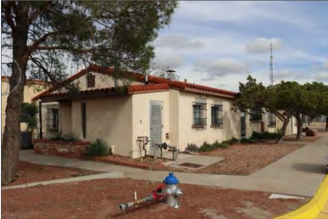
Figure 248. Office, looking northwest.
