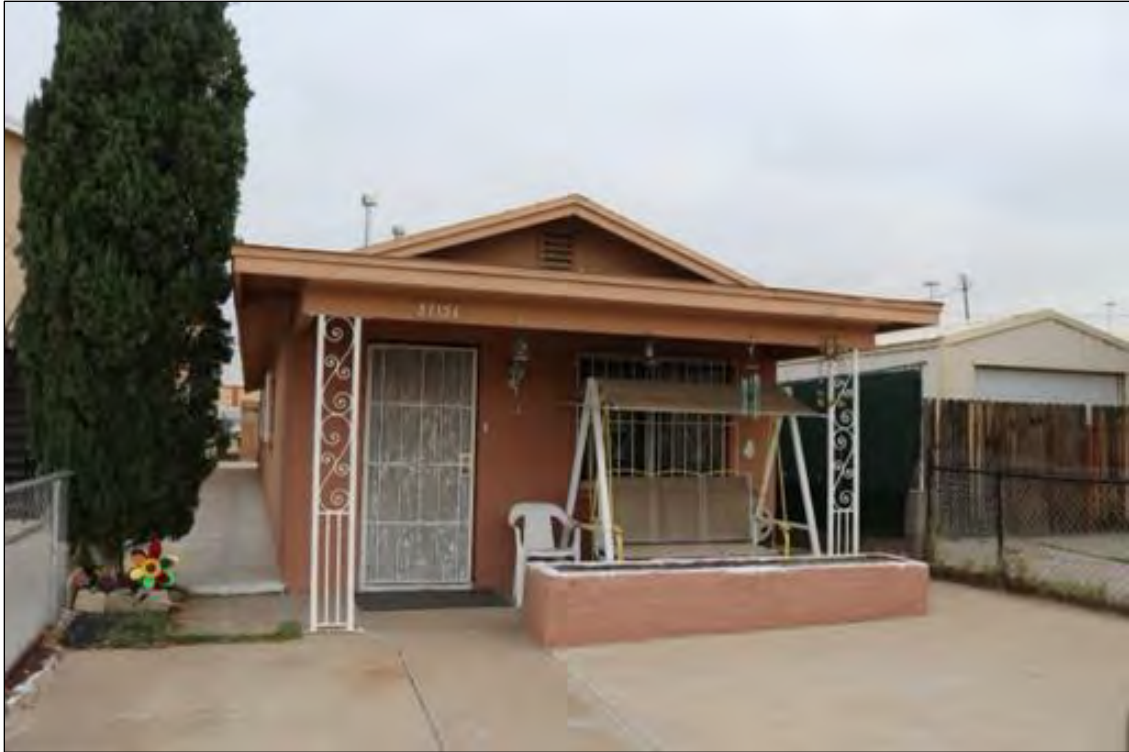
Figure 137. 3715 ½ Findley Avenue (Residence), looking north.
