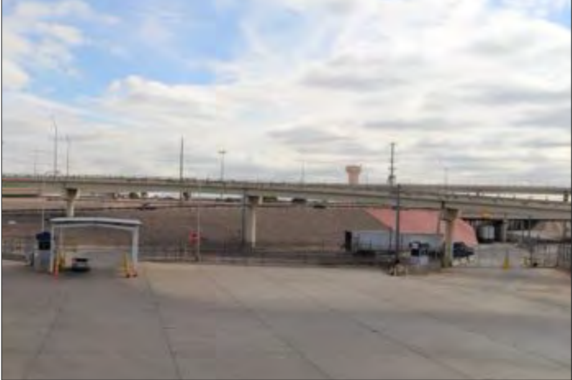
Figure 73. 3600 E Paisano Drive (Truck Exit Booth), northern booth on the left and southern booth on the right, looking southwest.
