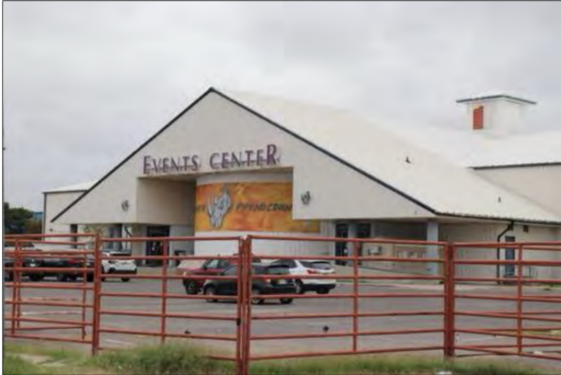
Figure 231. El Paso Events Center, looking southeast.
