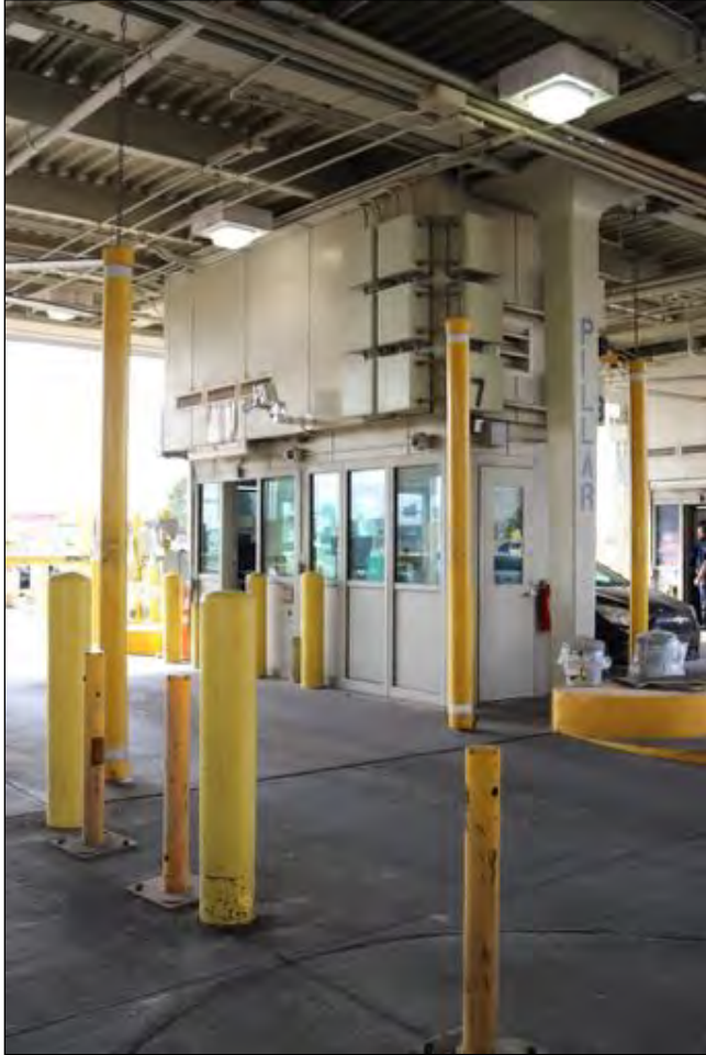
Figure 128. 3600 E Paisano Drive (Building K Primary/Secondary Inspection Canopy), Primary Inspection Canopy booth, looking southwest.
