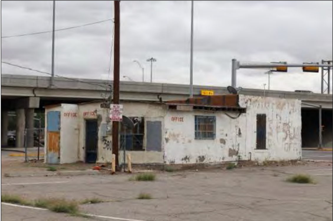
Figure 170. 3809 E Paisano Drive, looking southeast.
