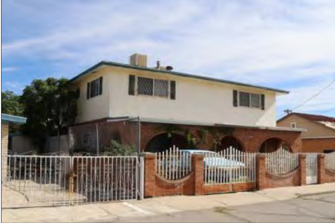
Figure 108. 224 Hardesty Place (Residence), looking southeast.
