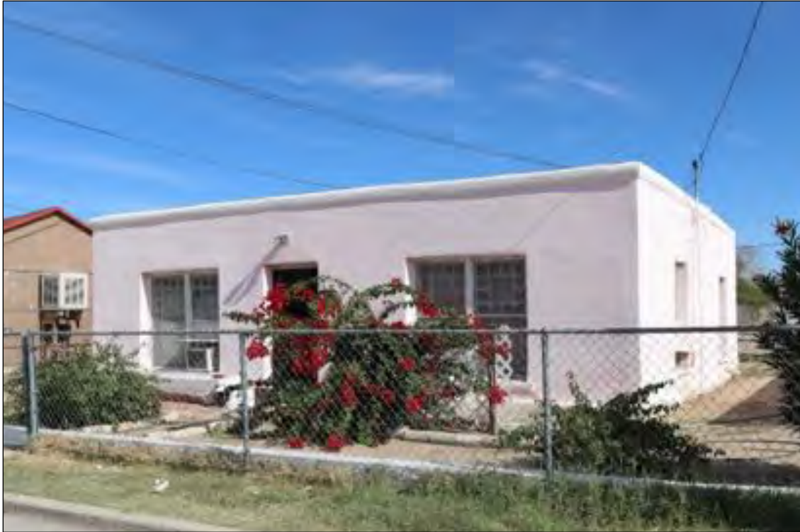
Figure 92. 210 Hardesty Place (Residence), looking northeast.
