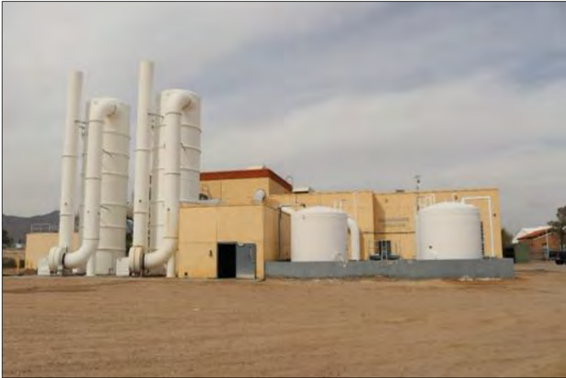
Figure 255. Headworks Building, looking north.
