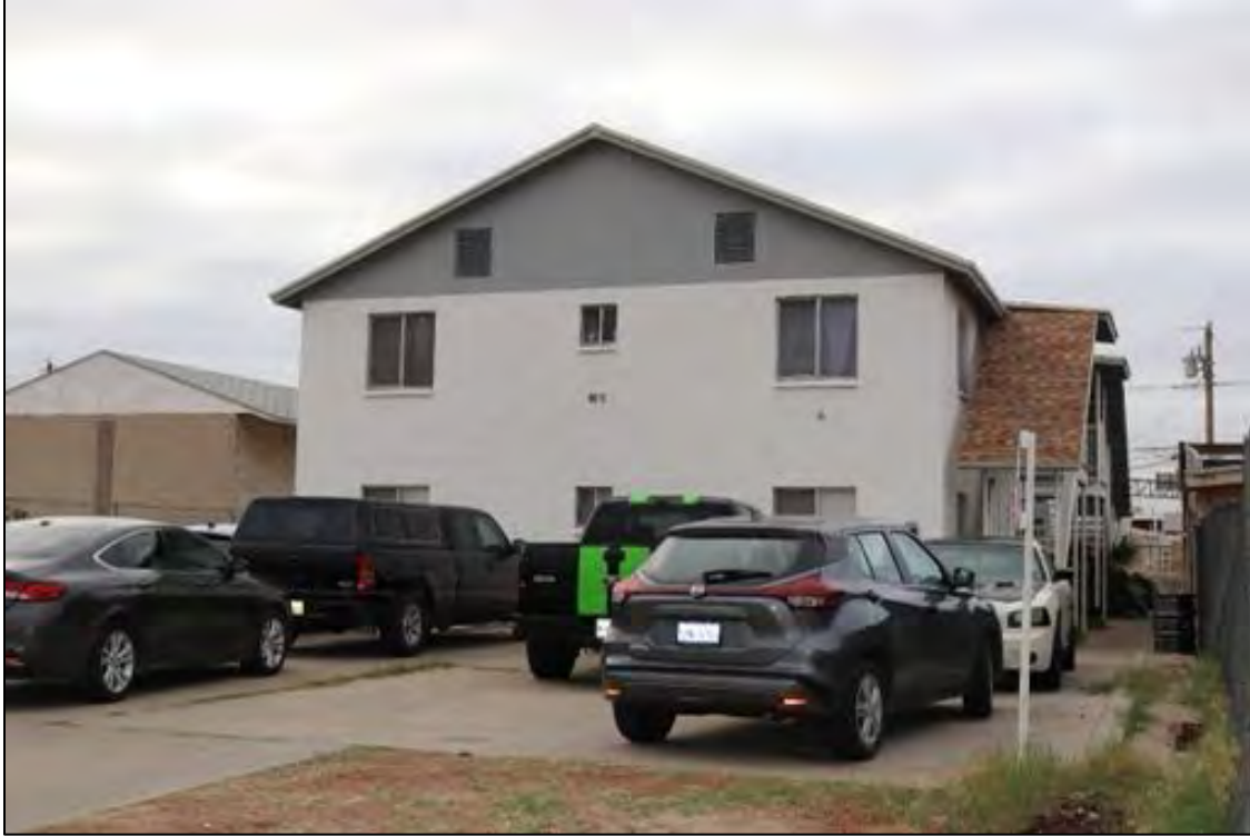
Figure 41. 4006 Laredo Avenue (Residence), looking south.
