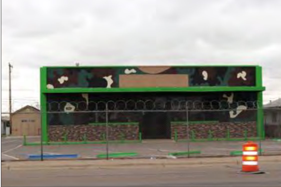
Figure 27. 3922 Delta Drive, looking south.
