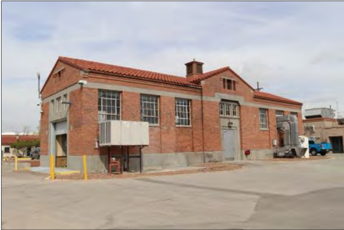
Figure 251. Shop, former Pump House, looking northeast.
