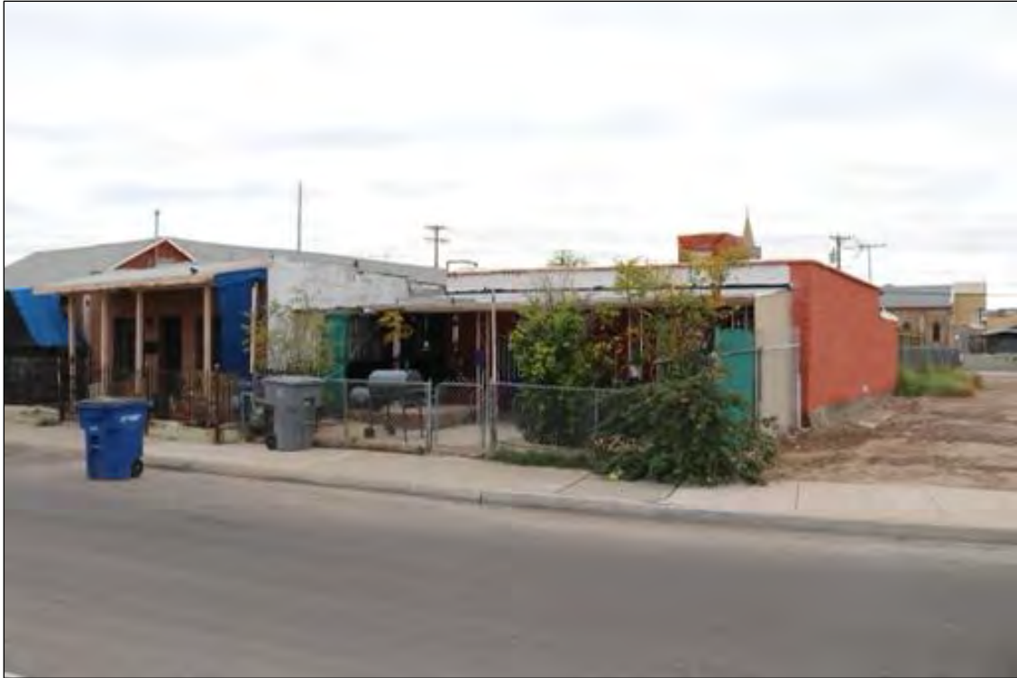
Figure 176. 3720 E San Antonio Avenue (Residence), looking southeast. Note that it is connected to 3722 E San Antonio (on the left).
