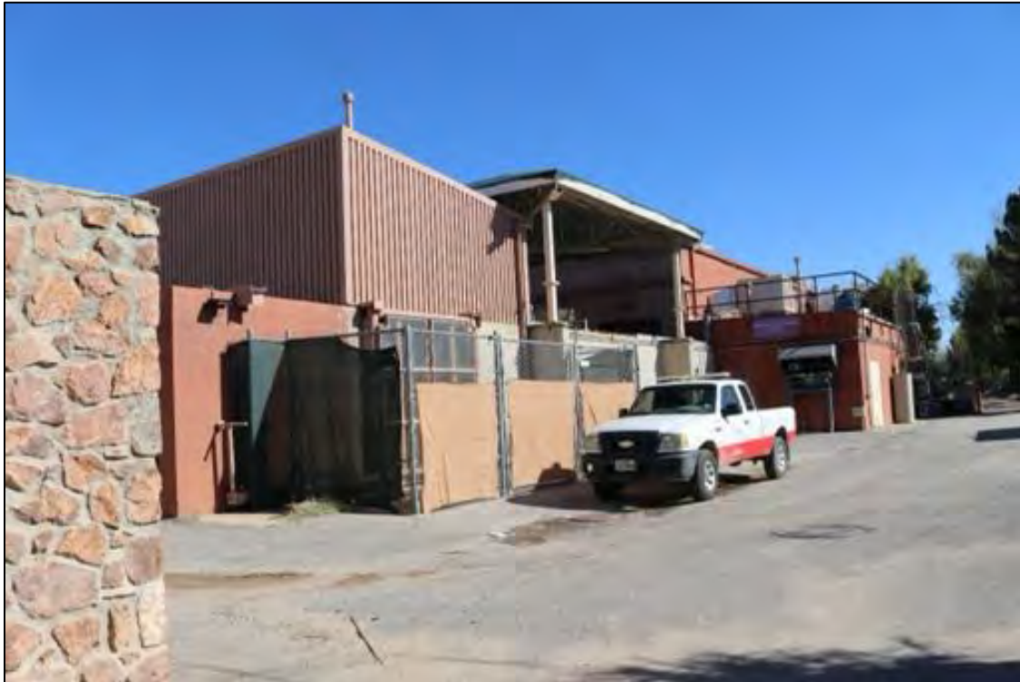
Figure 243. Elephant Barn Complex, looking northeast.
