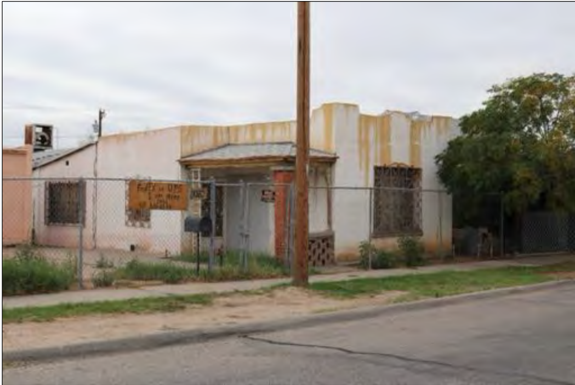
Figure 182. 3726 E San Antonio Avenue (Residence), looking southwest.
