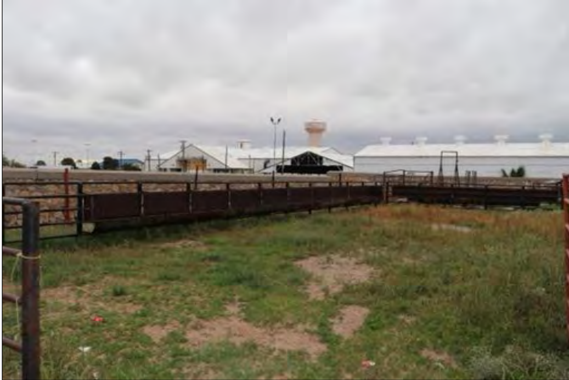
Figure 220. Coliseum Livestock barn coral, looking south.
