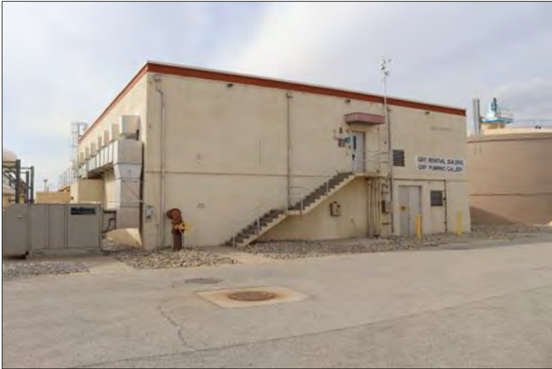
Figure 267. Grit Building, looking northwest.
