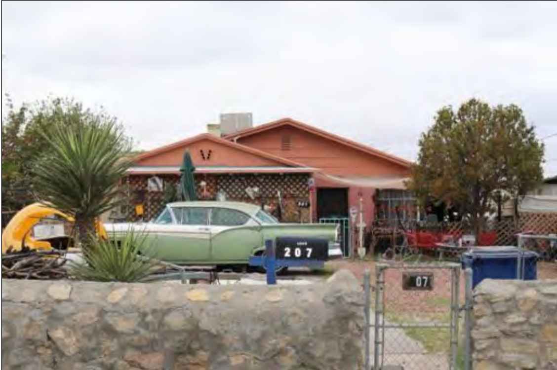
Figure 88. 207 Hardesty Place (Residence), looking east.
