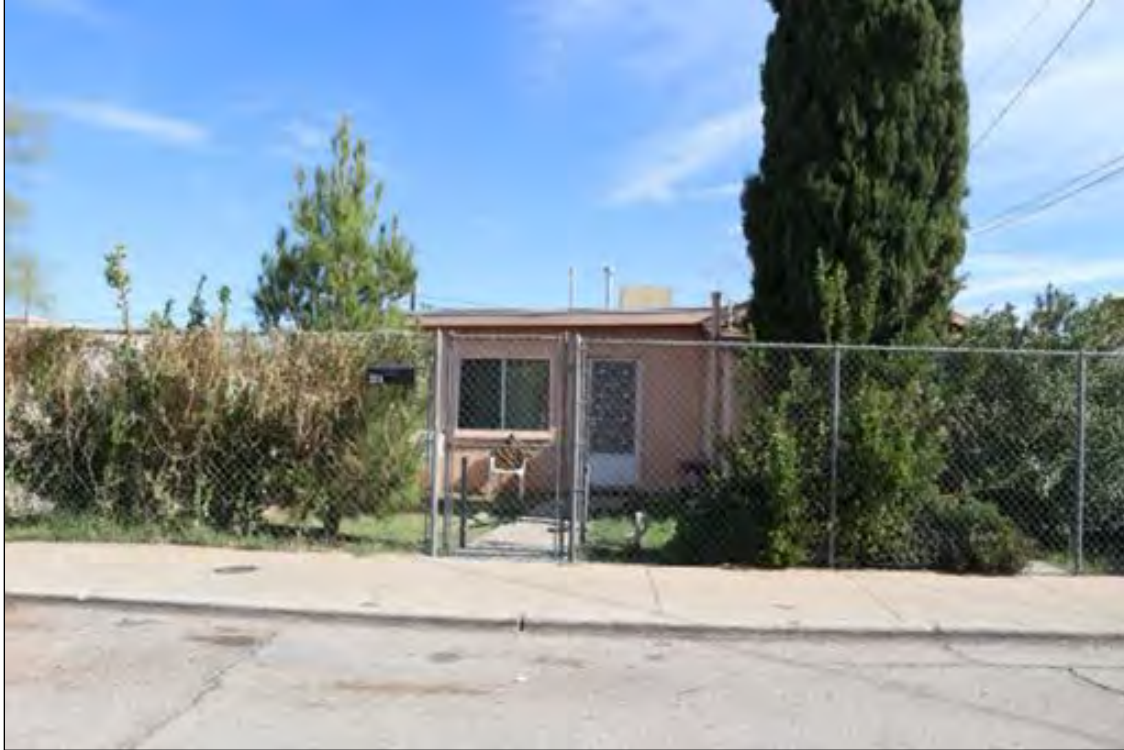
Figure 102. 218 Hardesty Place (Residence), looking east.
