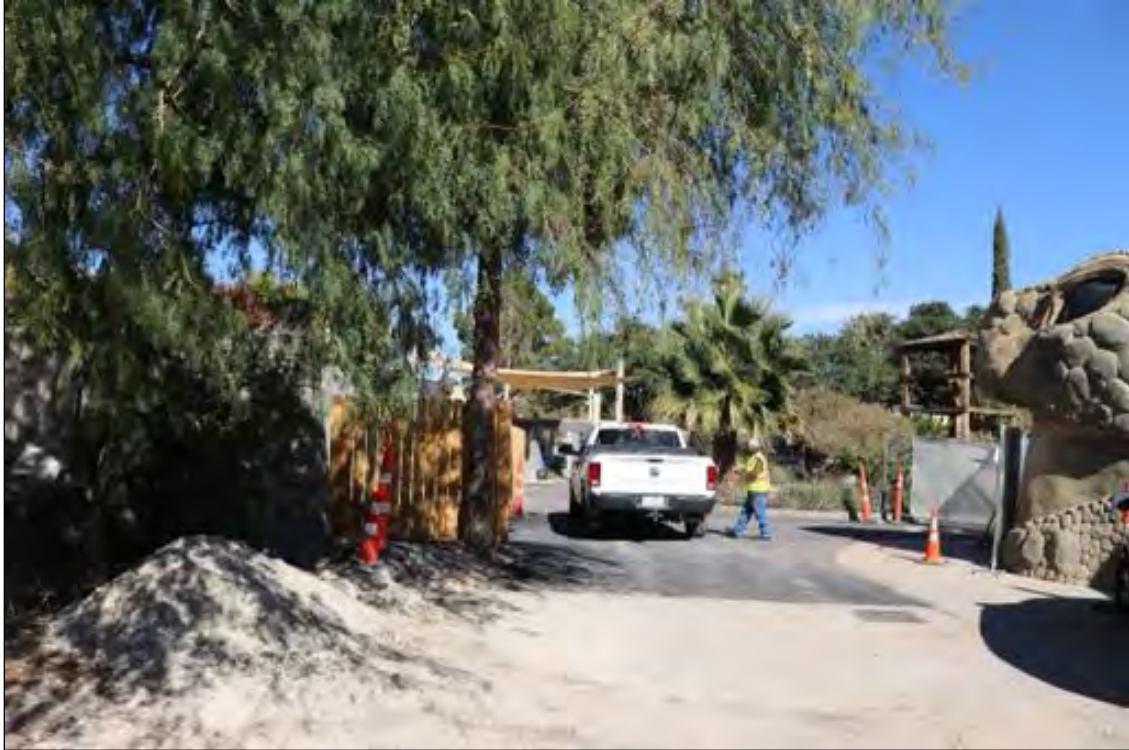
Figure 240. Holding, under construction, looking southwest.
