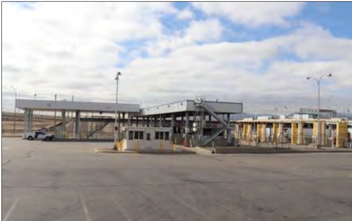
Figure 714. 3600 E Paisano Drive (Inbound Commercial Primary Inspection Canopy with Booth and Empty Truck Canopy), Empty Truck Canopy (left), Inbound Commercial Primary Inspection Canopy (right) and Booth (foreground), looking south.
