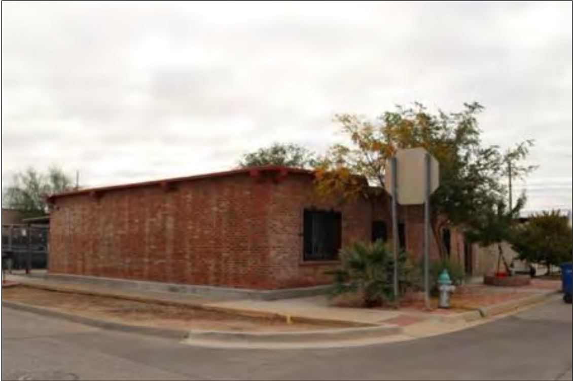
Figure 186. 3800 E San Antonio Avenue (Residence), looking southeast.
