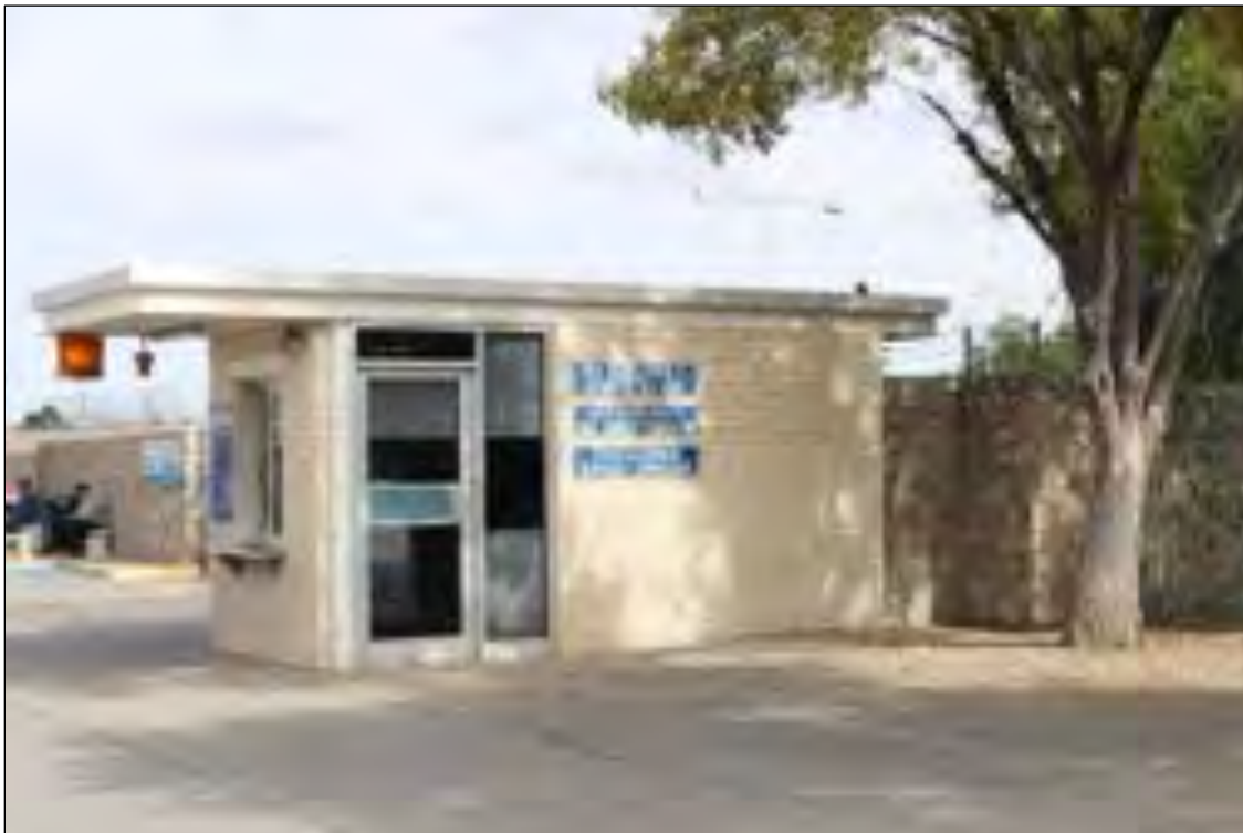
Figure 74. 3600 E Paisano Drive (TABC Booth), Pedestrian TABC Booth, looking northeast.
