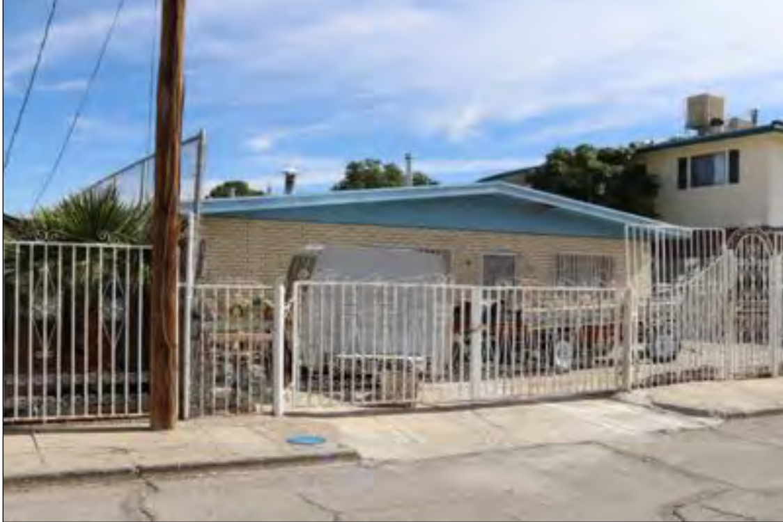
Figure 106. 222 Hardesty Place (Residence), looking east.
