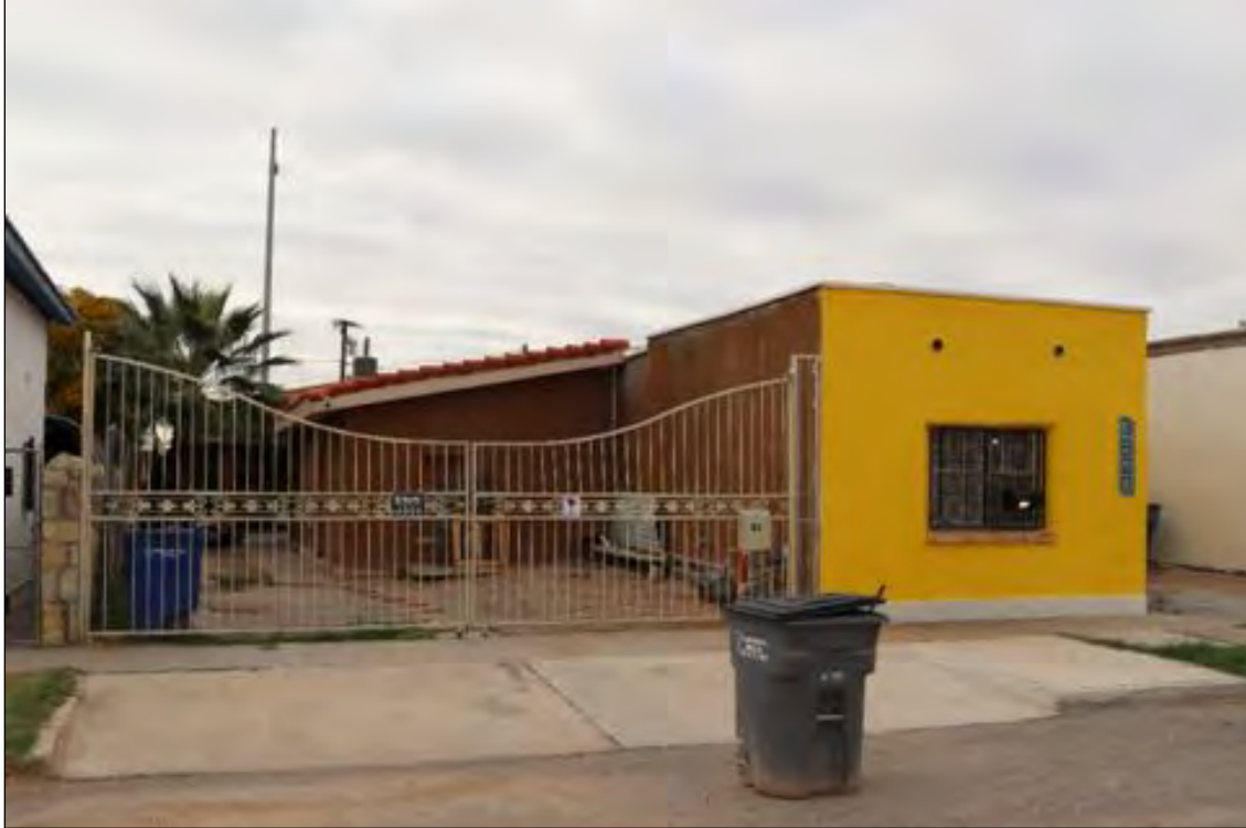
Figure 193. 3822 E San Antonio Avenue (Residence), looking southwest.
