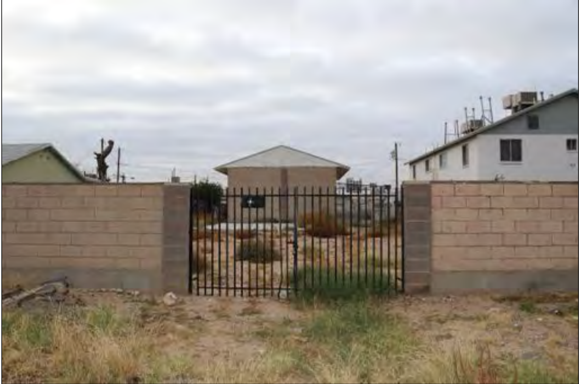
Figure 42. 4008 Laredo Avenue (Residence), looking south.
