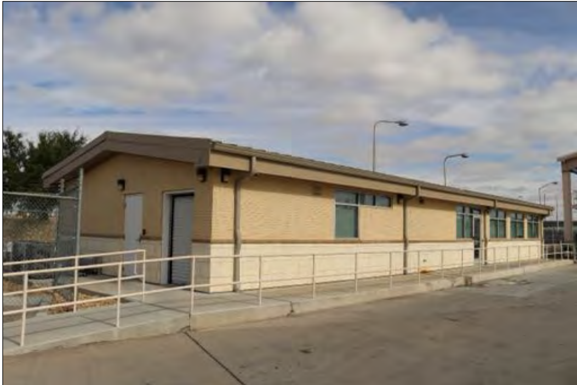
Figure 78. 3600 E Paisano Drive (FMCSA Administration Building), looking northwest.
