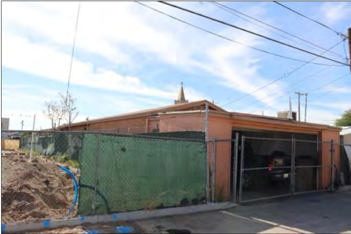
Figure 154. 3809 Findley Avenue (Residence) rear, looking southwest.
