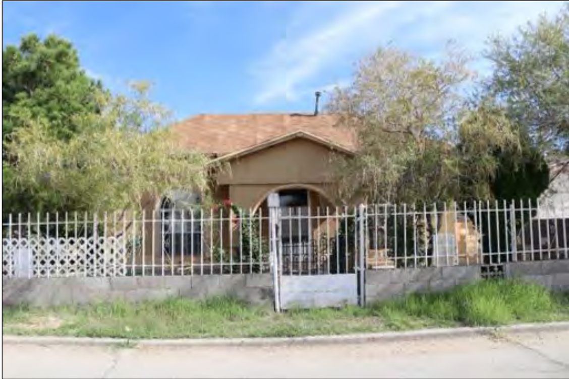
Figure 83. 200 Hardesty Place (Residence), looking east.
