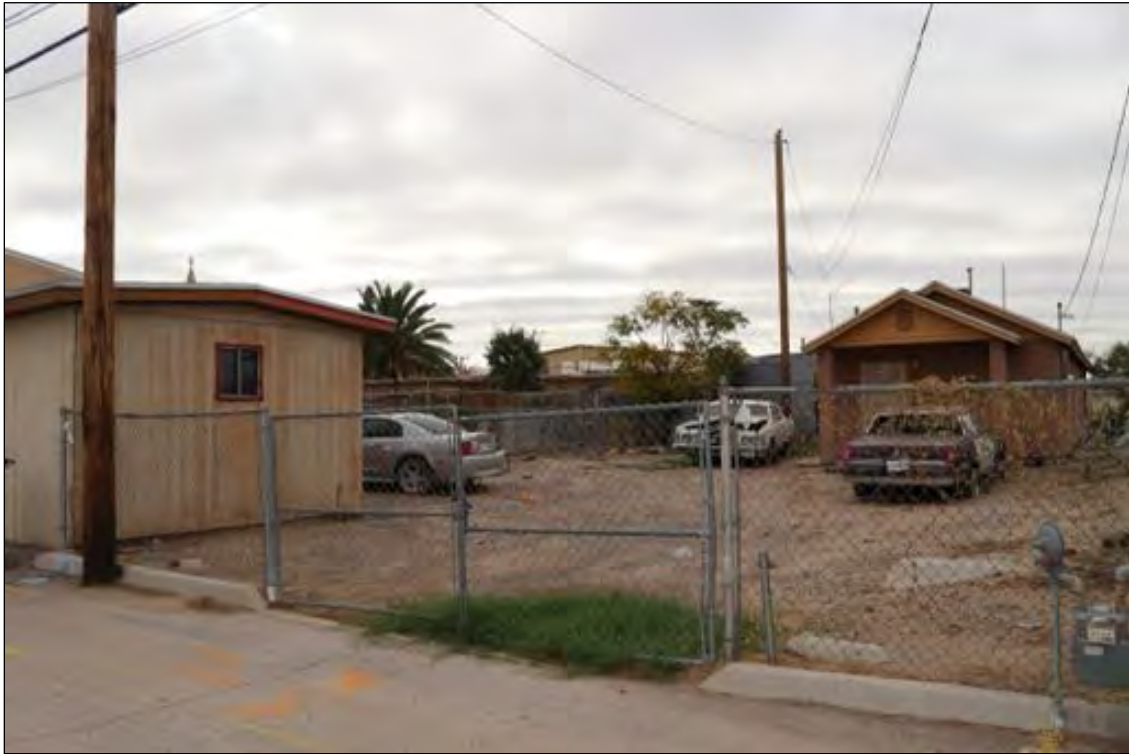
Figure 130. 3703 Findley Avenue (Residence) rear, looking south.
