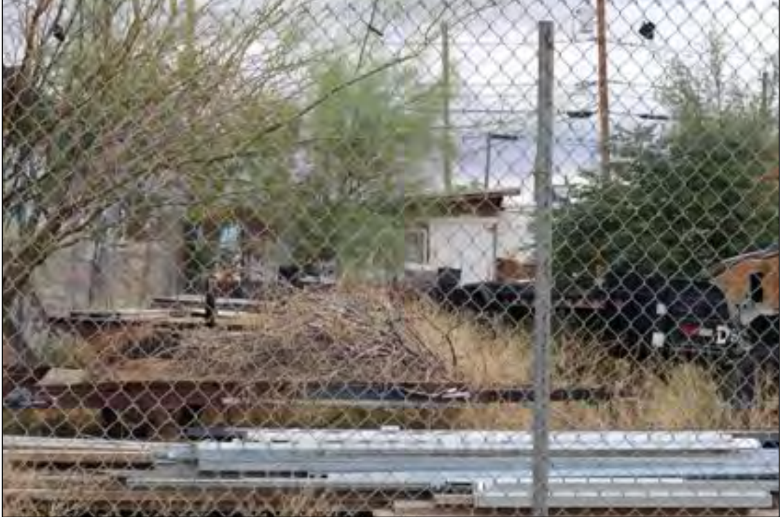
Figure 40. 4003 Laredo Avenue (Residence), looking north.
