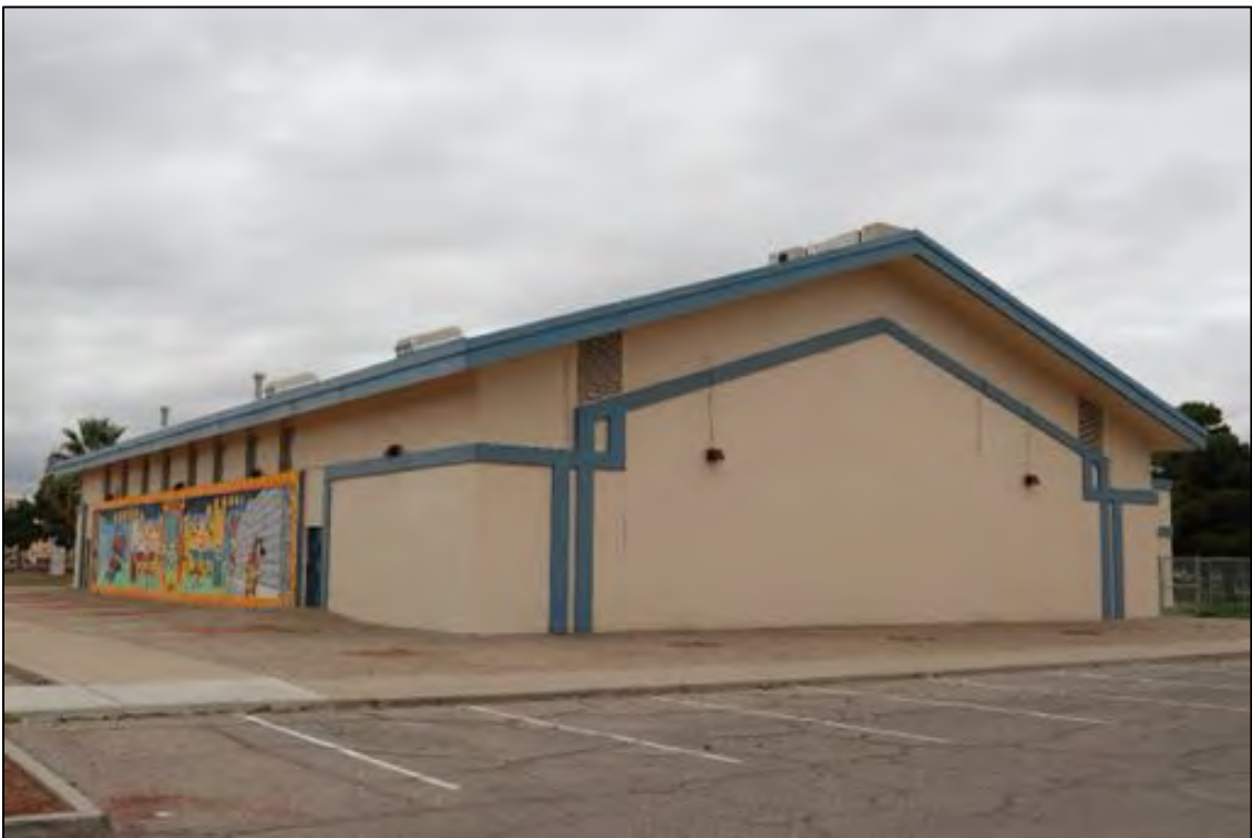
Figure 16. 4321 Delta Drive (Acosta Sports Center), looking southwest.
