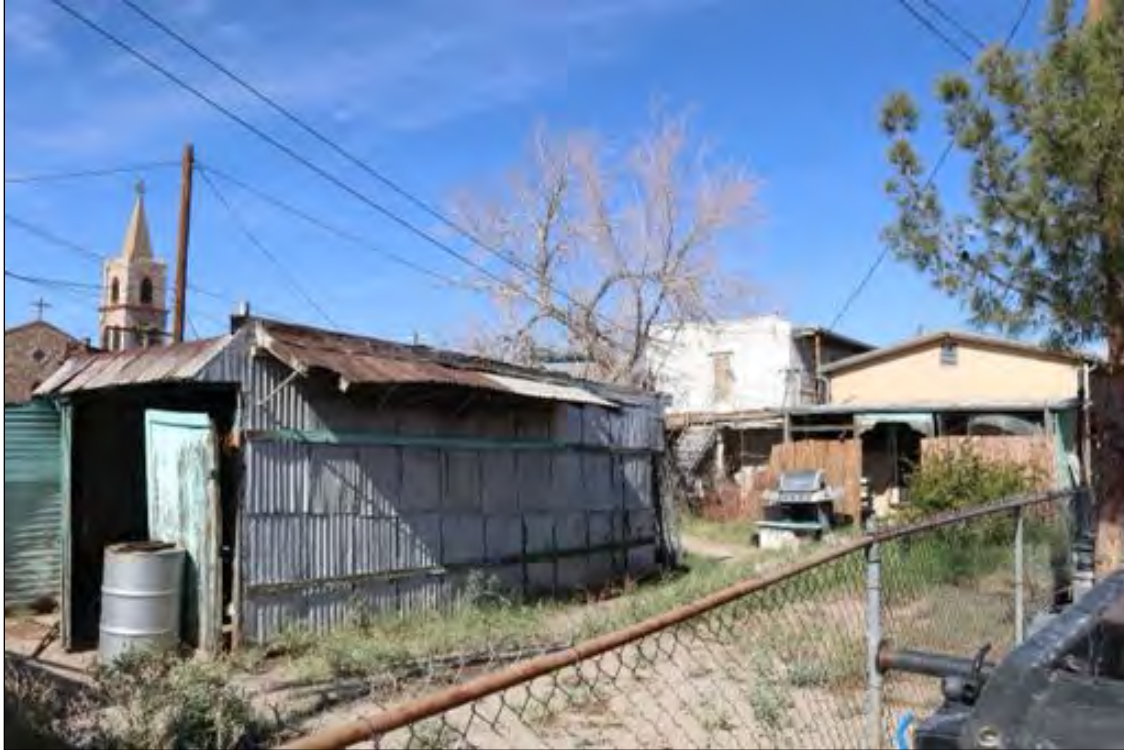
Figure 158. 3812 Findley Avenue (Residence) rear, looking southwest.
