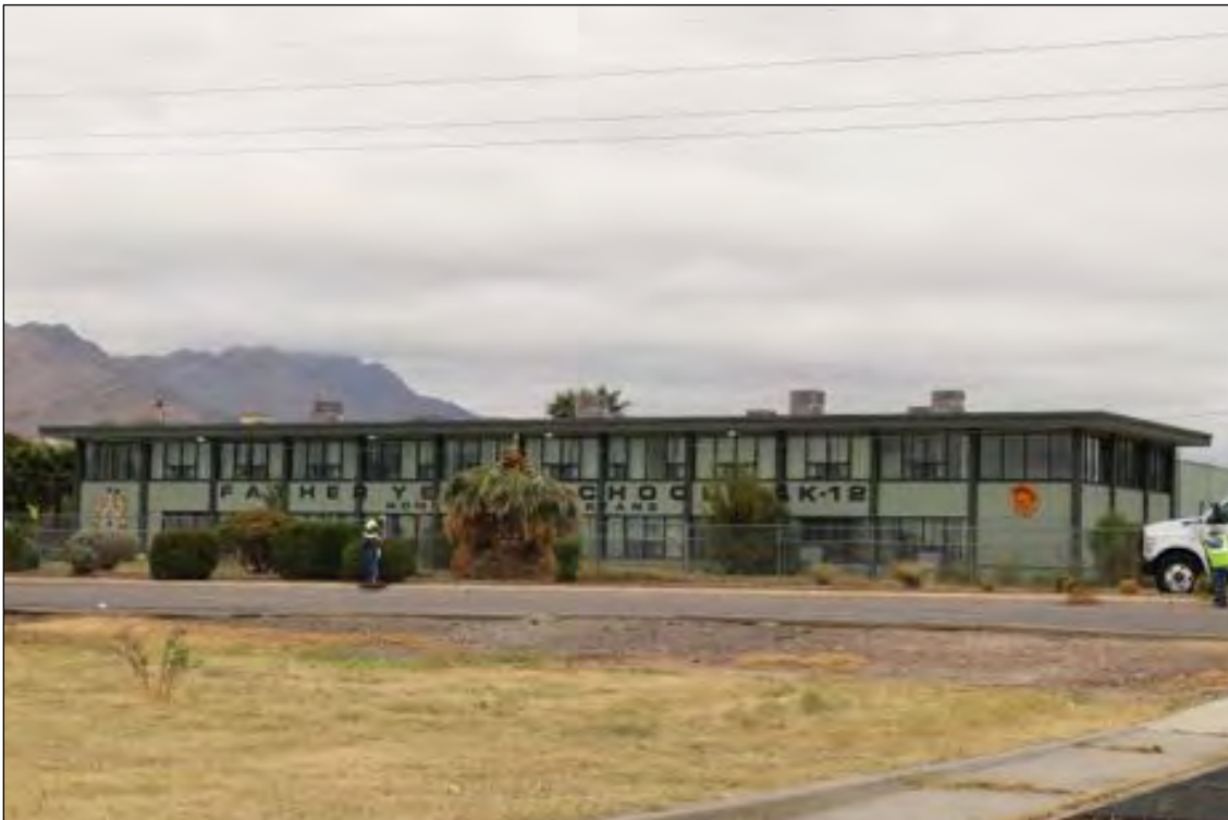
Figure 10. 200 Washington Street (Father Yermo High School), looking north.
