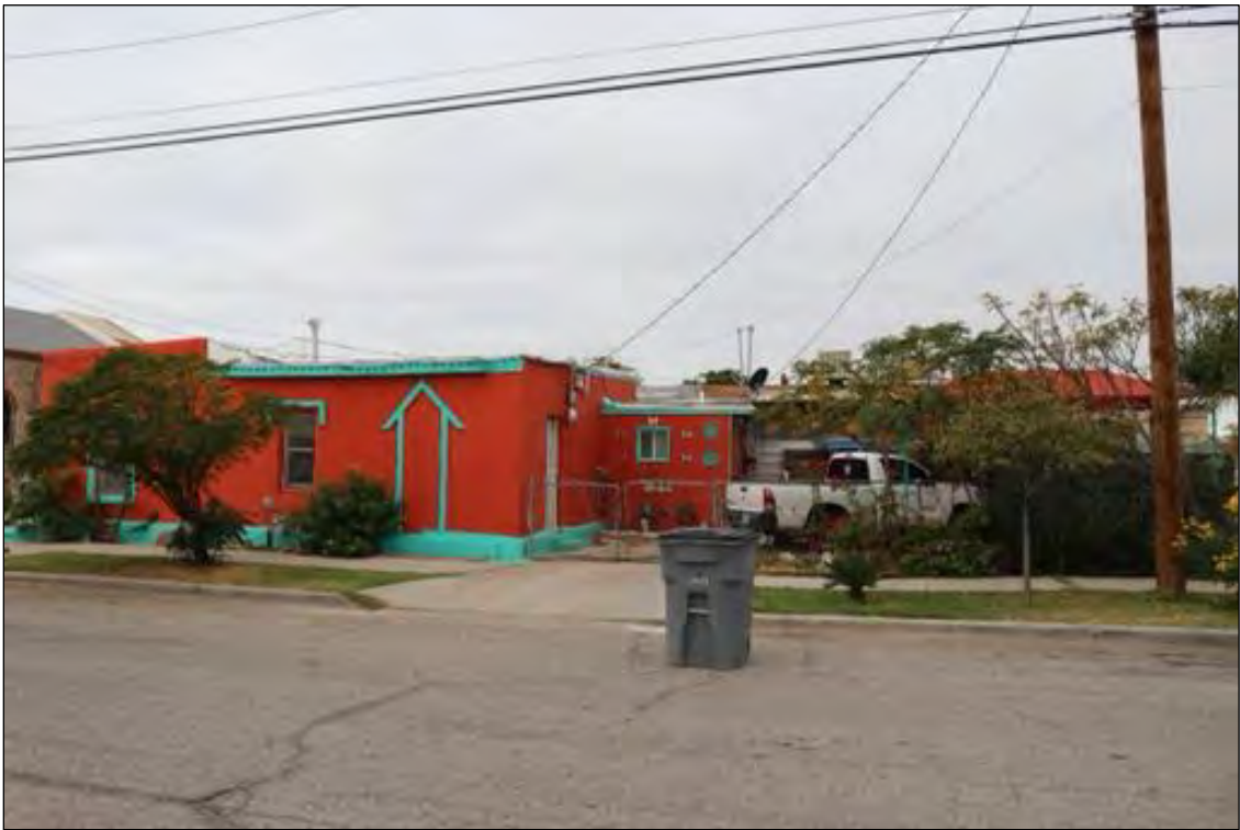
Figure 150. 3737 Findley Avenue (Residence) rear, looking west.
