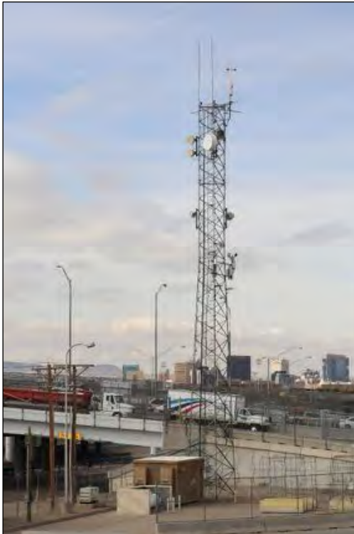
Figure 75. 3600 E Paisano Drive (RVSS Tower), looking west.
