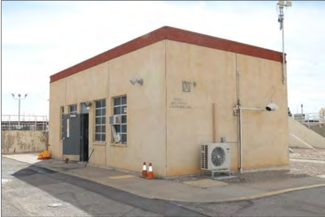
Figure 262. Oxygen Generation Control Building, looking southwest.
