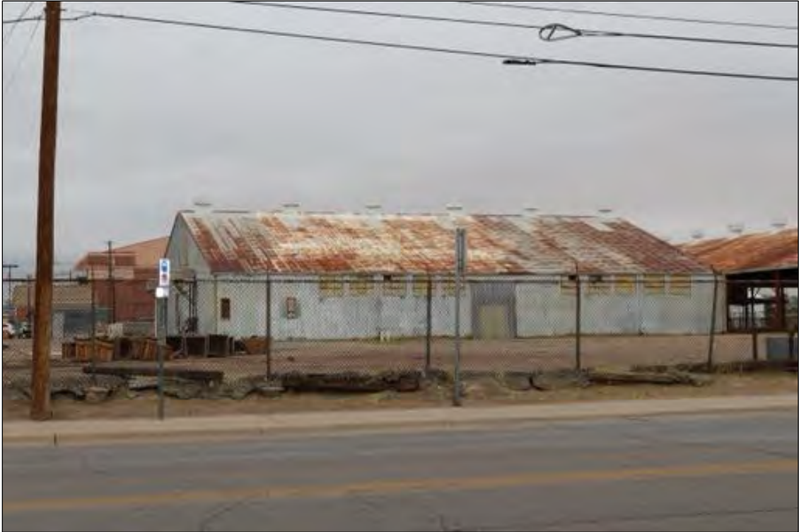
Figure 227. Holding Area Shelter, western wing, looking north.
