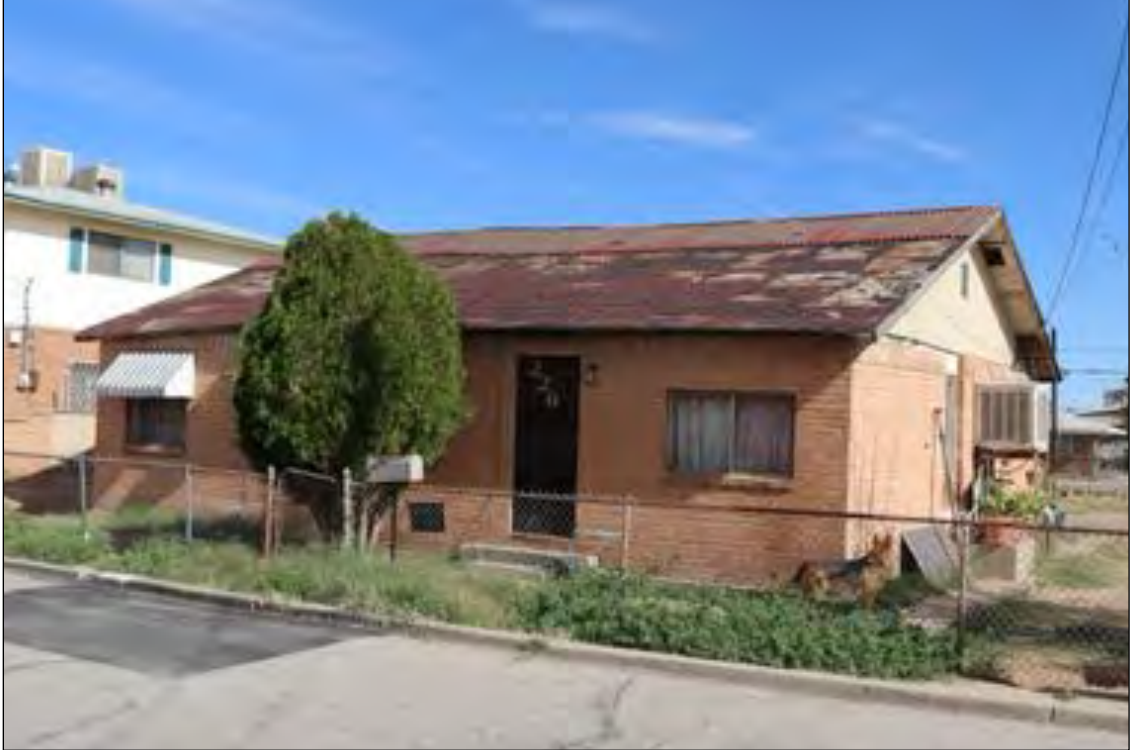
Figure 109. 226 Hardesty Place (Residence), looking northeast.
