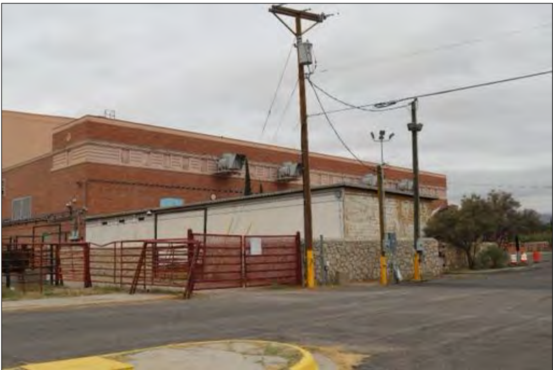
Figure 213. El Paso County Coliseum, looking northwest.
