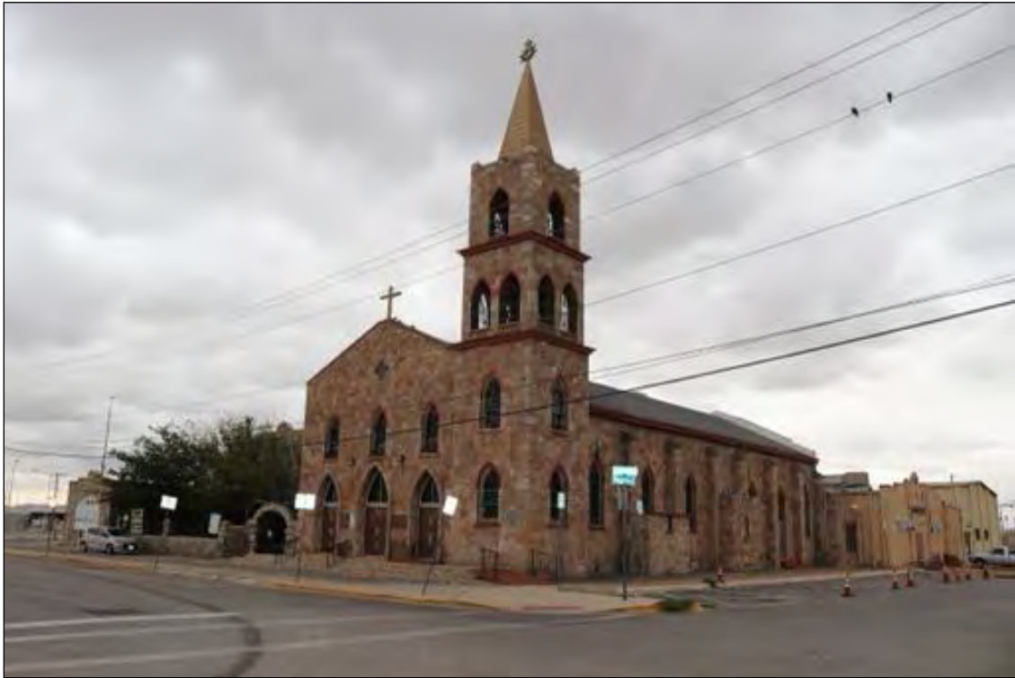
Figure 124. 519 S Latta (Saint Francis Xavier Church), looking southwest.
