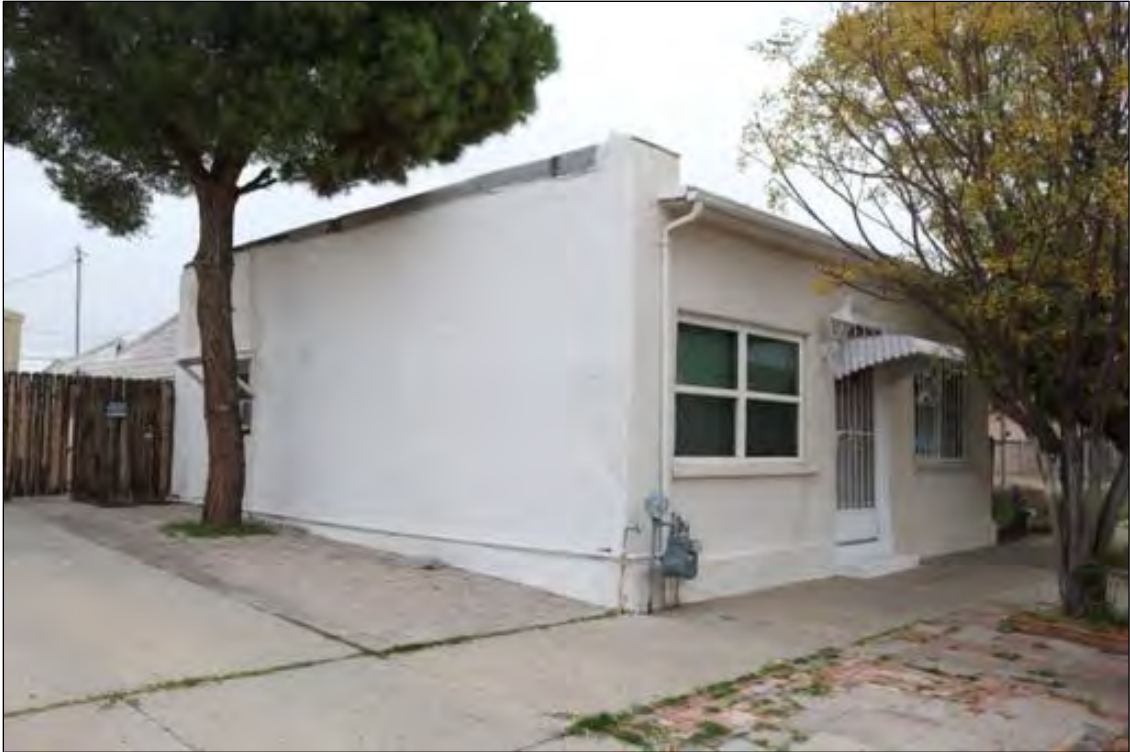
Figure 141. 3719 Findley Avenue (Residence), looking northeast.
