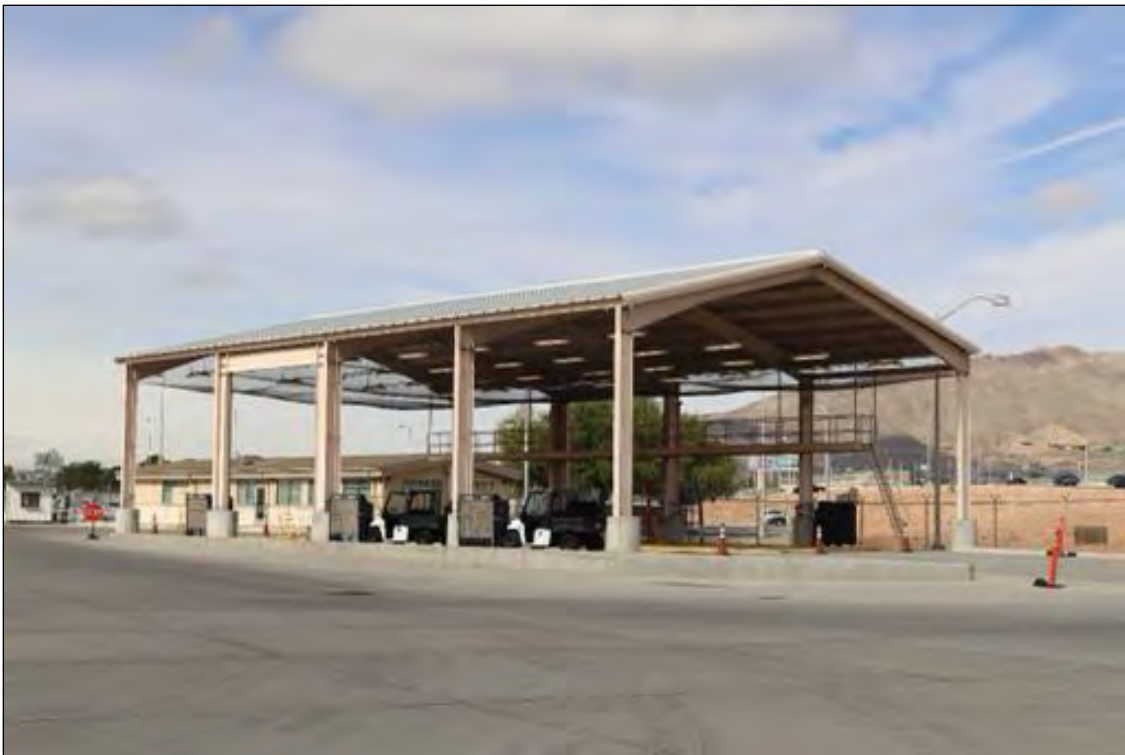
Figure 77. 3600 E Paisano Drive (FMCSA Inspection Canopy), looking northwest.
