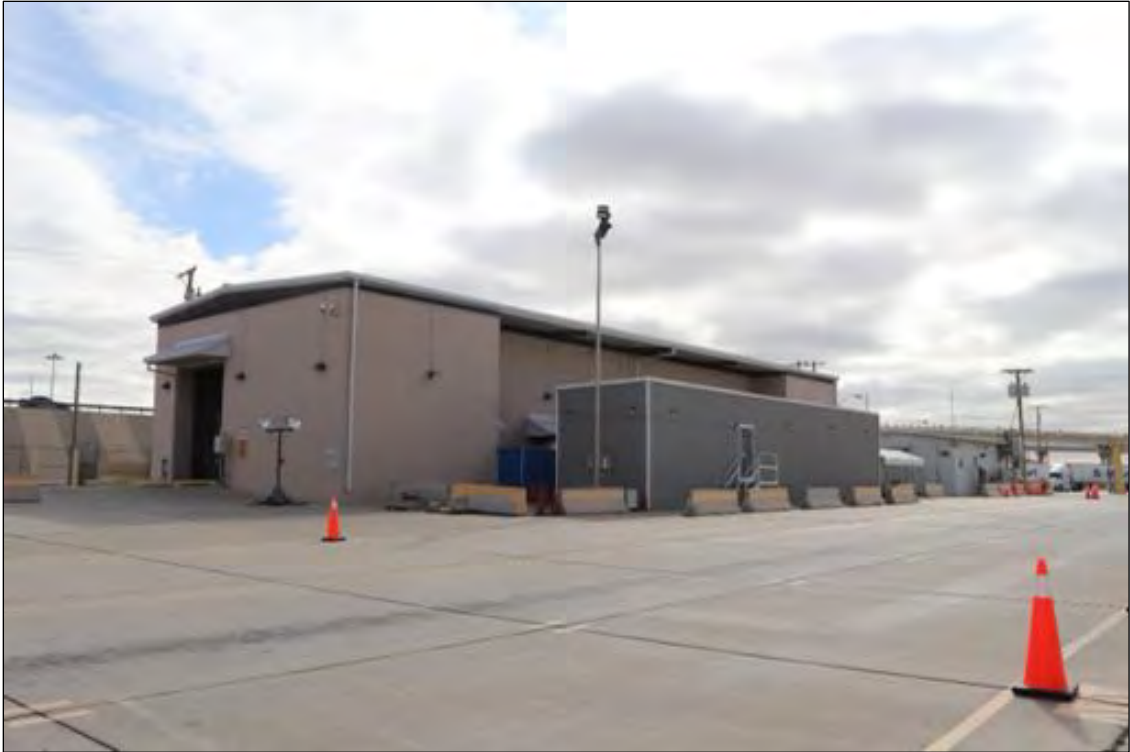
Figure 71. 3600 E Paisano Drive (VACIS), looking southeast.
