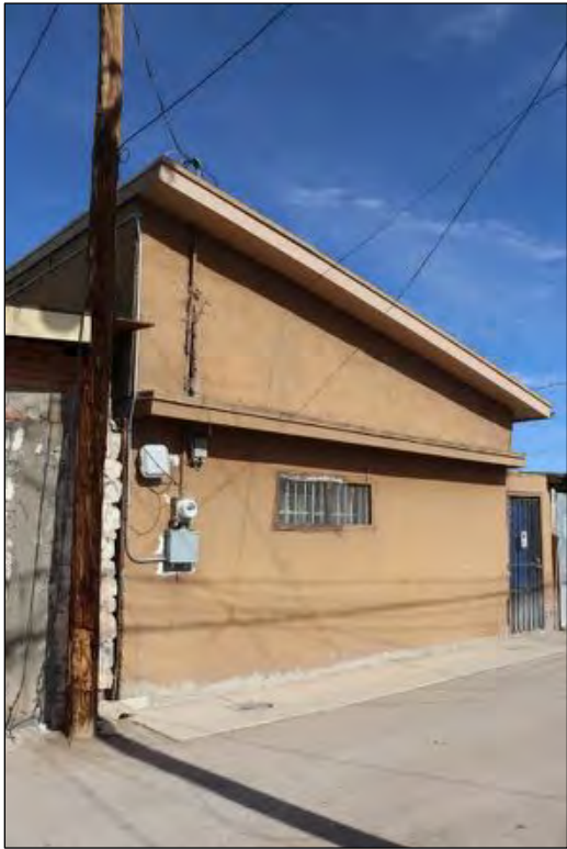
Figure 194. 3822 E San Antonio Avenue (Residence) rear, looking north.
