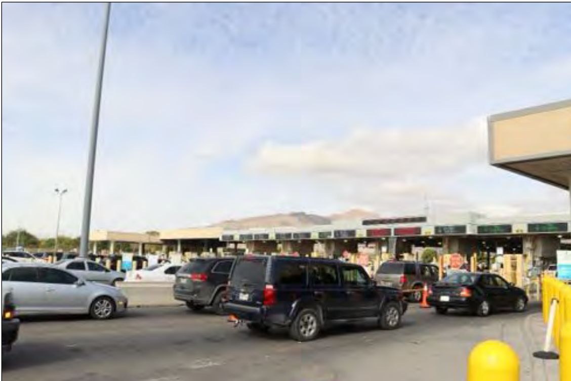
Figure 117. 3600 E Paisano Drive (Building K Primary/Secondary Inspection Canopy), south elevation of Primary Inspection Canopy (on the right), looking north.
