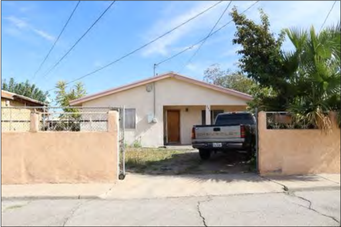
Figure 85. 202 Hardesty Place (Residence), looking east.
