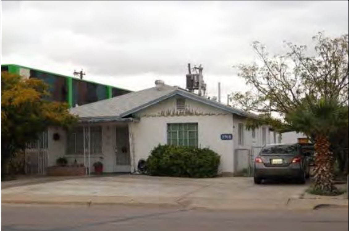
Figure 22. 3918 Delta Drive (Residence), looking south.
