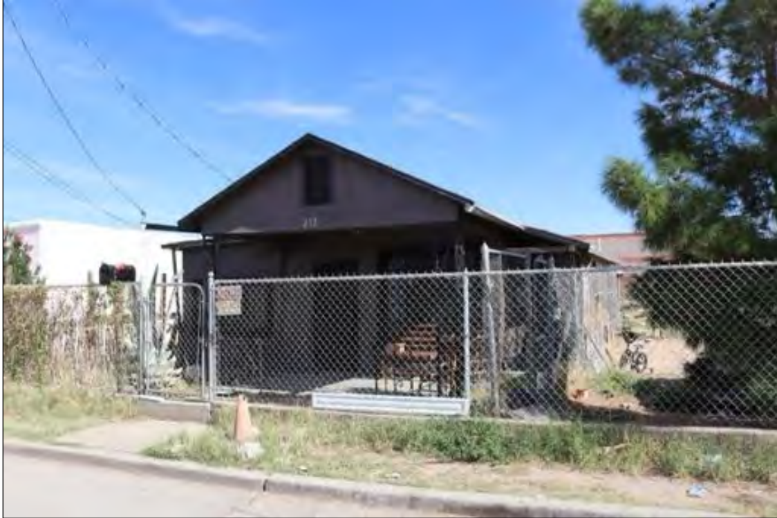
Figure 95. 212 Hardesty Place (Residence), looking northeast.
