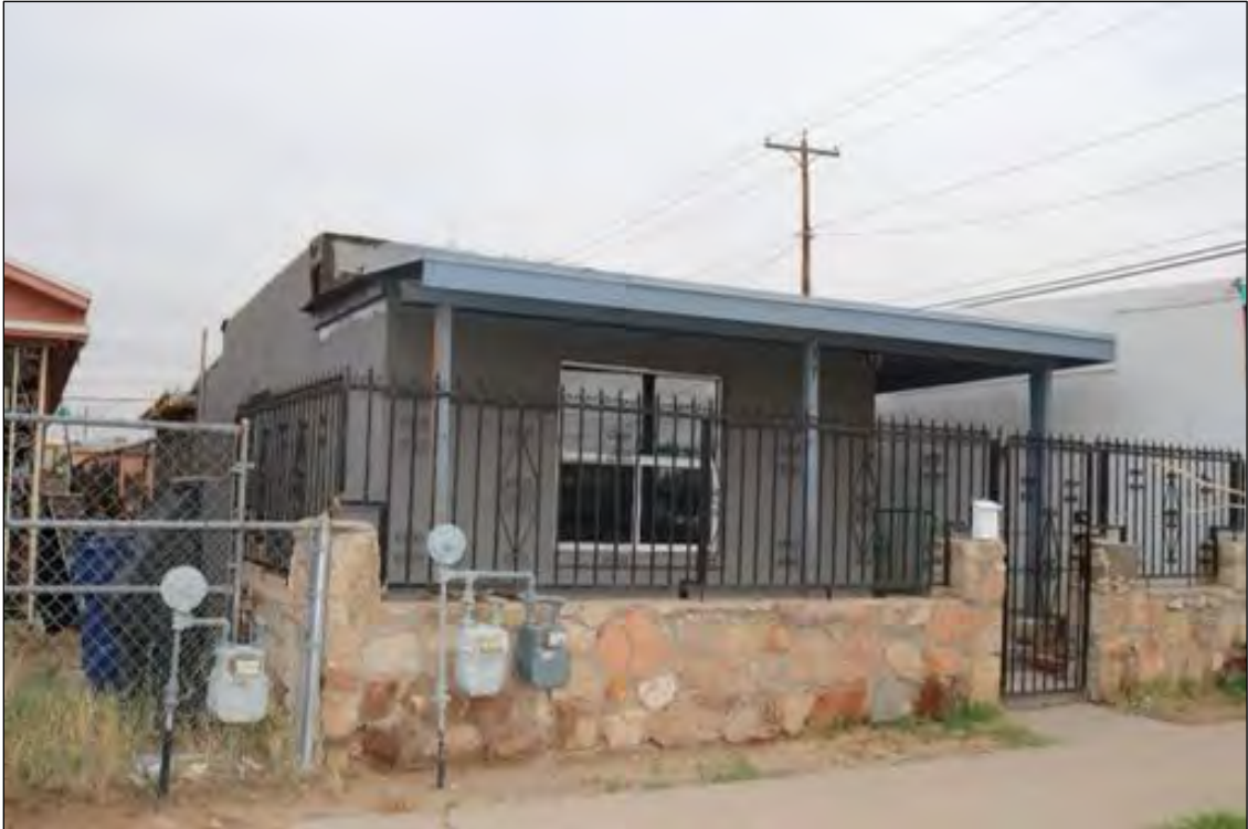
Figure 147. 3735 Findley Avenue (Residence), looking northeast.
