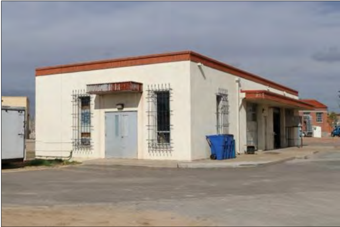
Figure 259. Electrical Shop, looking north.
