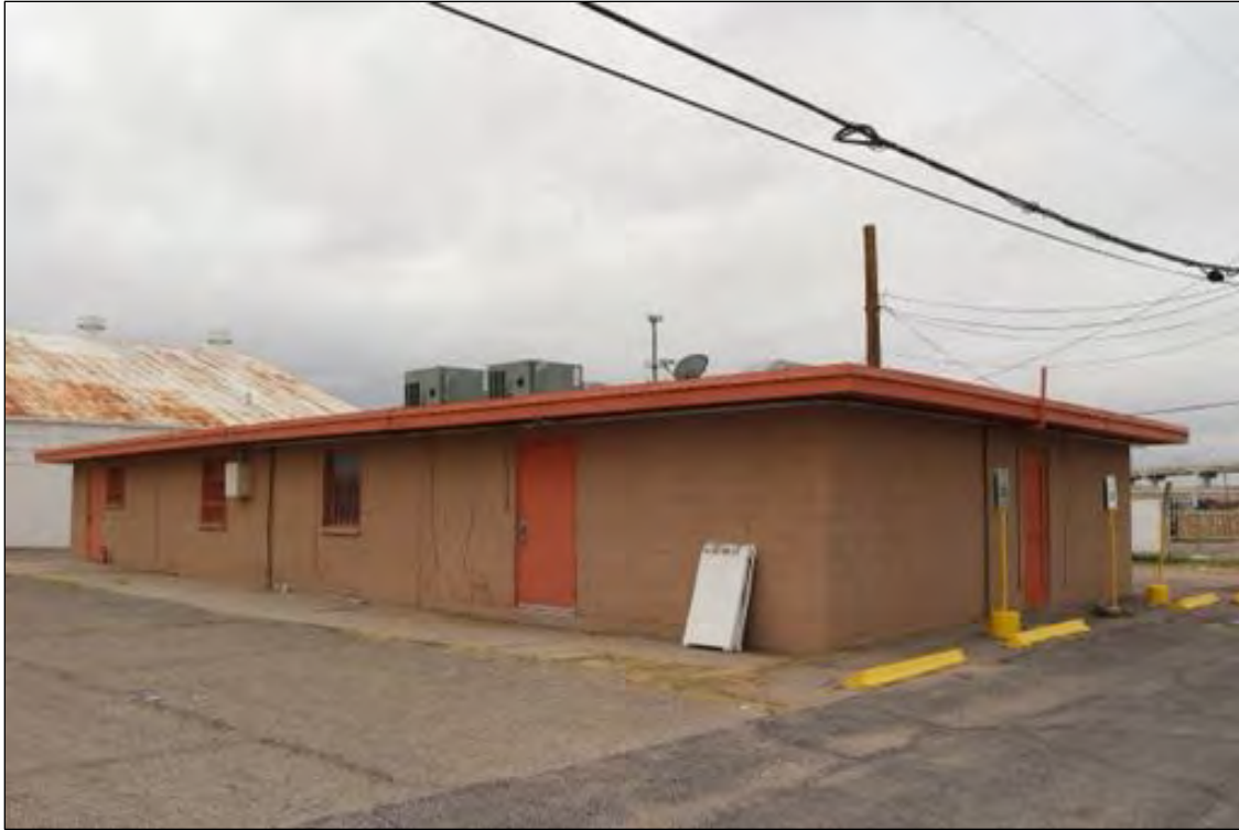
Figure 223. Accessory Building, looking southeast.
