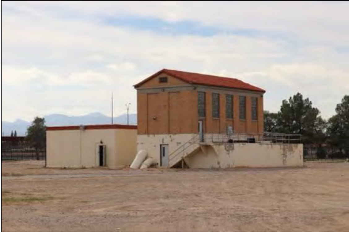
Figure 258. Building, looking southwest.
