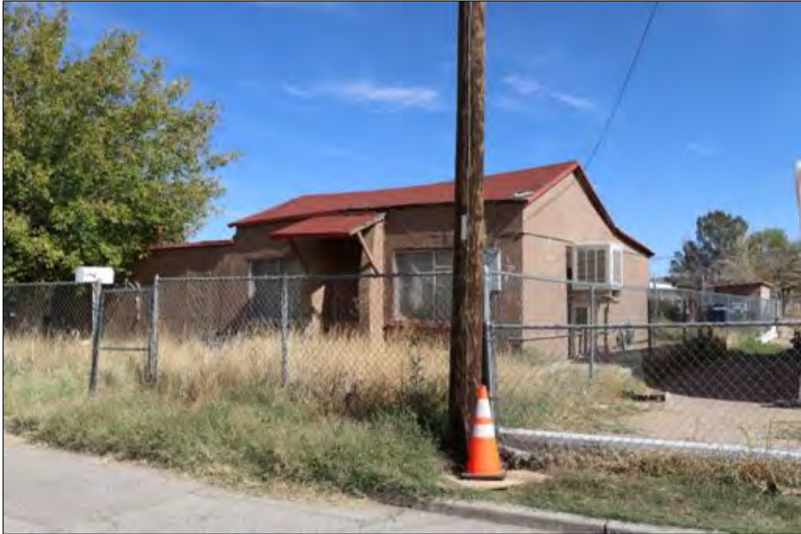
Figure 89. 208 Hardesty Place (Residence), looking northeast.
