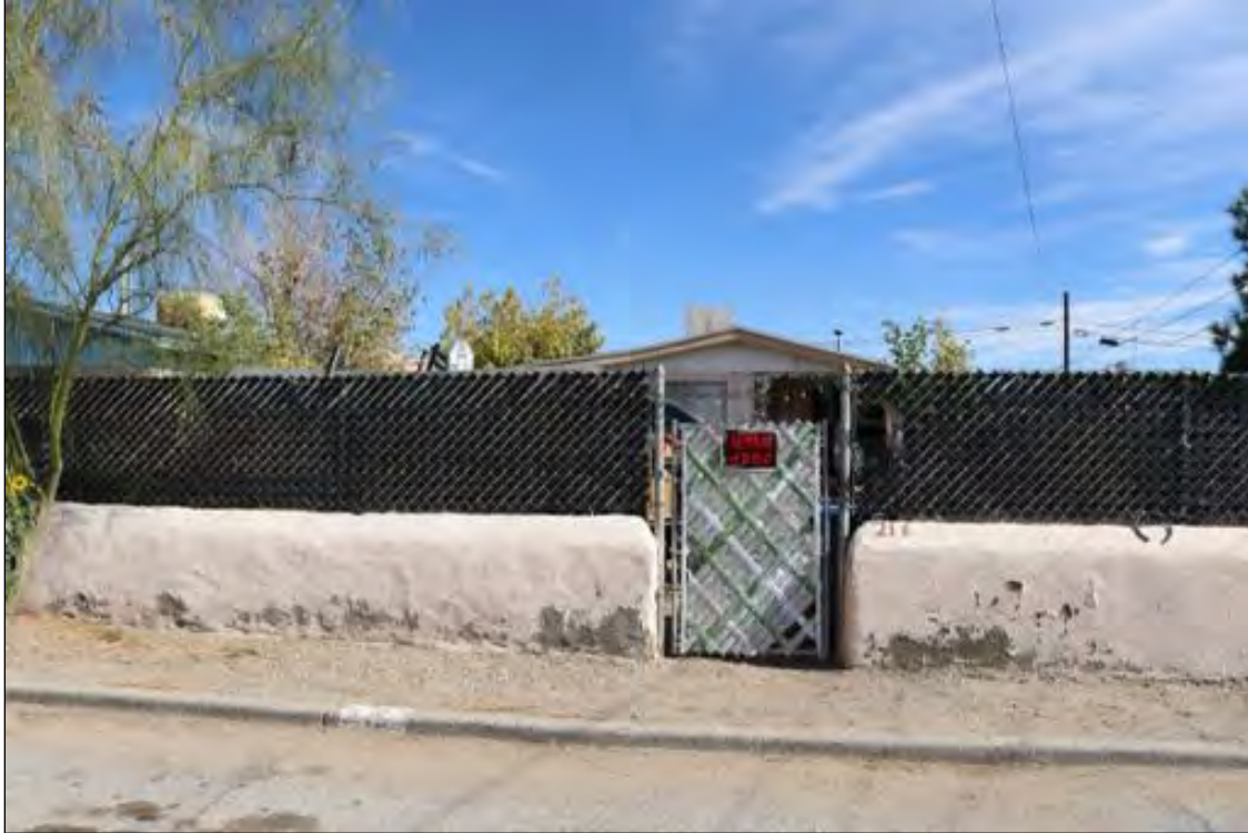
Figure 100. 216 Hardesty Place (Residence), looking east.
