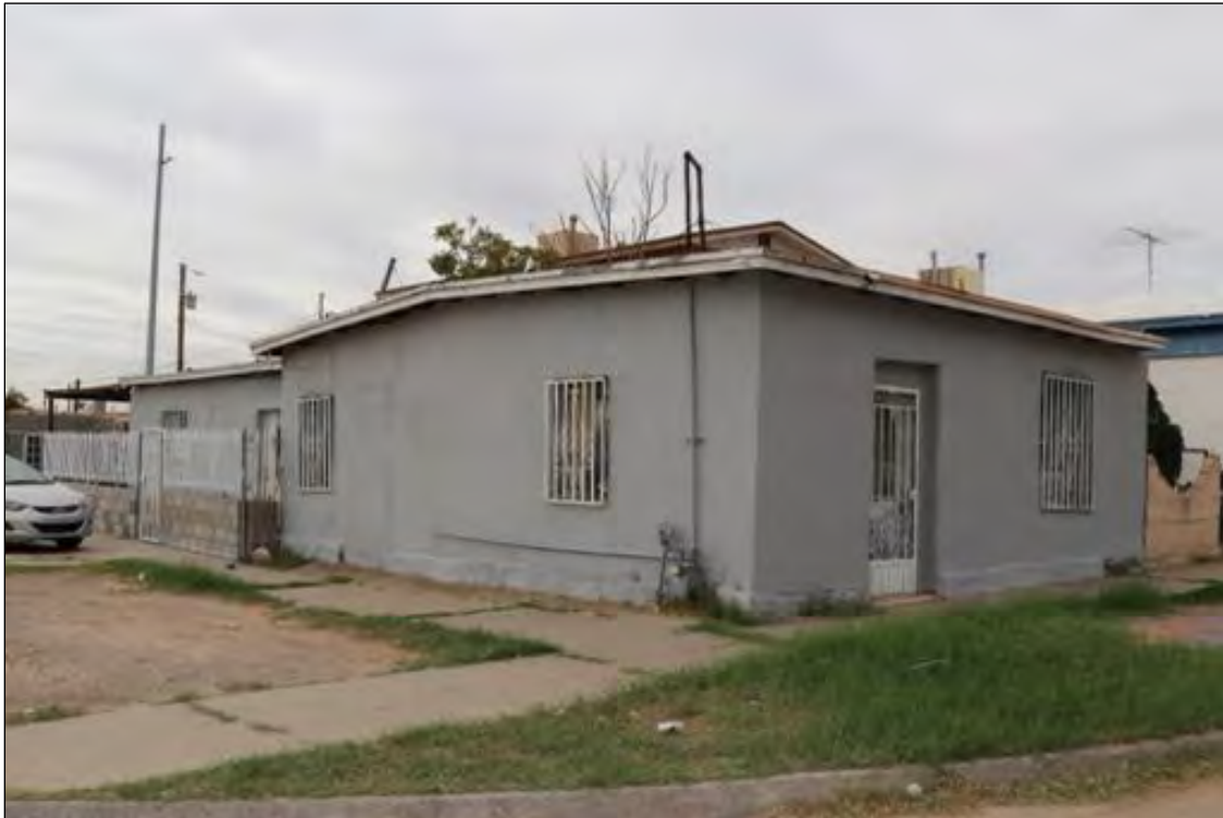
Figure 199. 3828 E San Antonio Avenue (Residence), looking southwest.
