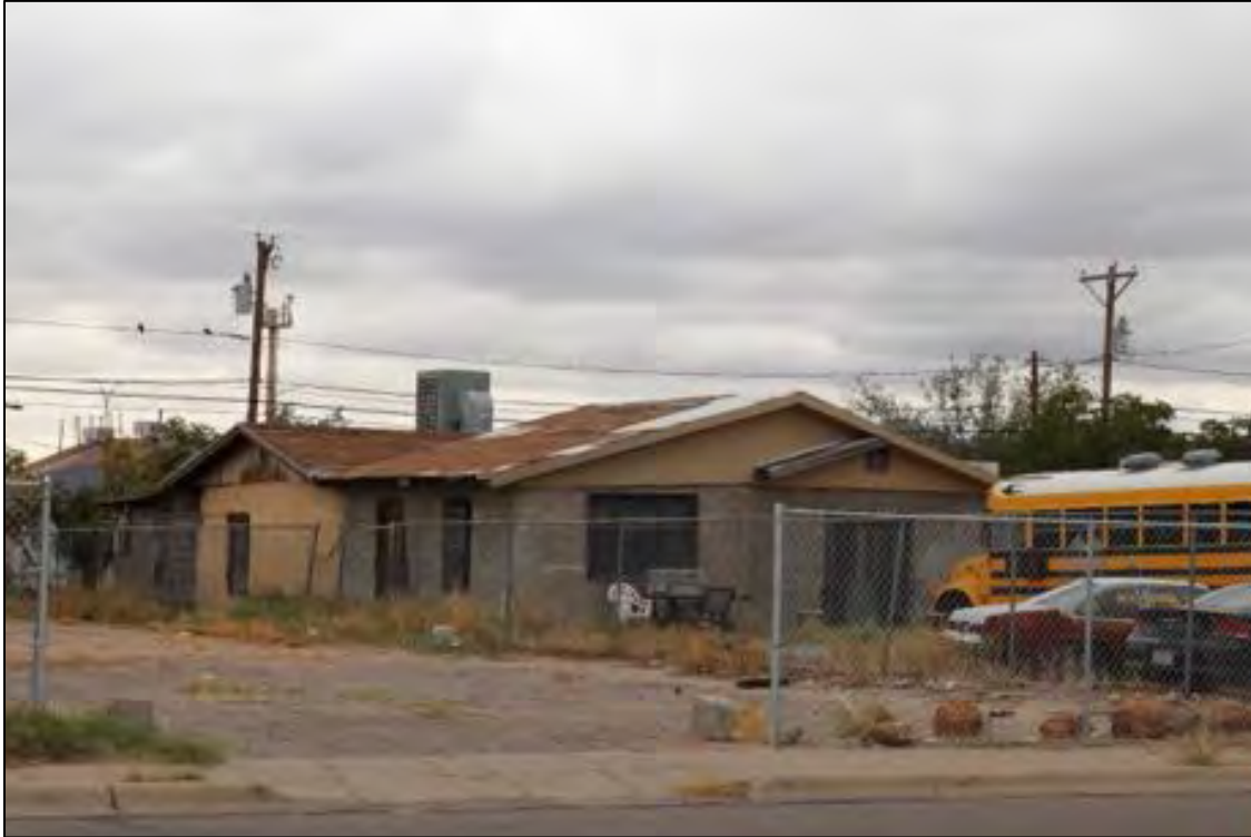
Figure 32. 4036 Delta Drive (Residence), looking south.
