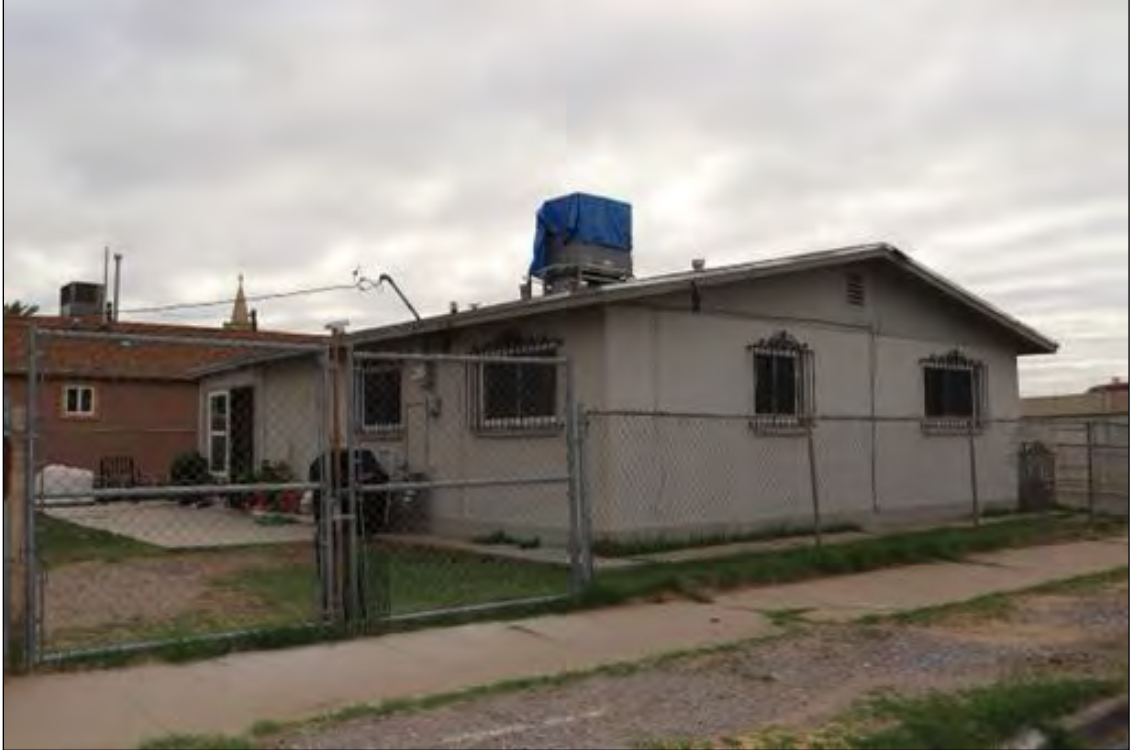
Figure 128. 3701 Findley Avenue (Residence) rear, looking southwest.
