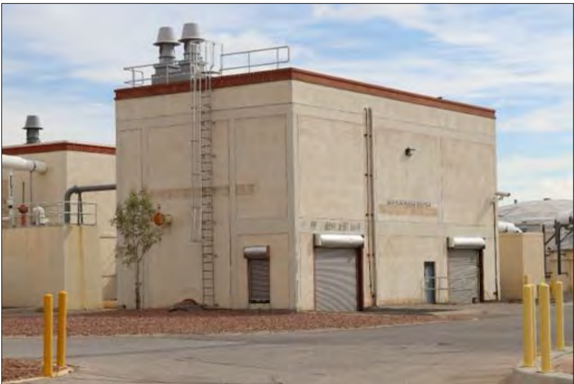
Figure 257. Grit Dewatering Building, looking southeast.
