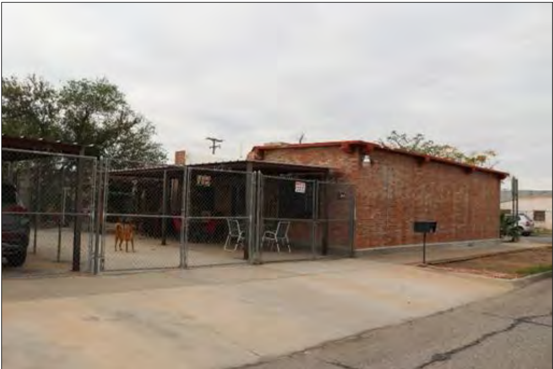
Figure 187. 3800 E San Antonio Avenue (Residence), looking southwest.
