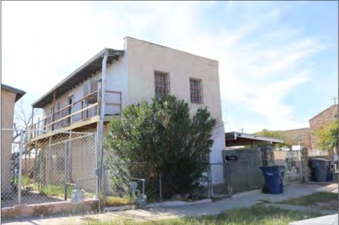
Figure 155. 3810 Findley Avenue (Residence), looking southwest.
