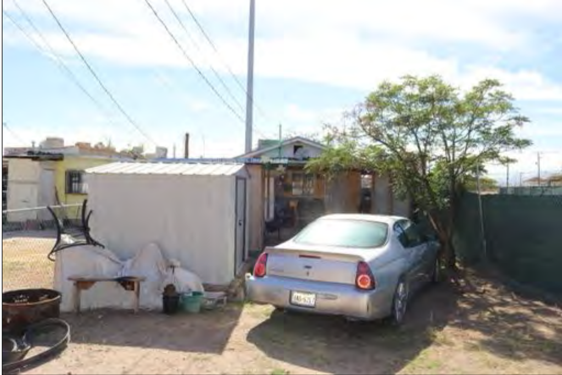
Figure 163. 3817 Findley Avenue (Residence) rear, looking south.
