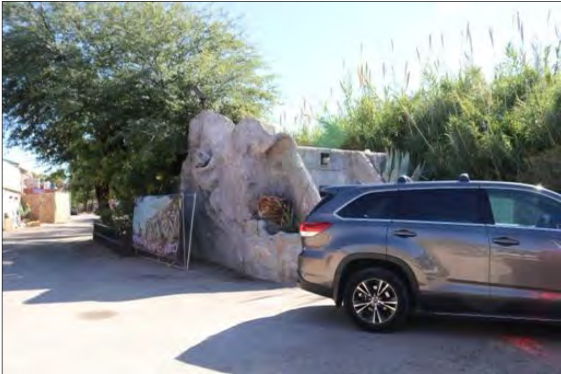
Figure 241. Holding, under construction, looking southeast.
