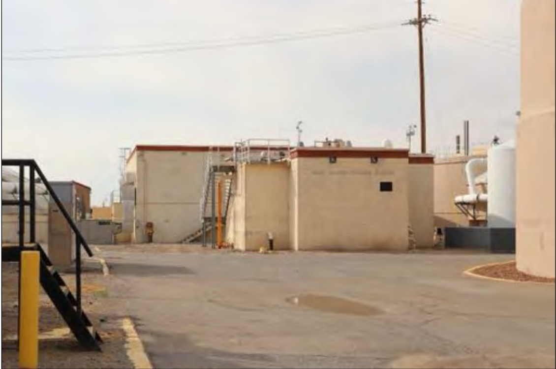
Figure 268. Mixed Sludge Pumping Station, looking west.
