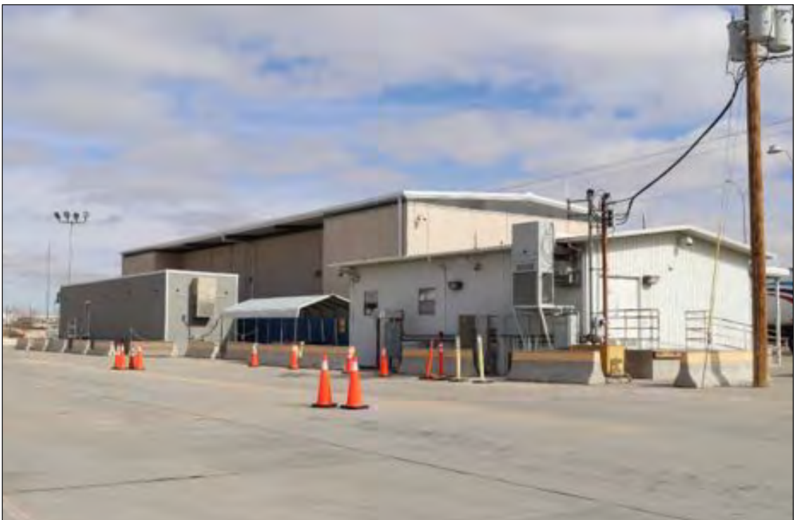
Figure 72. 3600 E Paisano Drive (Office Building for VACIS), note VACIS in background, looking northeast.
