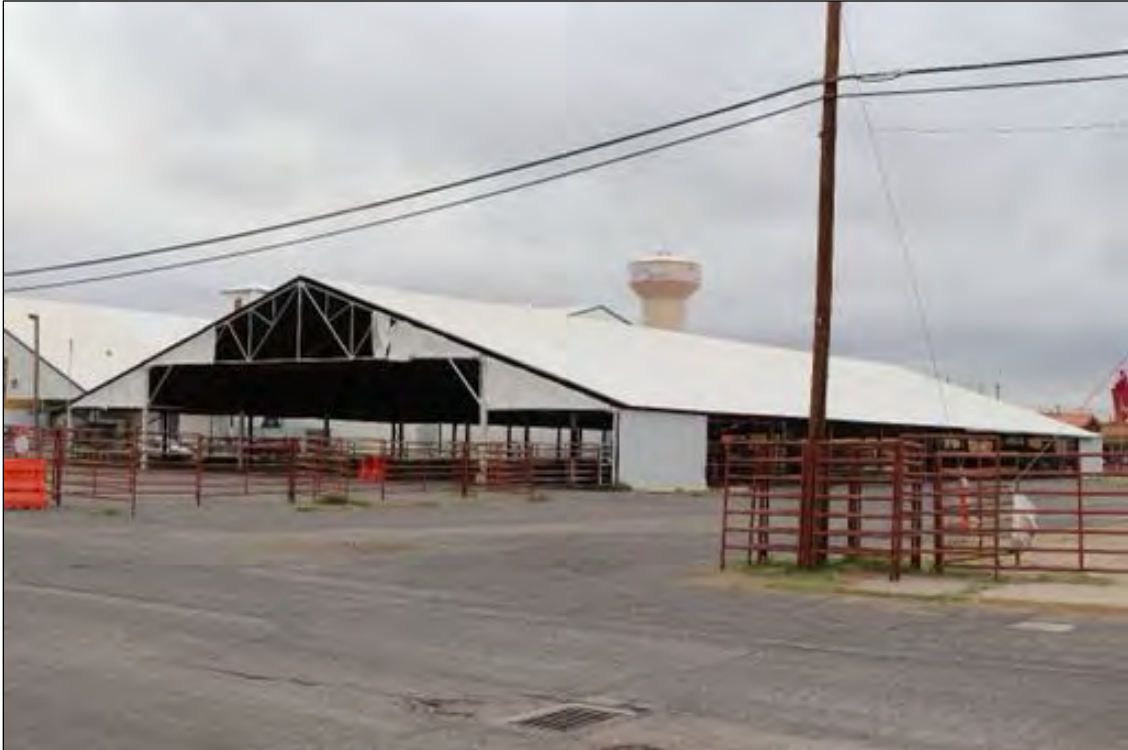
Figure 230. Event Center Shed Structure, looking southeast.
