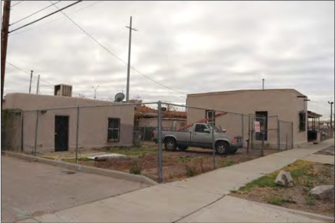
Figure 122. 420 S Latta (Residence) rear, looking southeast.
