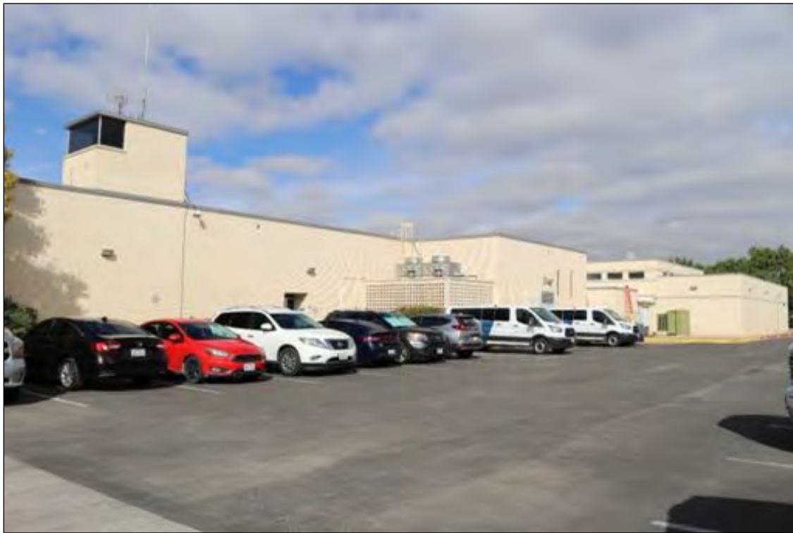
Figure 40. 3600 E Paisano Drive (Building A Administration Building), looking northwest.
