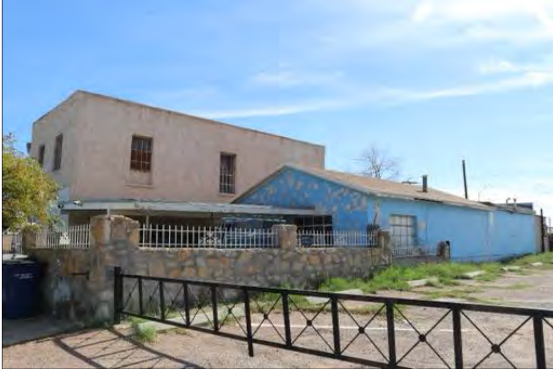
Figure 151. 3808 Findley Avenue (Residence), looking southeast.
