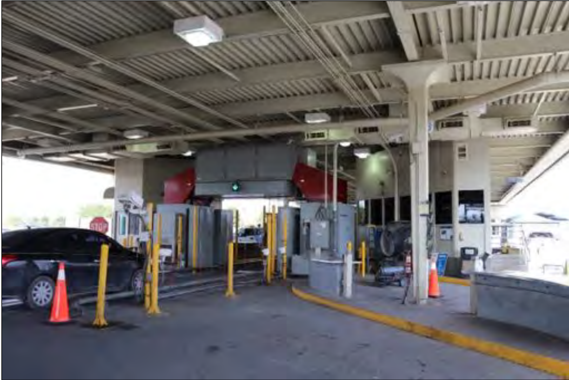
Figure 139. 3600 E Paisano Drive (Building K Primary/Secondary Inspection Canopy), Secondary Inspection Canopy.
