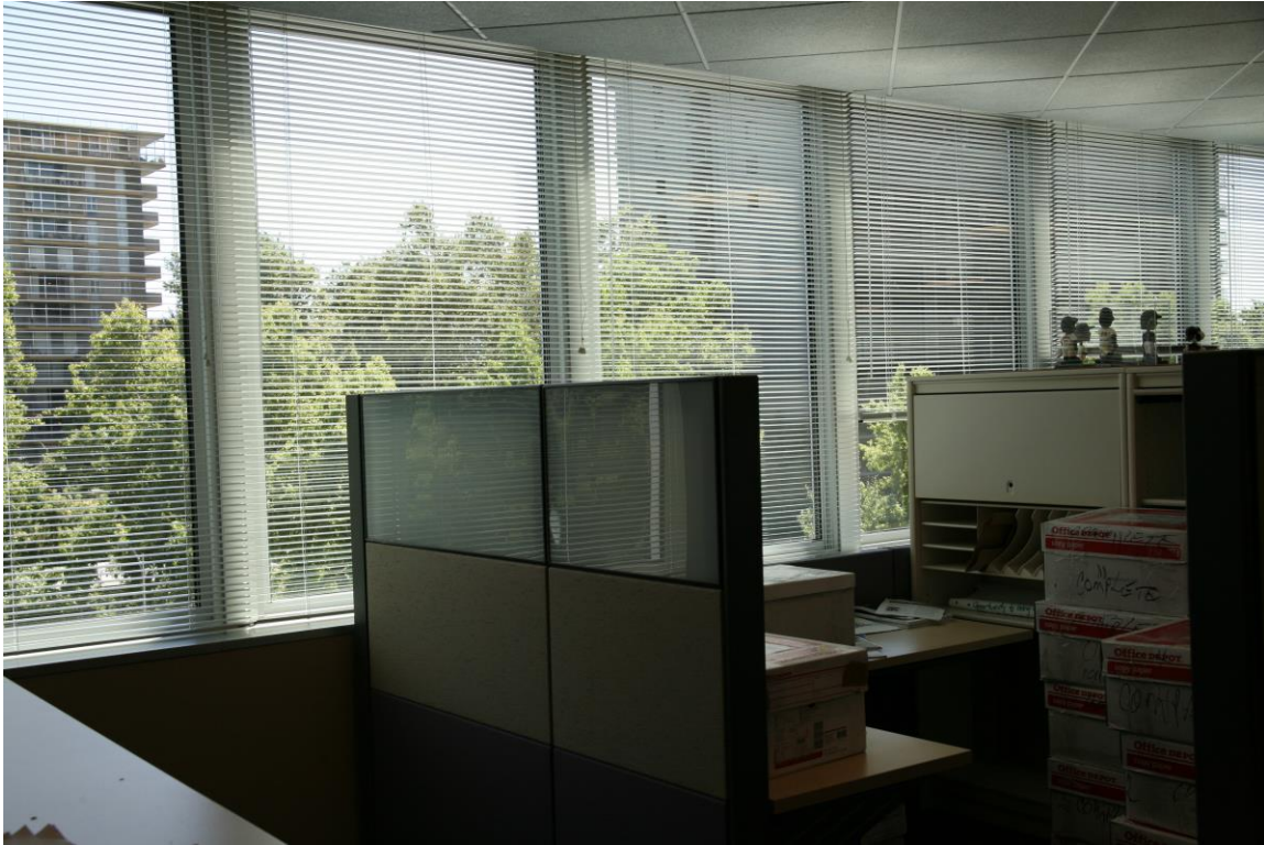
Figure IV-7. Original double-pane, low-emissivity, windows installed in the late 2000s.
