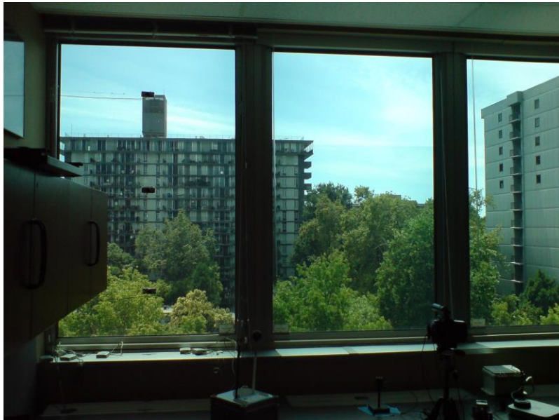
Figure IV-4. EC windows in daylight mode (zone 18 on June 14, 2016). All subpanes are controlled to the same tint.
