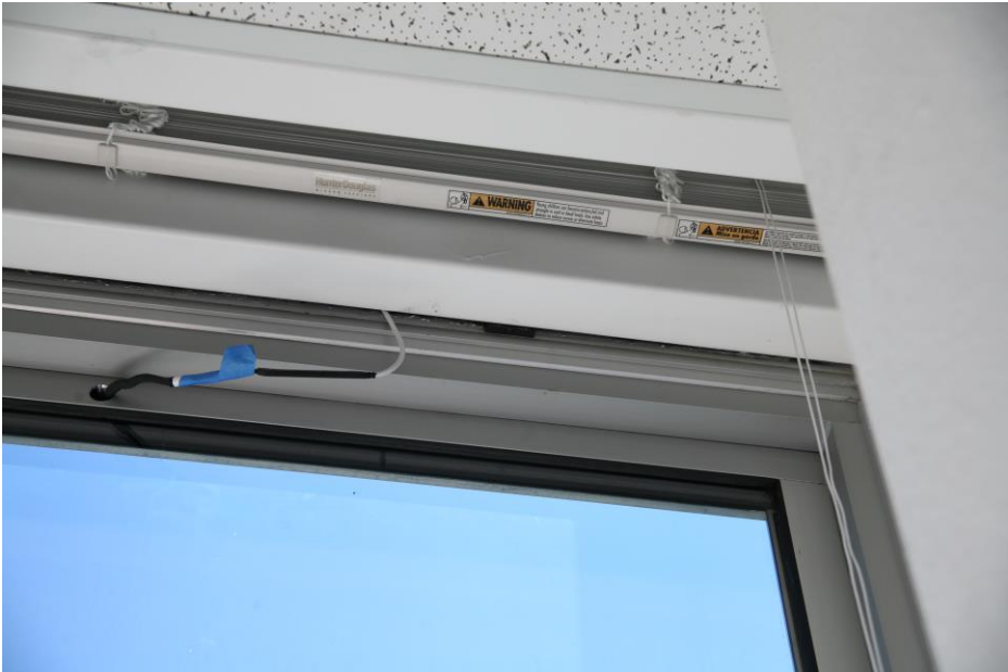
Figure IV-8. Frame with drilled hole allowing wire to exit window through the side of the frame.
