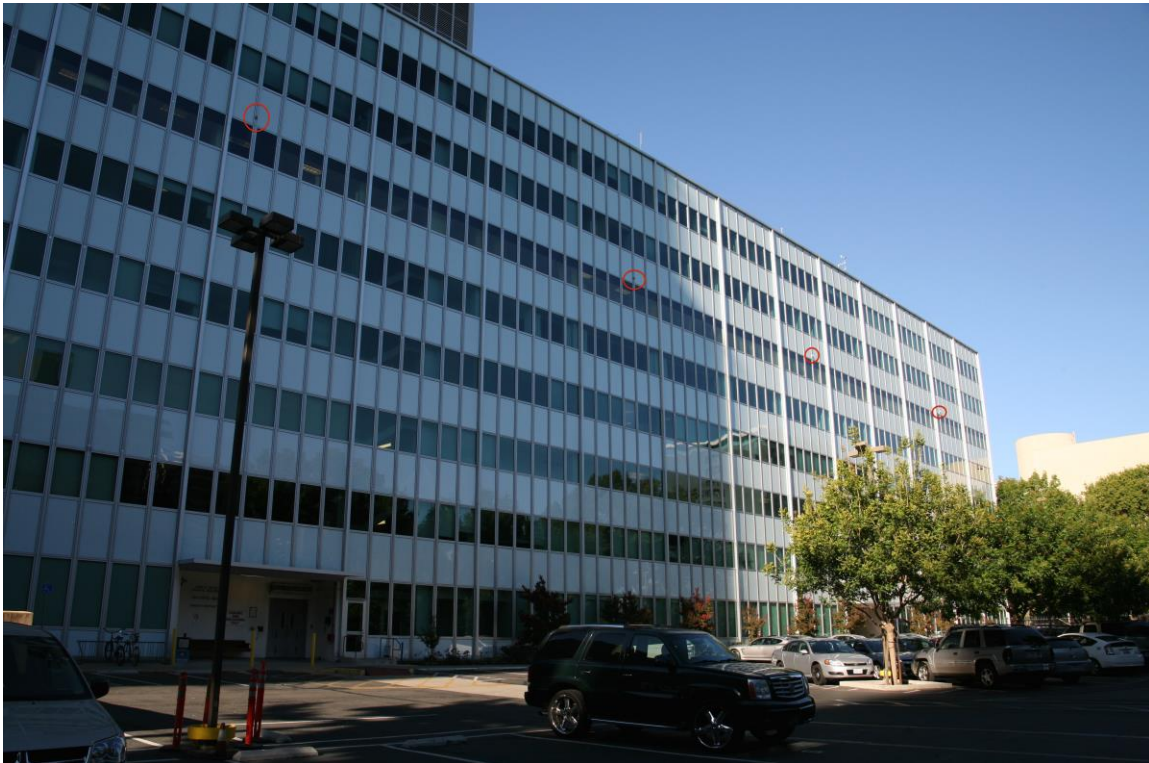
Figure IV-2. Location of sensors for electrochromic window control.
