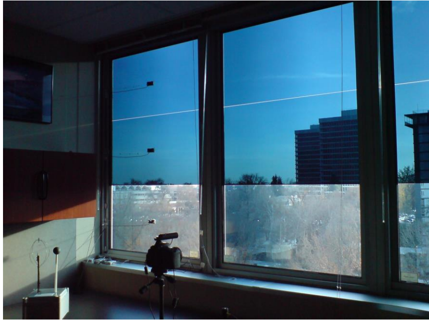
Figure IV-5. EC windows in glare mode (zone 18 on December 17, 2015). The top and middle subpanes are at full tint due to glare mode. The bottom pane is in daylight mode.
