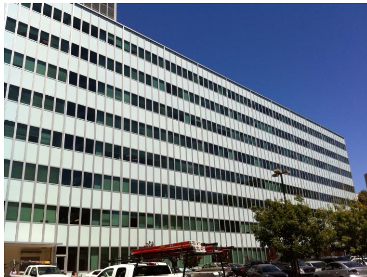
Figure III-1. Exterior of the South façade.
