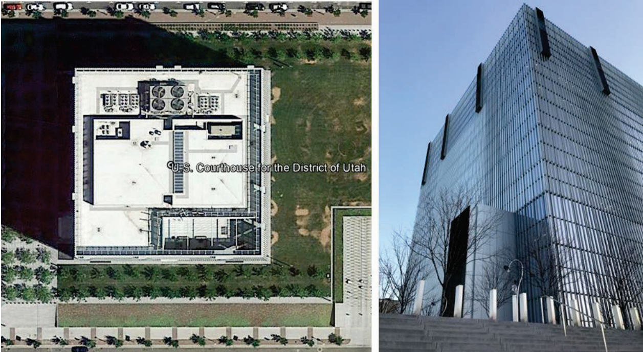
Figure 3: Salt Lake City courthouse. Sources: Google Earth (left); Jimmy Salasovich, NREL (right)
