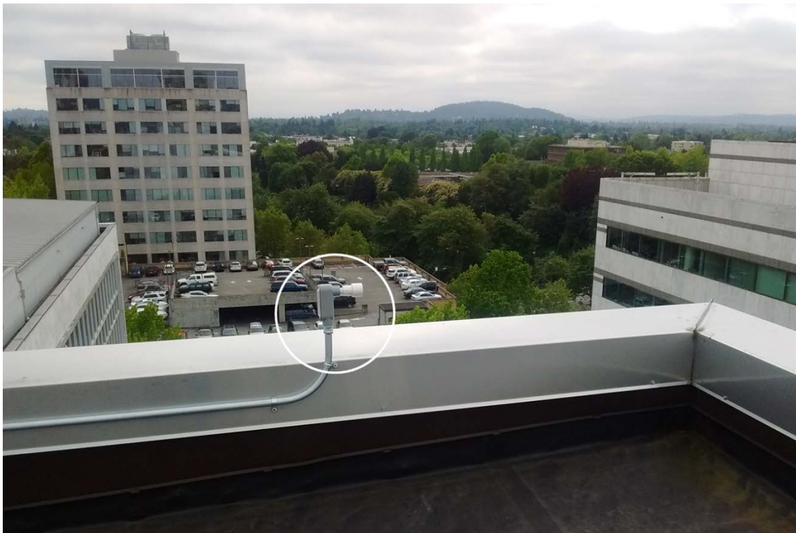
Figure IV.B.3. Rooftop sensor (circled).
