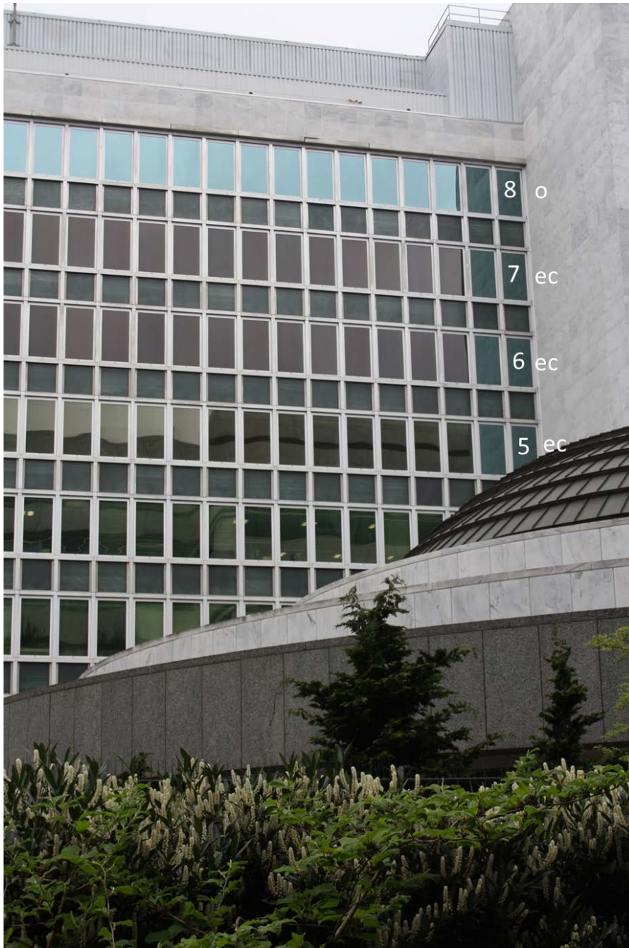
Figure V.A.14. Photograph of the west wing of the south façade on Saturday, April 9, 2016, at 8:30 AM. The Phase I EC windows on Floors 6–7 were operating in the Schedule mode and set to Tint 4. The Phase II EC windows on Floor 5 were operating in the automatic mode (Tints 1–3). Floor 8 shows the appearance of the original (“o”) existing reference low-e windows.
