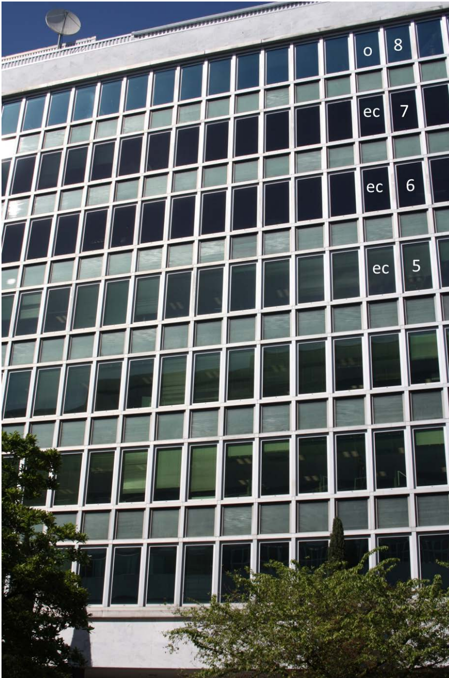
Figure V.A.13. Photograph of the east wing of the south façade on Friday, April 8, 2016, at 2:15 PM. The Phase I EC windows on Floors 6–7 were operating in automatic mode (Tints 1–3). Some windows may have been set manually to Tint 4. The Phase II EC windows on Floor 5 were set to Tint 1 (reference condition). Floor 8 shows the appearance of the original (“o”) existing reference low-e windows.
