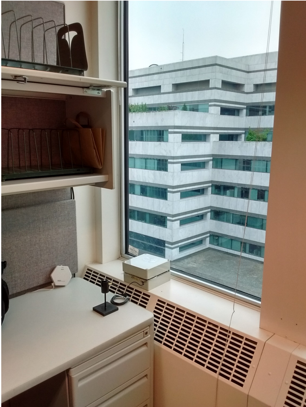
Figure C.4. Room with instrumentation level C. Image was taken prior to completion of installation.
