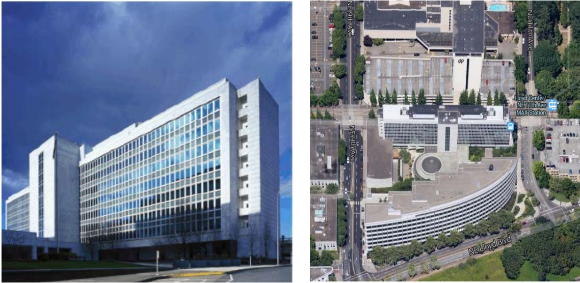
Figure IV.A.1. Exterior of the south façade (left) and site layout (right).
