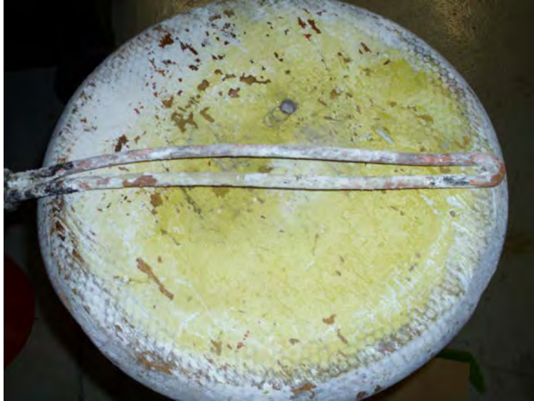
Figure 3. One of the Heating Elements Removed from the Electric Water Heater.
