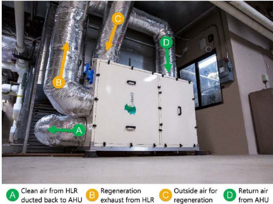
Figure 4. HLR installation in the ArcBest building
