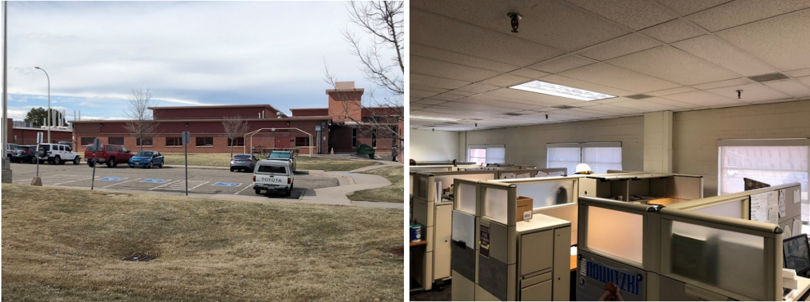
Figure 2: Building 53 - Exterior and Interior
