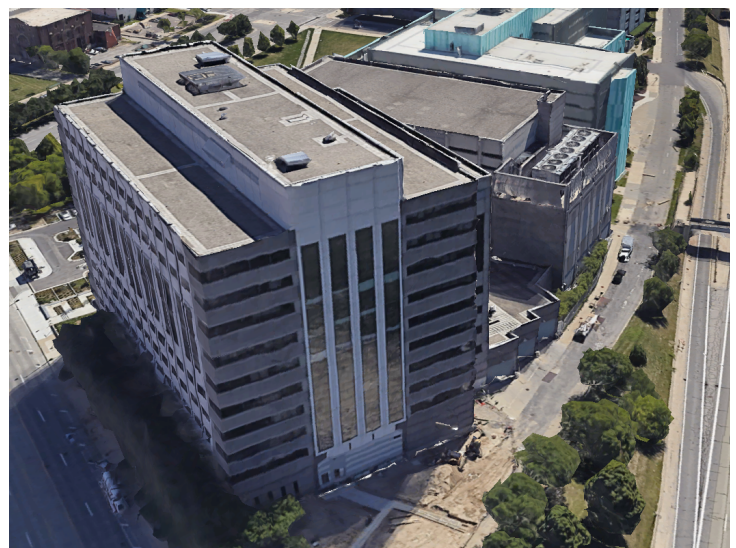
Aerial view of 985 Michigan showing the main building and parking garage. Cooling towers are adjacent to the parking garage.
