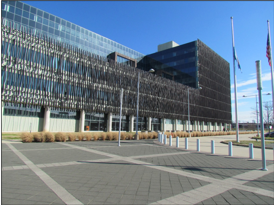
U.S. Census Bureau Building exterior, facing southeast (2020).
