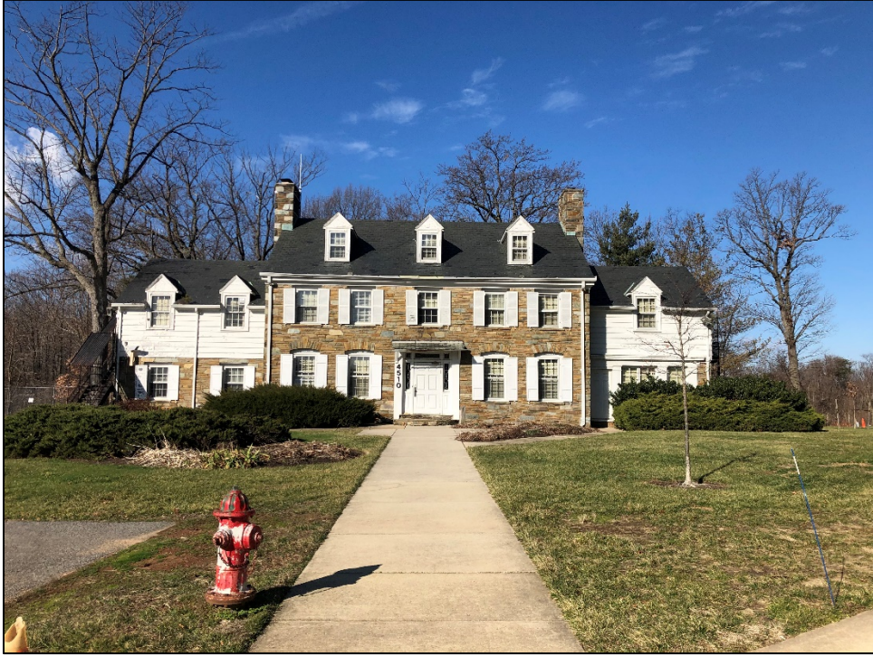
The Suitland House, southeast façade, facing northwest (2020).
