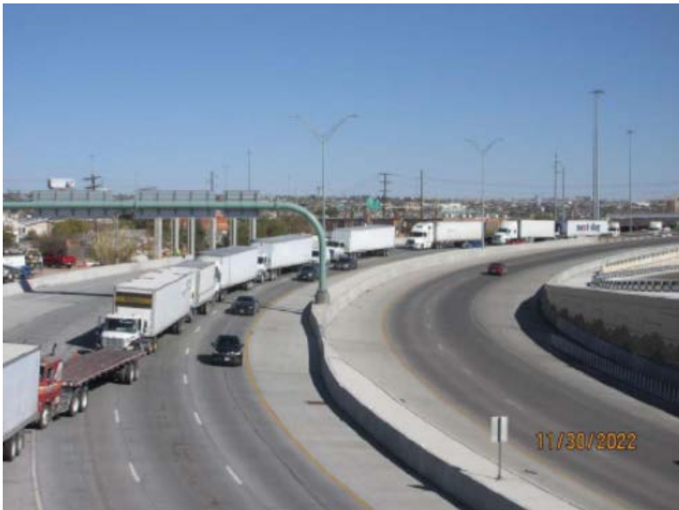
Photo of southbound traffic on I-110 next to Zavala Elementary/San Xavier, November 29, 2022, 2p MT
