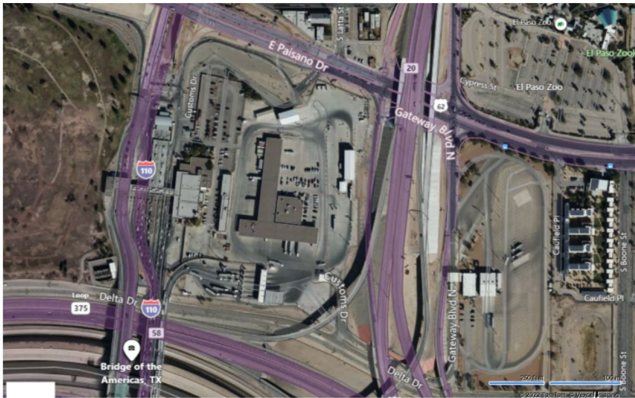
FIGURE 3. BRIDGE OF THE AMERICAS LPOE AERIAL MAP.
