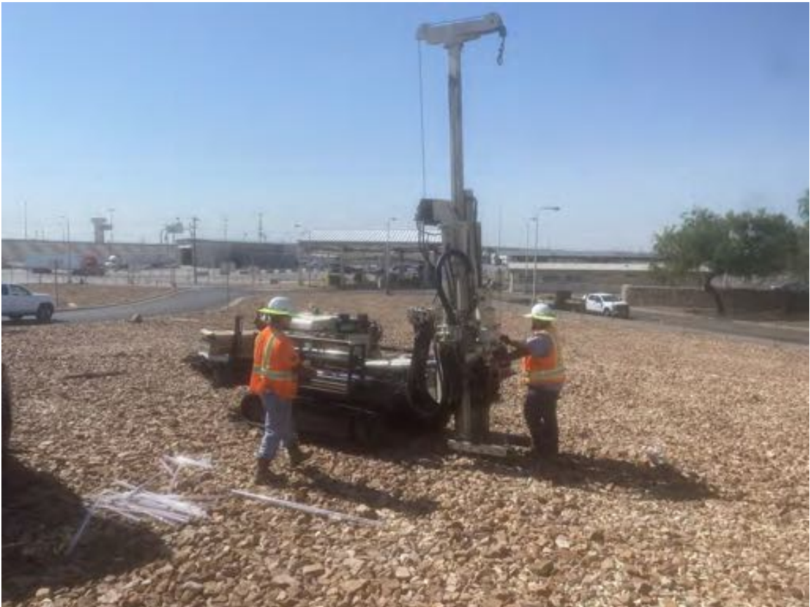
Photograph 2: View looking southeast of the drilling of soil boring SB-3.
