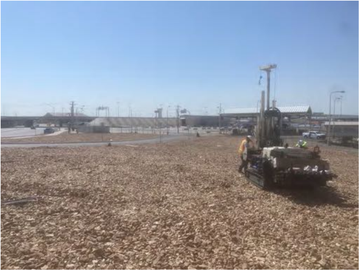
Photograph 3: View looking southeast of the drilling of soil boring SB-4.
