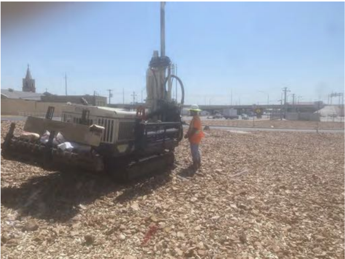
Photograph 4: View looking east of the drilling of soil boring SB-5.
