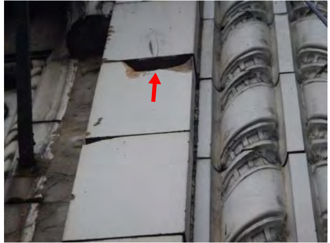
Photo 22: Remove loose+seal
