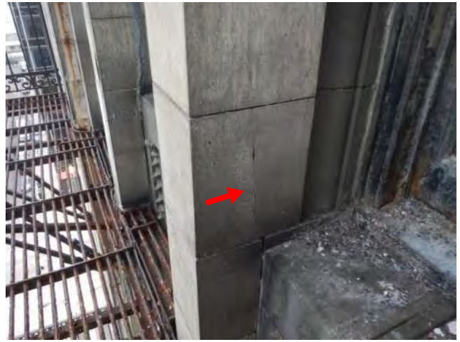
Photo 84: R/S cracks+ install straps
