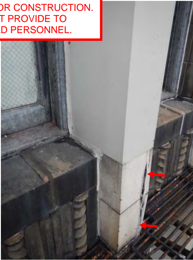
Photo 27: Remove loose + R/S cracks + install wood
