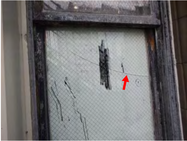
Photo 21: Cracked window
