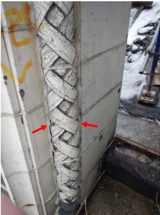
Photo 7: Seal joints
