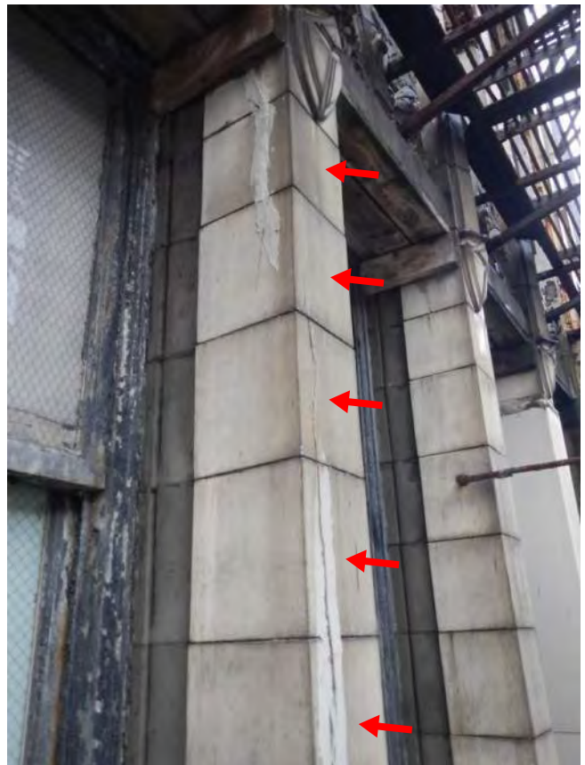
Photo 58: Remove loose + R/S cracks + install wood
