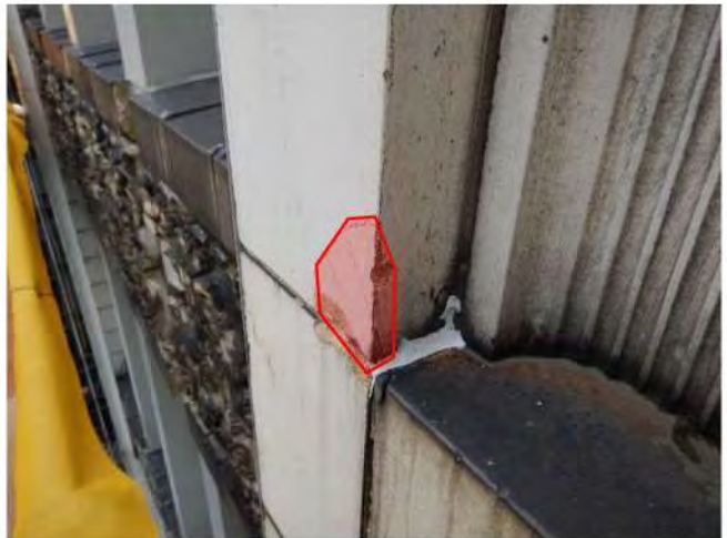
Photo 86: Remove loose
