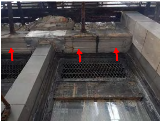
Photo 145: Install mesh or strap
