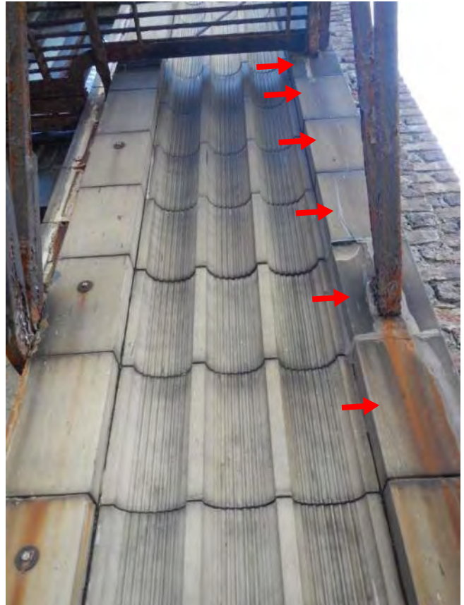
Photo 70: R/S cracks + install straps
