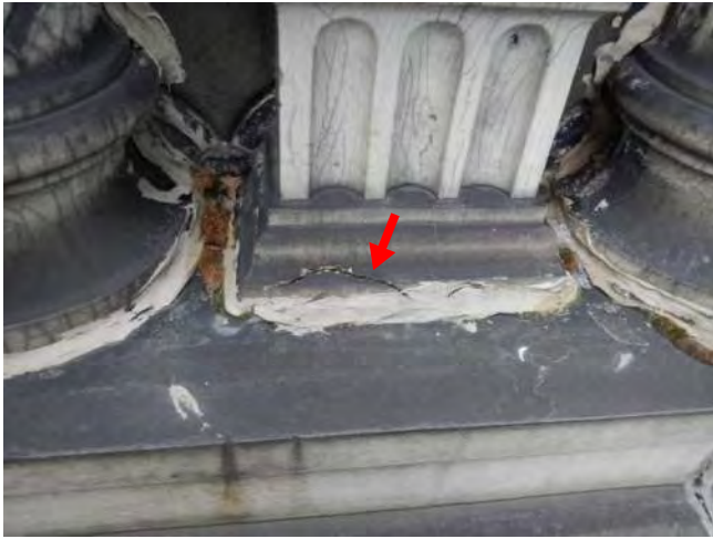
Photo 1: Remove loose + seal
