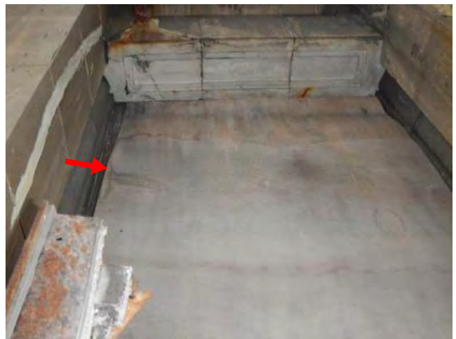
Photo 146: Remove loose panel
