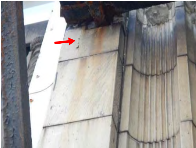
Photo 27: Remove loose + R/S cracks + install wood
