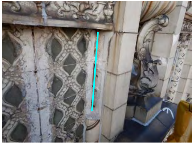
Photo 2: Fill holes with mortar
