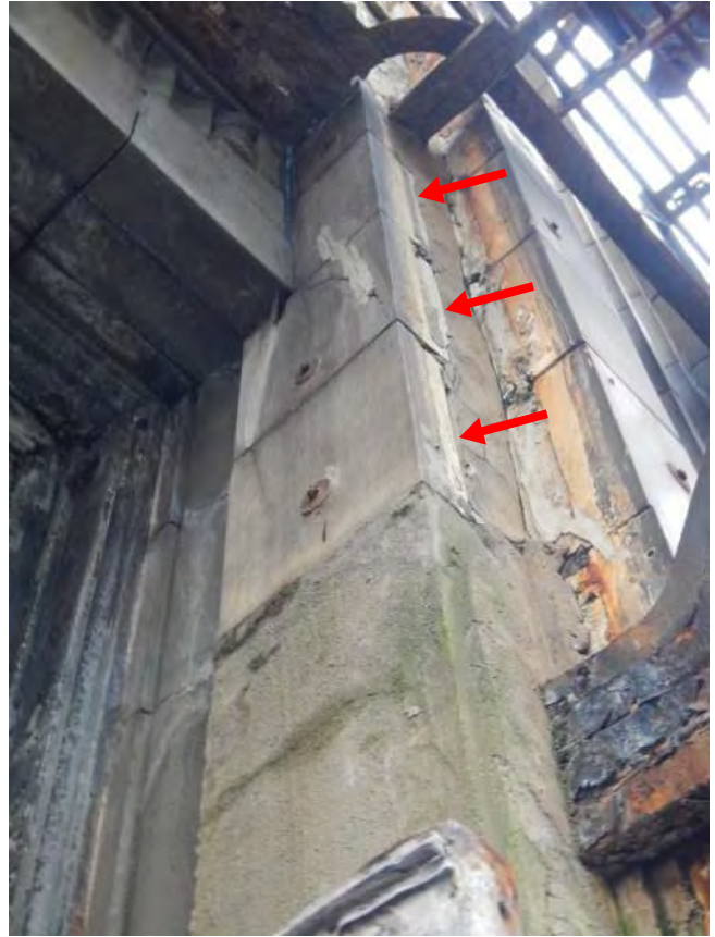
Photo 80: R/S cracks + install straps
