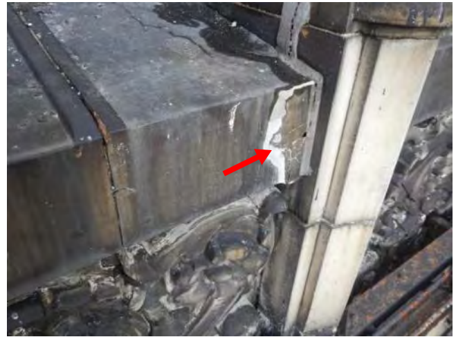
Photo 32: R/S cracks+ install straps
