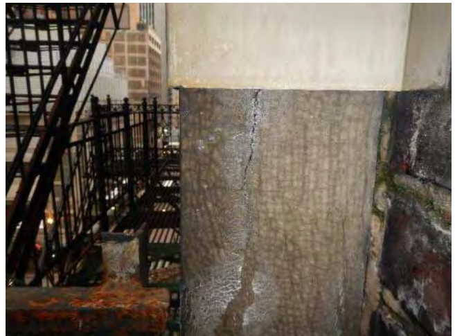
Photo 10: R/S at terra cotta
