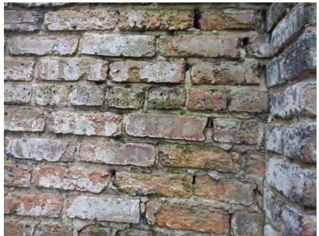
Photo 6: Miscellaneous brick replacement full story height
