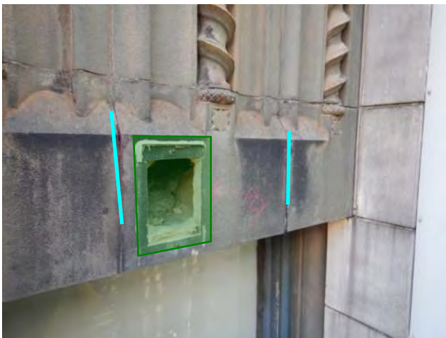
Photo 87: Install wood + TP
