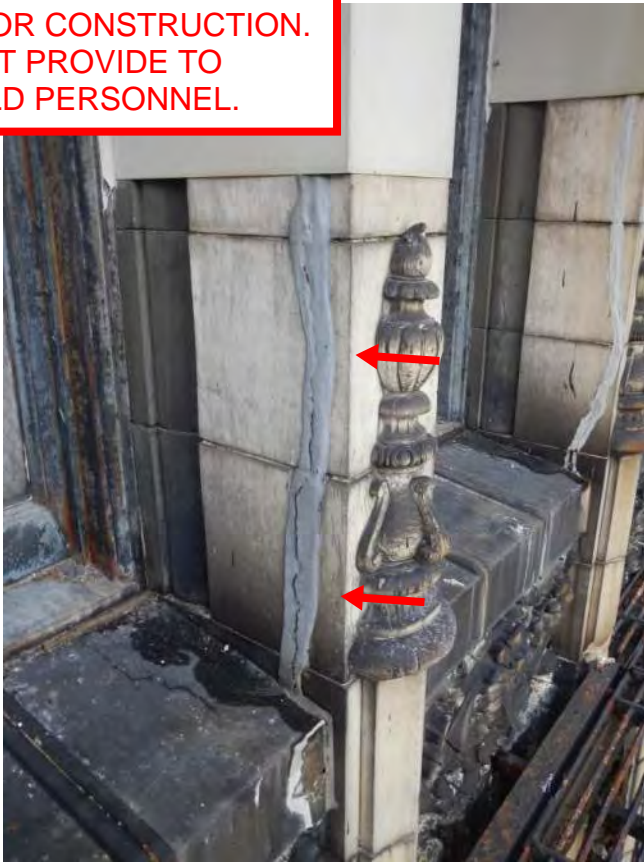
Photo 35: R/S cracks+ install straps
