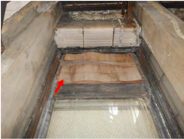
Photo 143: Remove loose panel
