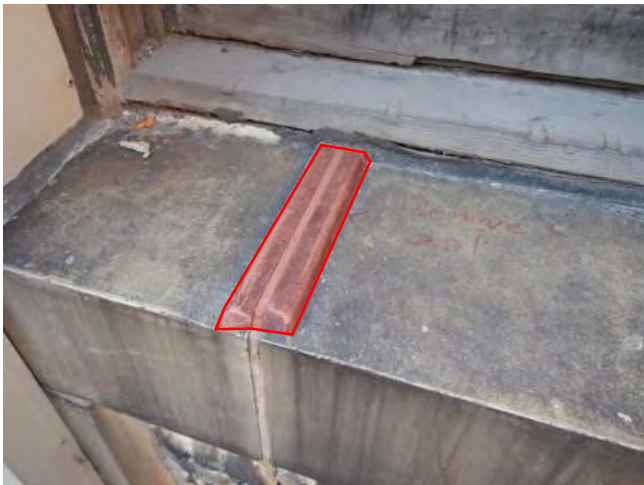
Photo 125: Remove spall
