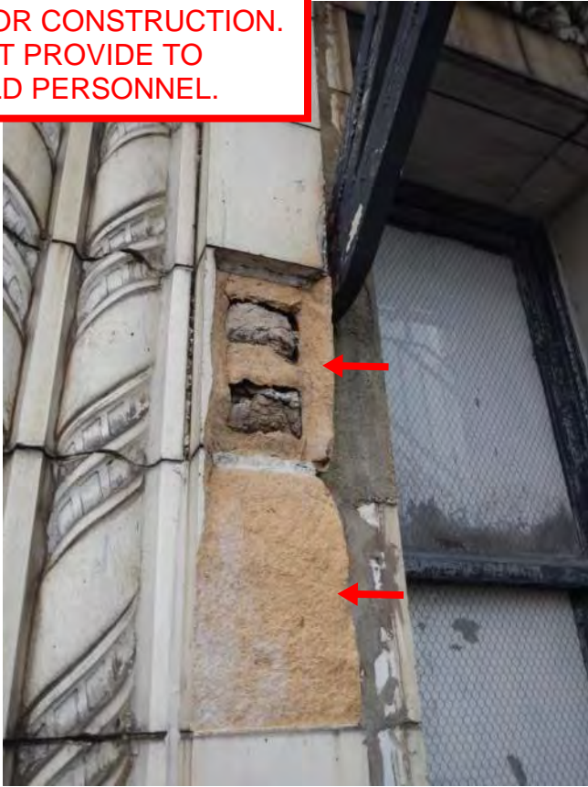
Photo 15: Remove loose + seal & R/S
