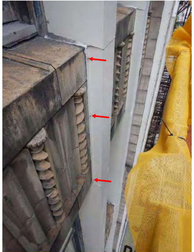
Photo 36: Replace (3) fasteners
