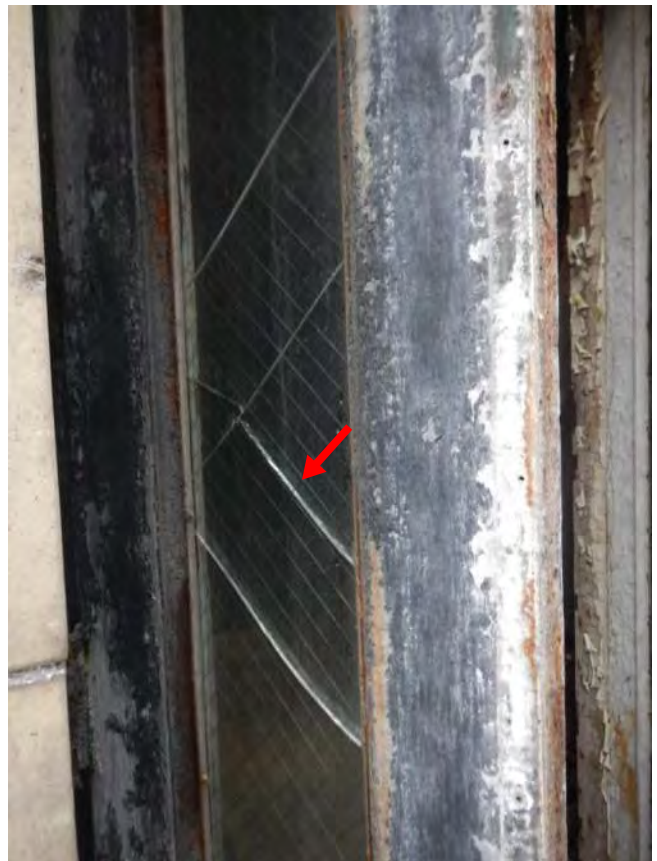
Photo 100: Cracked window
