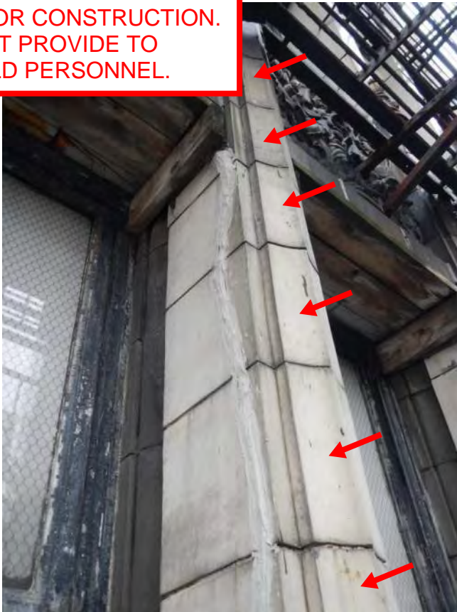
Photo 47: Remove loose + R/S cracks + install wood
