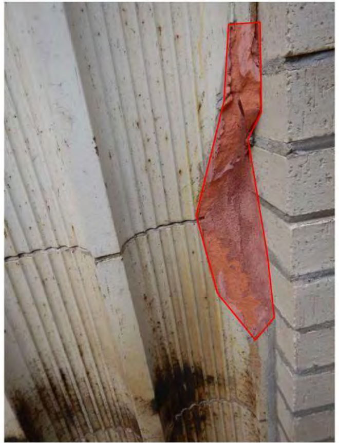
Photo 46: Grind, clean, seal
