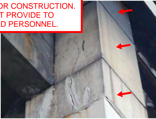
Photo 31: R/S cracks + install straps
