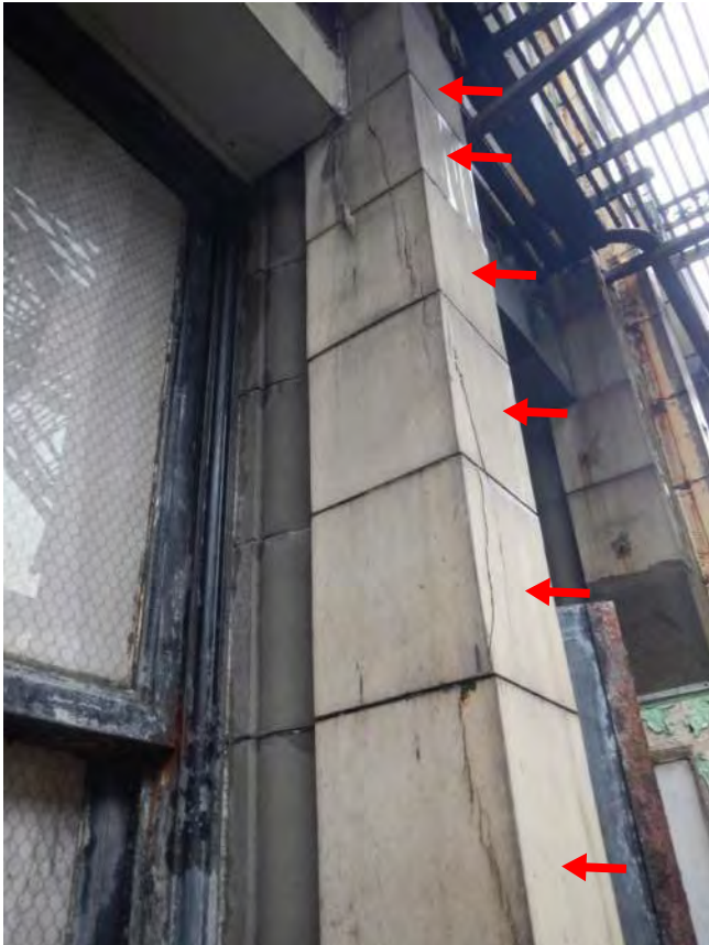
Photo 65: Remove loose + R/S cracks + install wood
