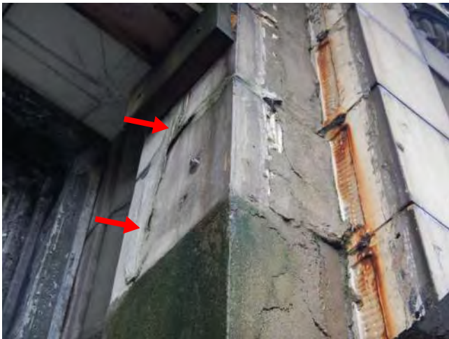
Photo 47: Remove loose + R/S cracks + install wood
