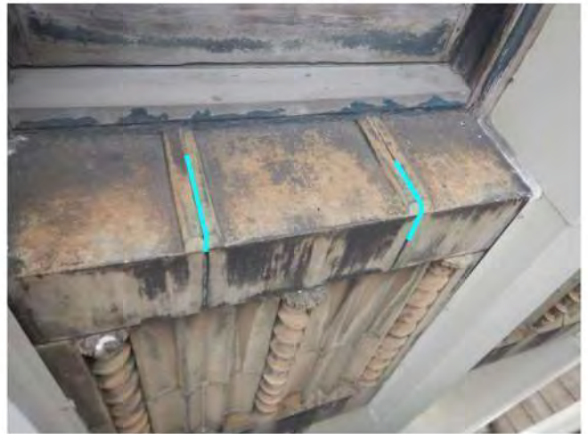
Photo 46: Grind, clean, seal
