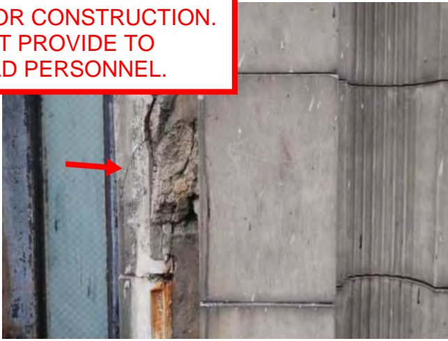
Photo 141: R/S crack + install strap
