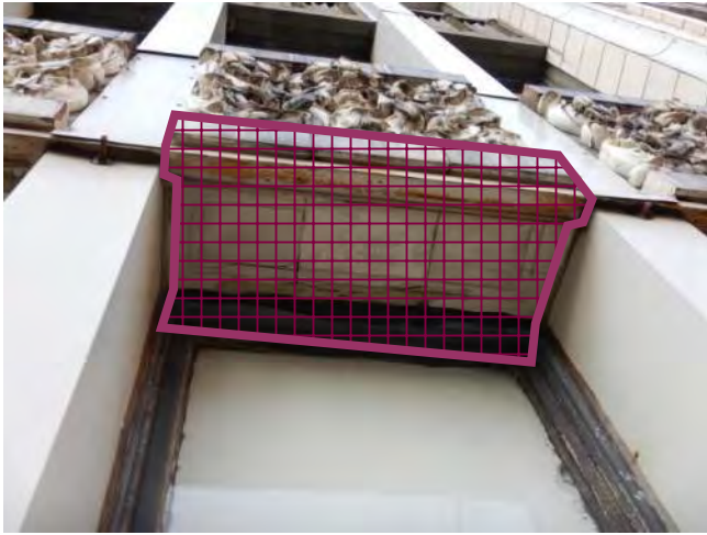
Photo 3: Install mesh
