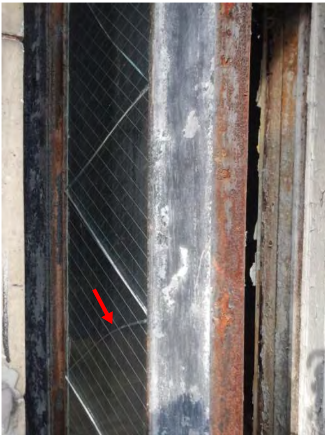
Photo 95: Cracked window
