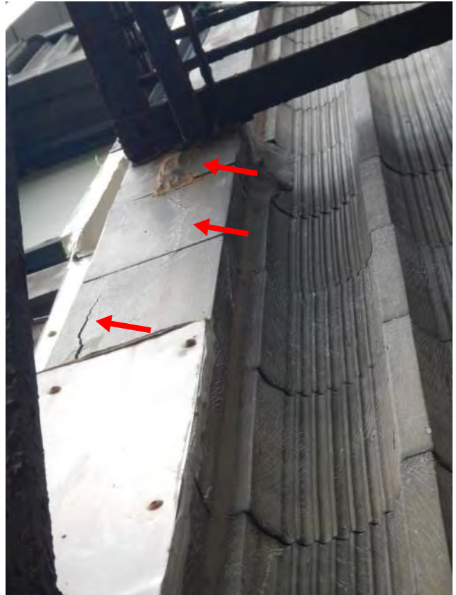
Photo 86: R/S cracks+ install straps
