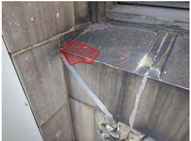
Photo 10: Remove loose
