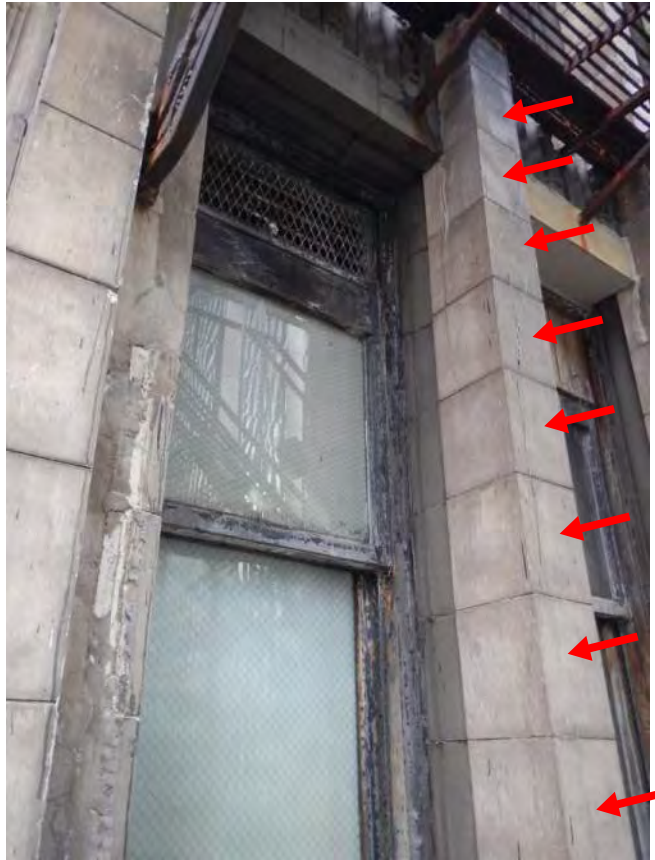
Photo 132: R/S cracks + install straps
