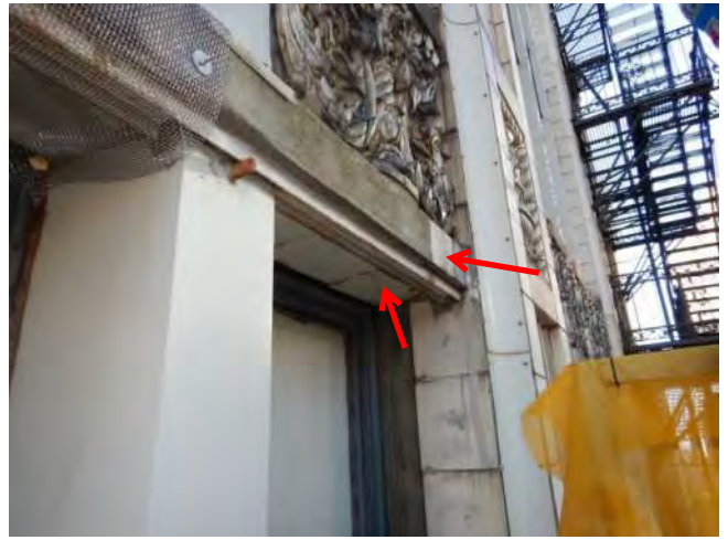
Photo 24: Remove header, clean & paint steel, + install plywood
