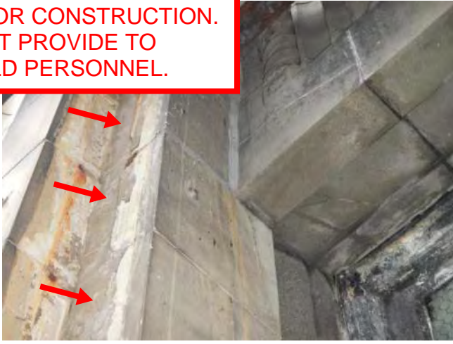
Photo 59: Remove loose + seal
