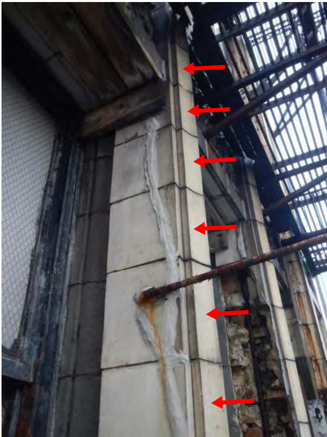
Photo 45: Remove loose + R/S cracks + install wood
