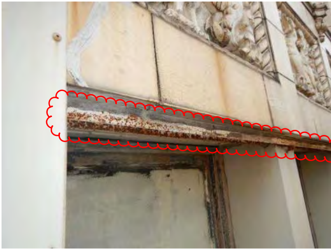
Photo 93: Clean & paint steel channels
