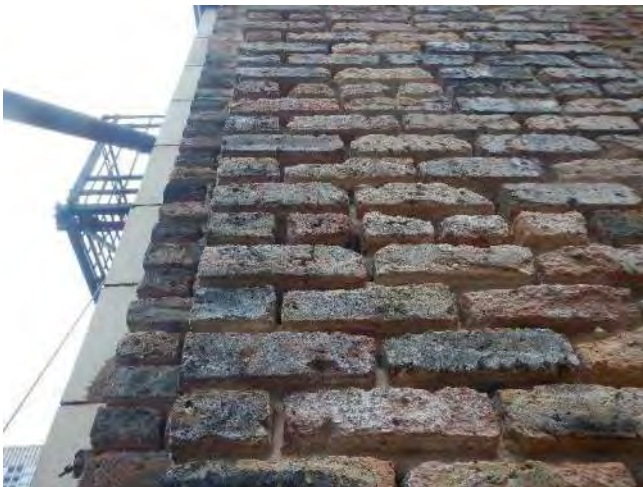
Photo 5: TP mortar joints
