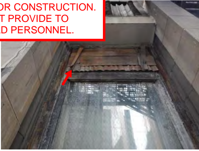
Photo 133: Remove loose panel
