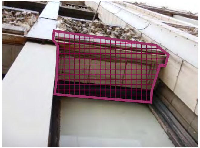
Photo 4: Install mesh
