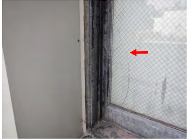
Photo 20: Cracked window
