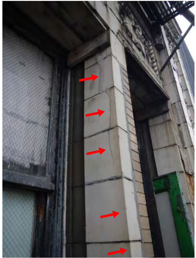
Photo 28: Remove loose + R/S cracks + install wood
