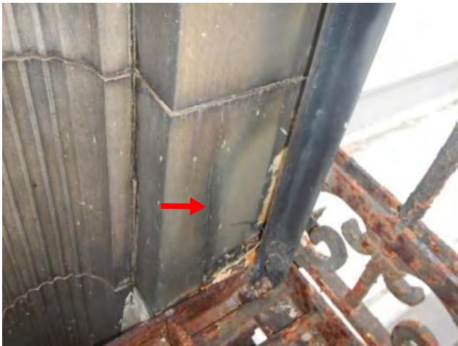
Photo 121: R/S cracks+ install straps
