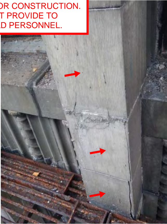
Photo 121: R/S cracks+ install straps
