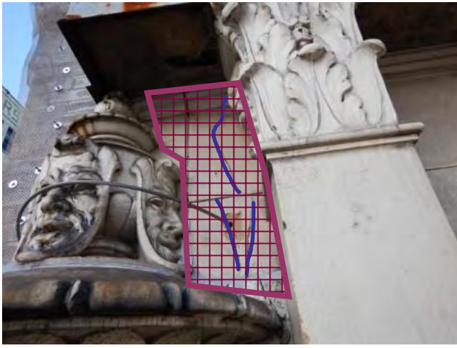
Photo 1: R/S & Install mesh
