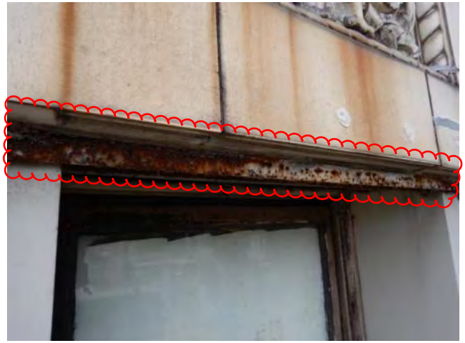
Photo 2: Clean & paint steel channels
