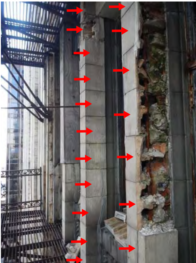
Photo 73: Remove loose + R/S cracks + install wood
