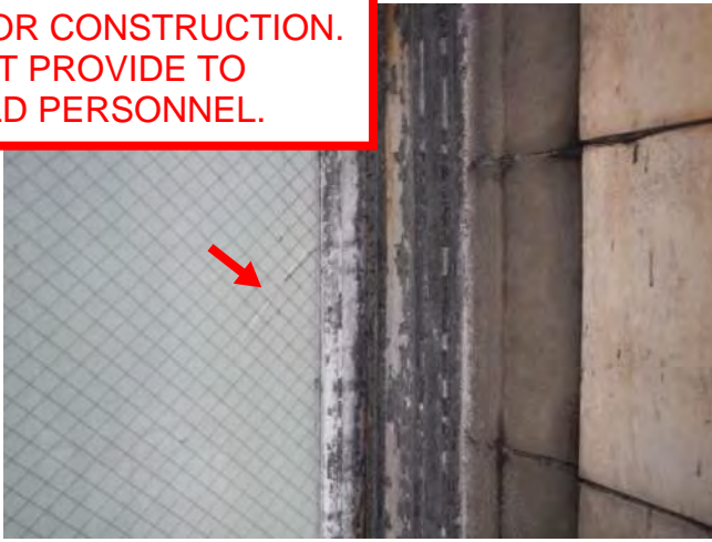
Photo 83: Cracked window
