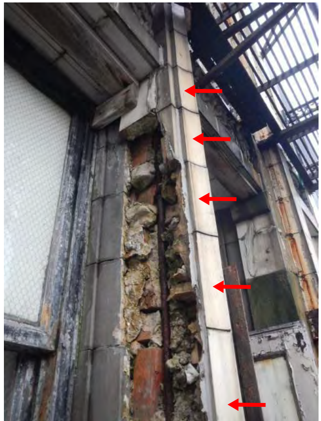
Photo 50: Remove loose + R/S cracks + install wood
