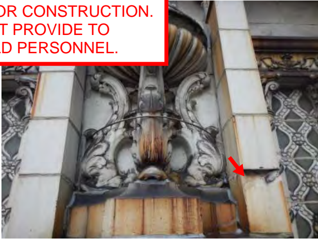
Photo 1: Remove loose + seal
