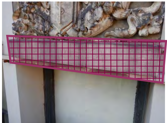
Photo 38: Install mesh
