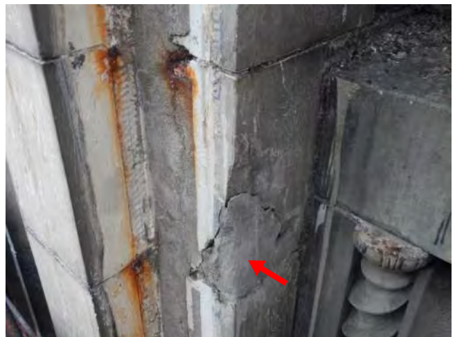
Photo 92: Remove loose
