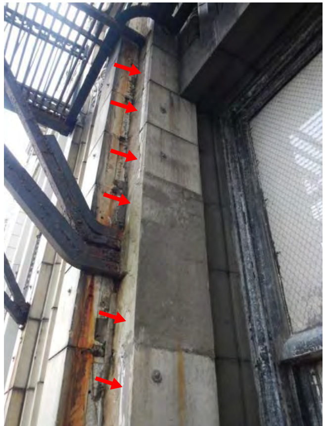
Photo 30: Remove loose patch material + replace
