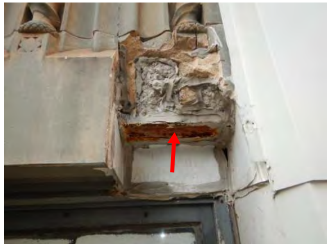
Photo 6: Seal terracotta, clean & paint steel
