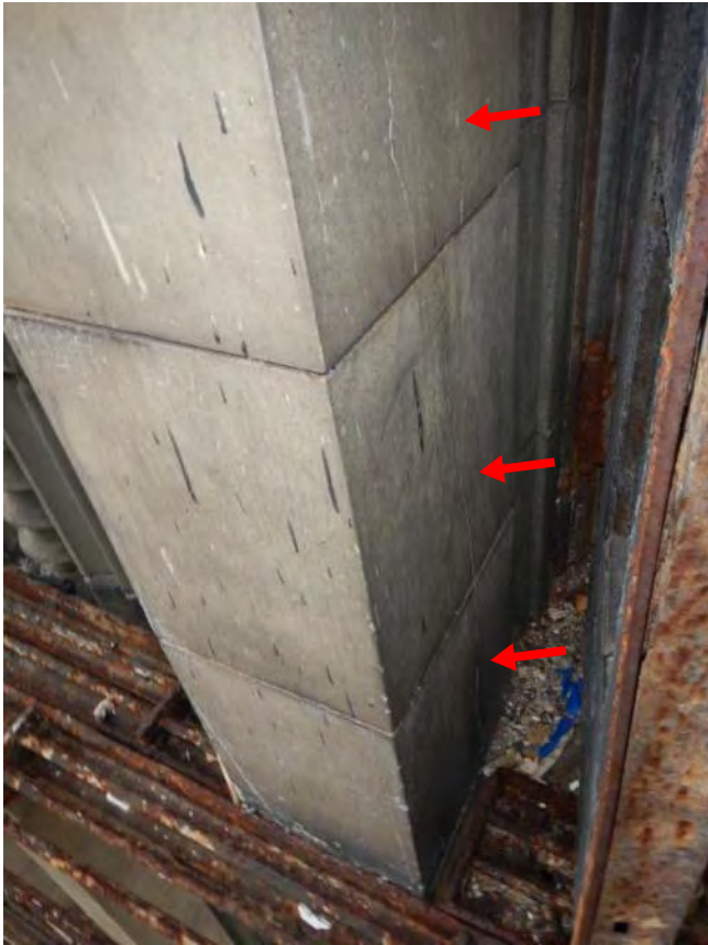
Photo 135: R/S cracks + install straps
