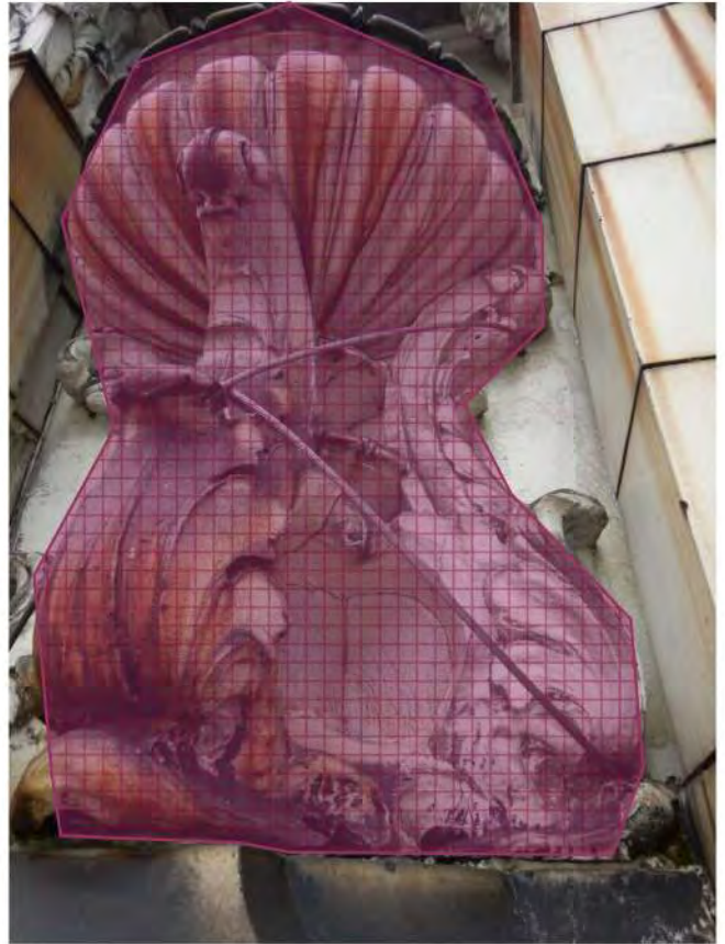
Photo 102: Install mesh over urn
