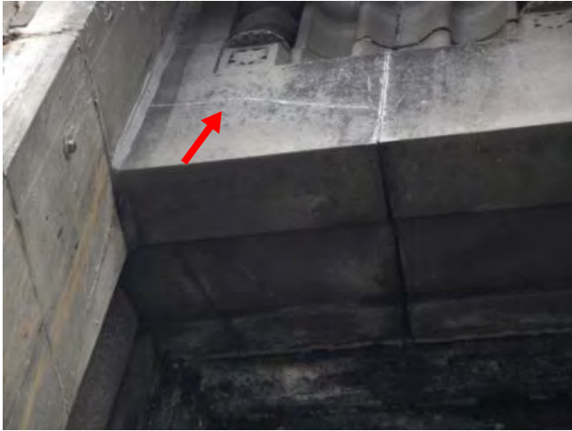
Photo 59: Remove loose + seal
