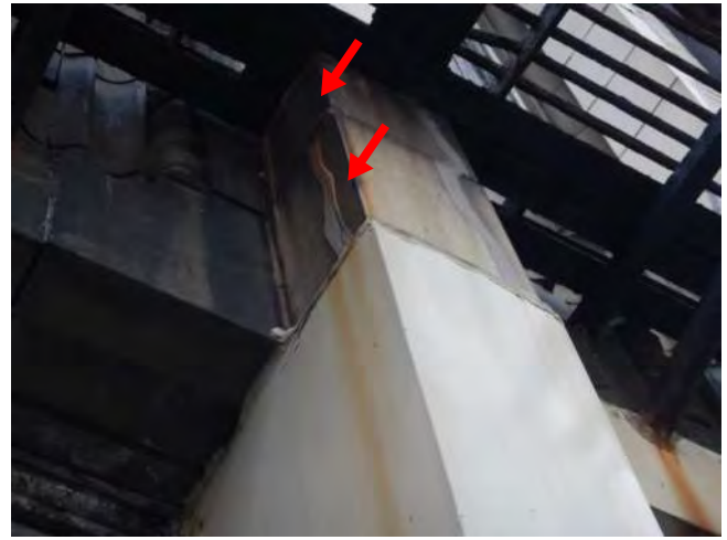
Photo 32: R/S cracks+ install straps
