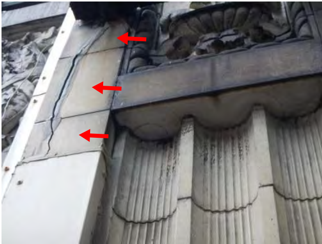
Photo 53: R/S cracks + install straps
