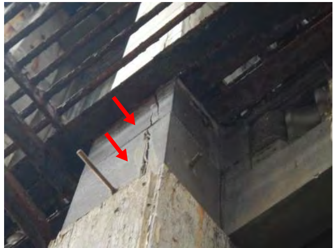
Photo 150: Remove loose + install wood
