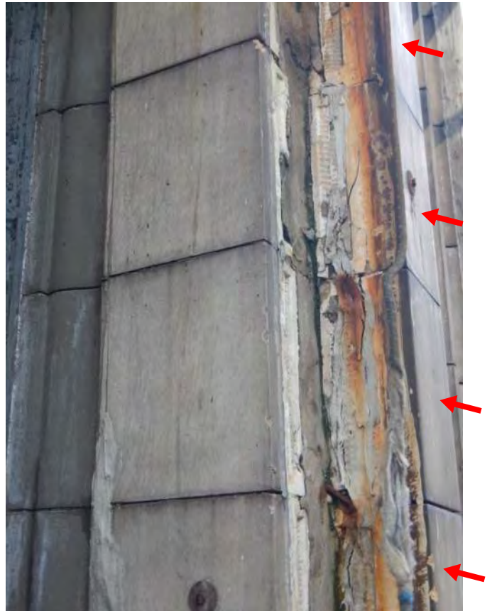
Photo 106: R/S cracks + install straps
