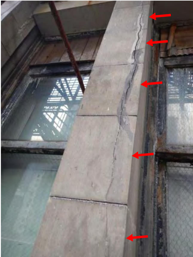
Photo 131: R/S cracks + install straps
