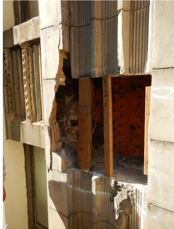
Photo 38. Exploratory opening at 7th floor column, east elevation.
