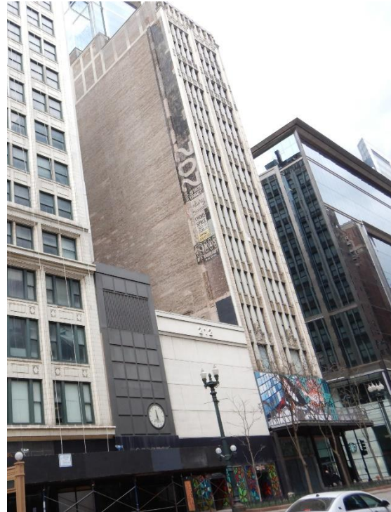
Photo 4. South and east elevations.
