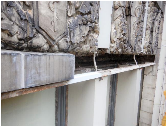
Photo 45. Exploratory opening at 13th floor window headers, north elevation.
