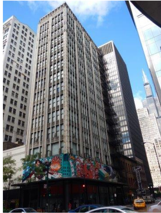
Photo 2. East and north elevations.
