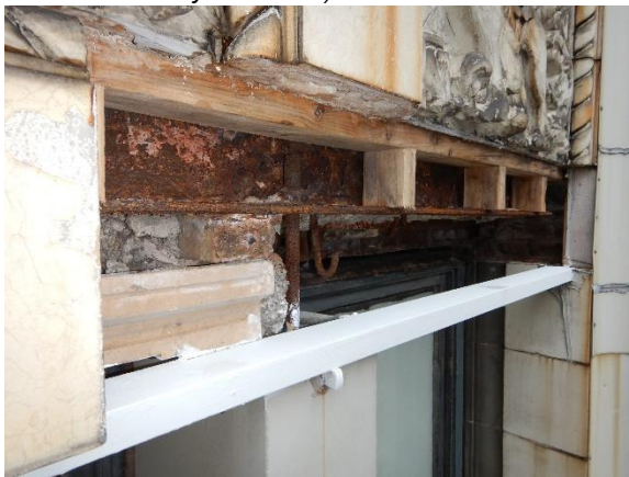
Photo 49. Exploratory opening #2 at attic floor window headers, north elevation.
