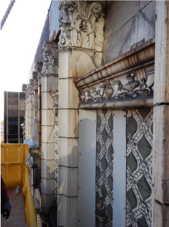
Photo 5. Lower portion of cornice throughout north and east elevations.
