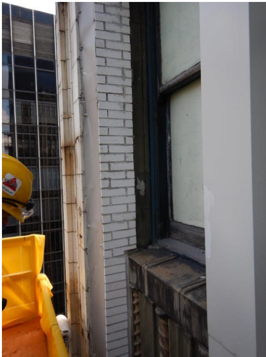
Photo 29. Replacement of terra cotta units with brick masonry.
