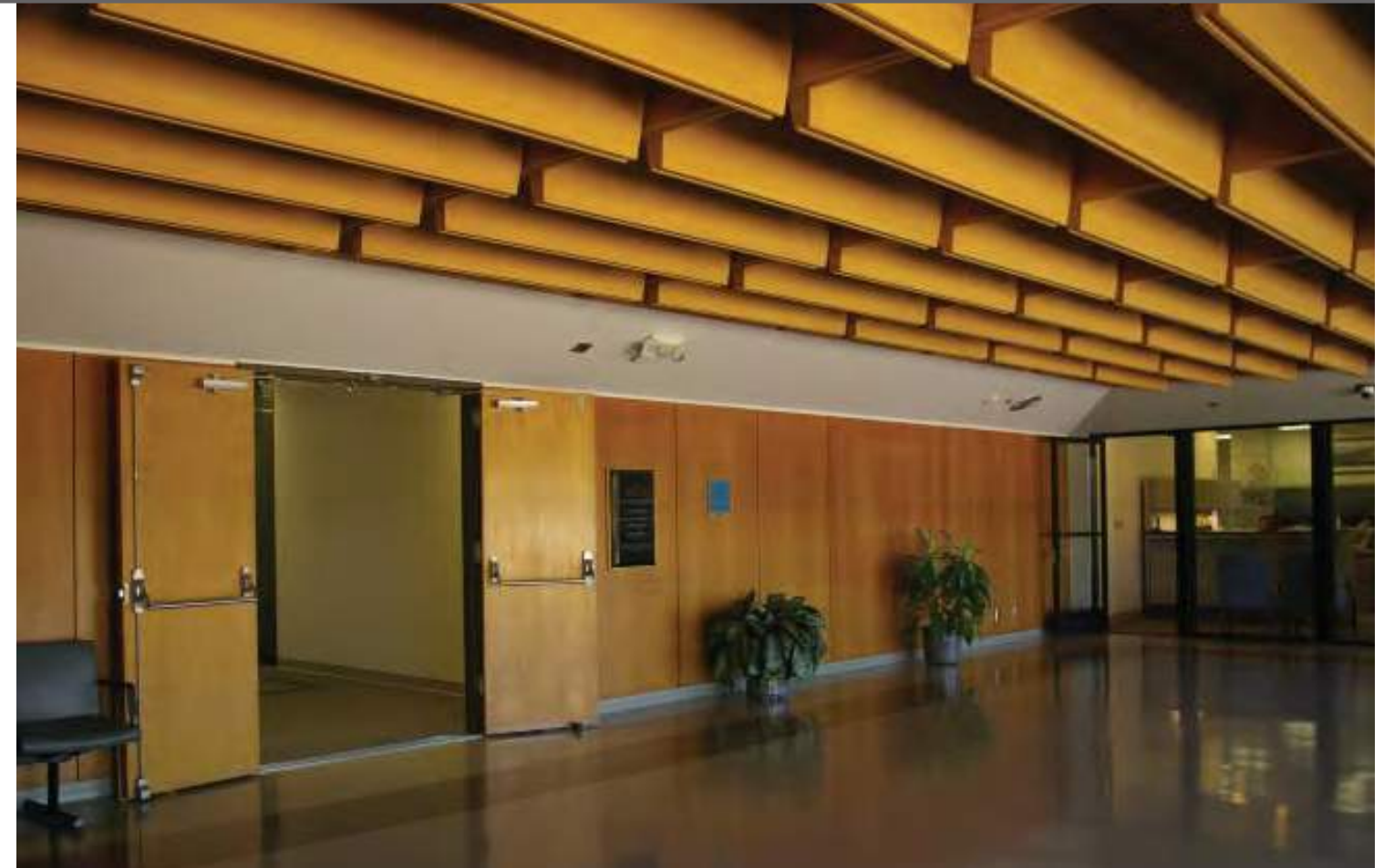
4th Floor lobby
