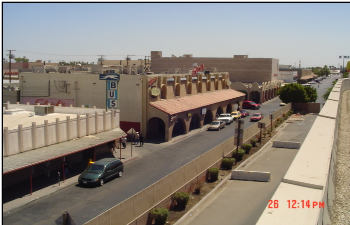
Figure 3.4-2. View looking northeast along First Street from the Main LPOE Building.
