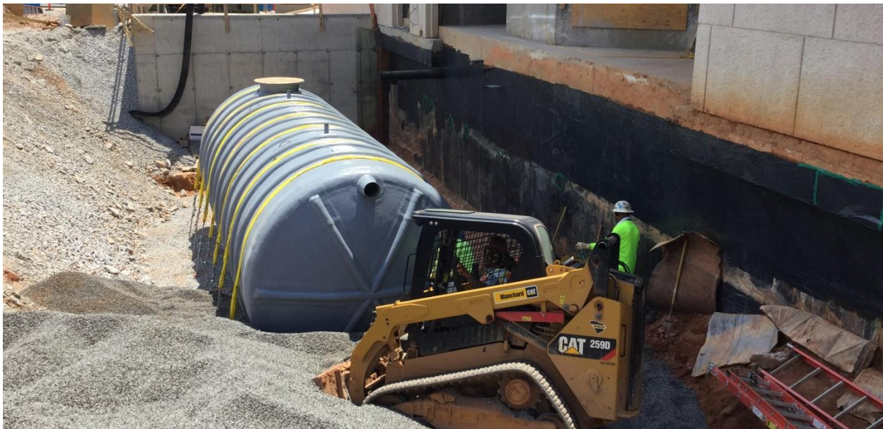
Installation Photo of the Irrigation Cistern
