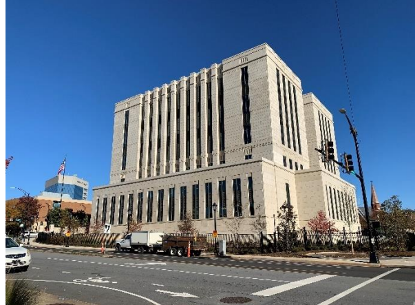
After: Completed construction
