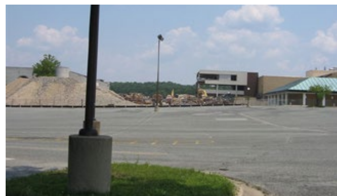
Landover Mall during Demolition (2006).
