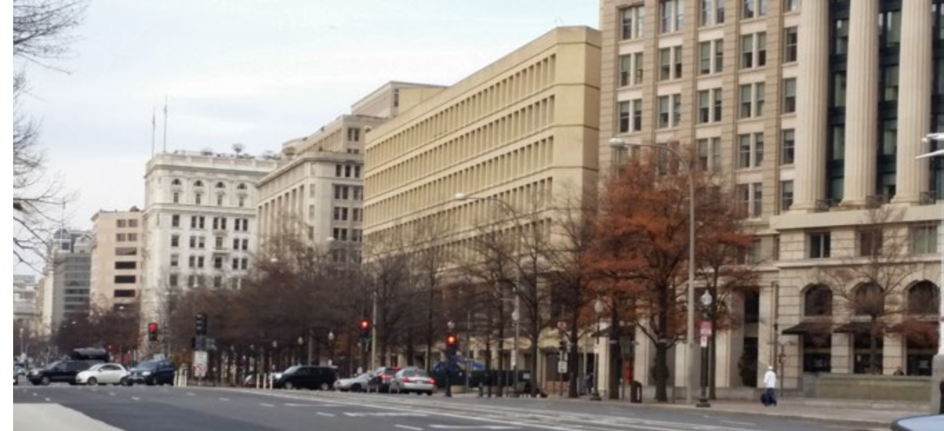
View of JEH building from archives building, looking northwest
