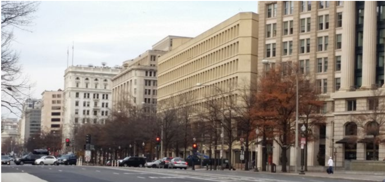
View of JEH from National Archives Building along Pennsylvania Avenue NW
