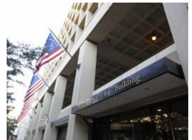
Entrance to the JEH building
