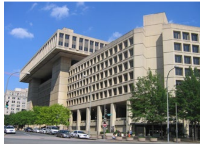
The existing JEH building
