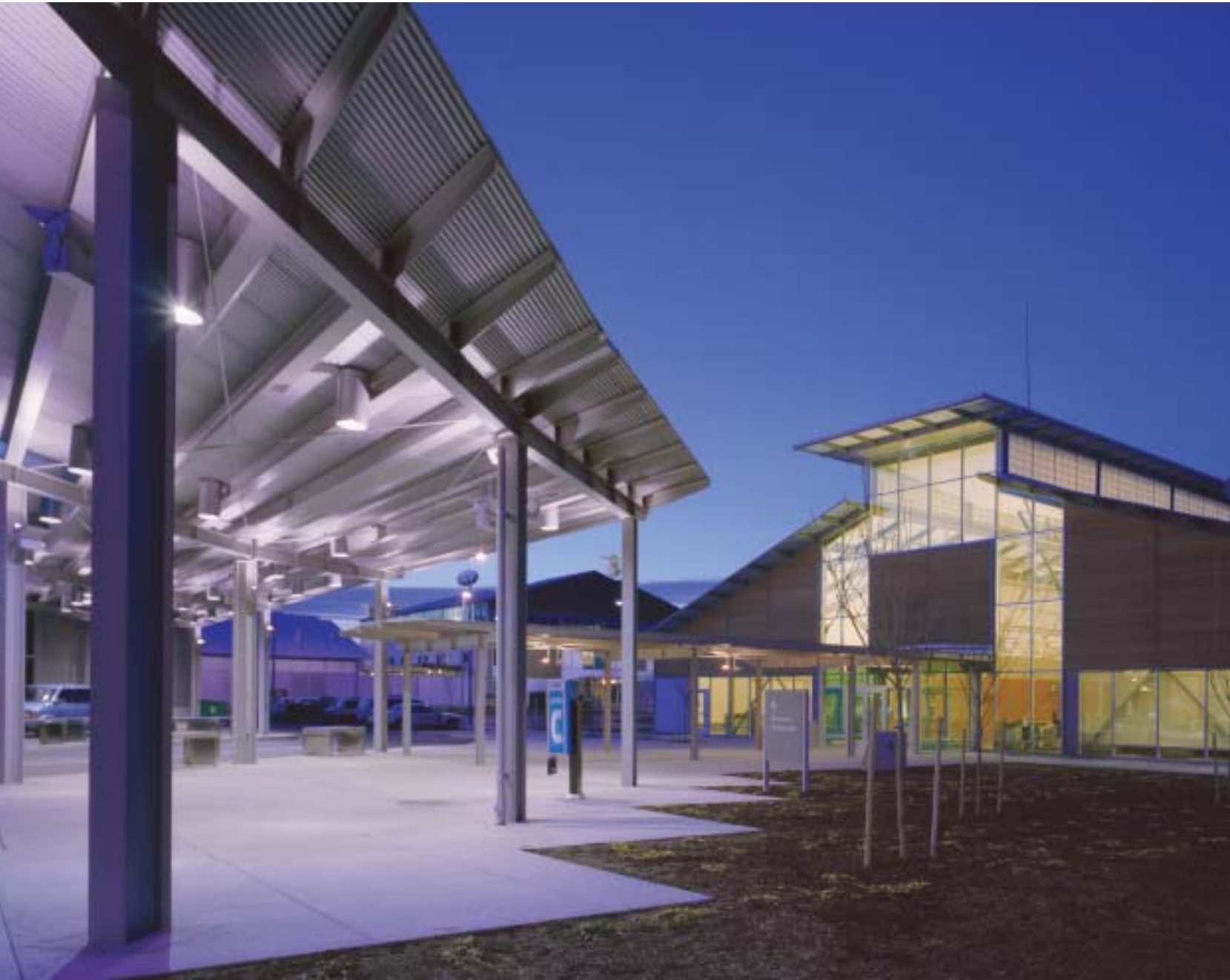
THE COMBINATION OF WOOD SIDING AND CORRUGATED METAL GIVES THE STRUCTURE A REGIONAL MOOD AND MODERN LEGIBILITY. / JURY COMMENT
