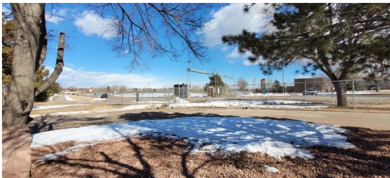
PHOTO 3. VIEW TOWARDS THE SOUTHEAST FIELD FROM BUILDING 710.
