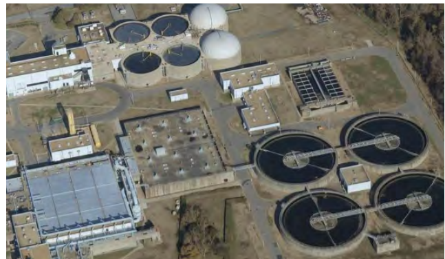
The HRSD Treatment Plant, whose effluent pipeline was used in the Dam Neck GSHP system image courtesy of: Trane U.S., Inc.
