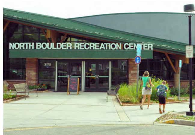
The North Boulder Recreation Center was a key building in the portfolio
