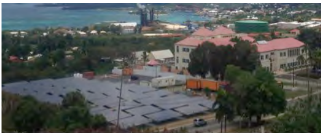
Almeric L. Christian Federal Building image courtesy of: Schneider Electric
