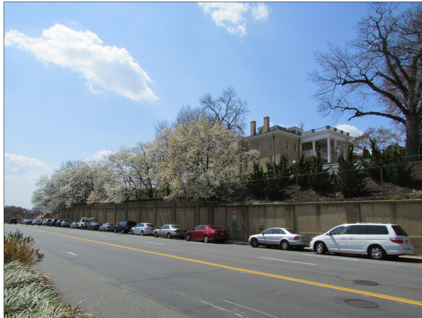
23rd Street Retaining Wall
