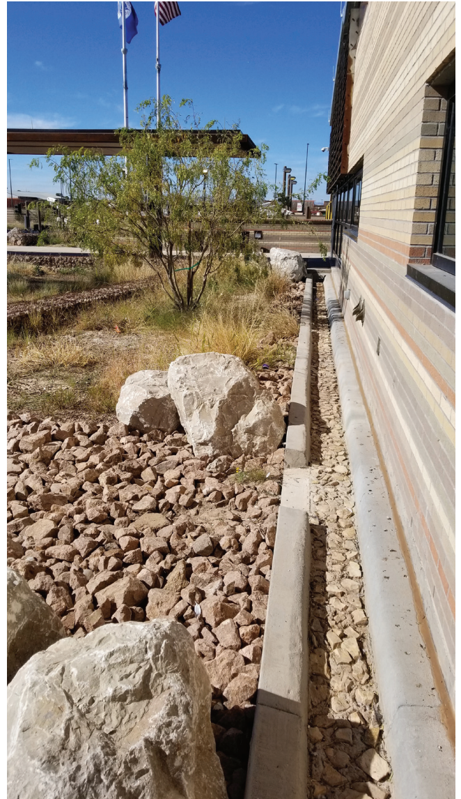
The runnel collects roof runoff, distributing it to water harvesting terraces. Photo by Aaron Zahm.
