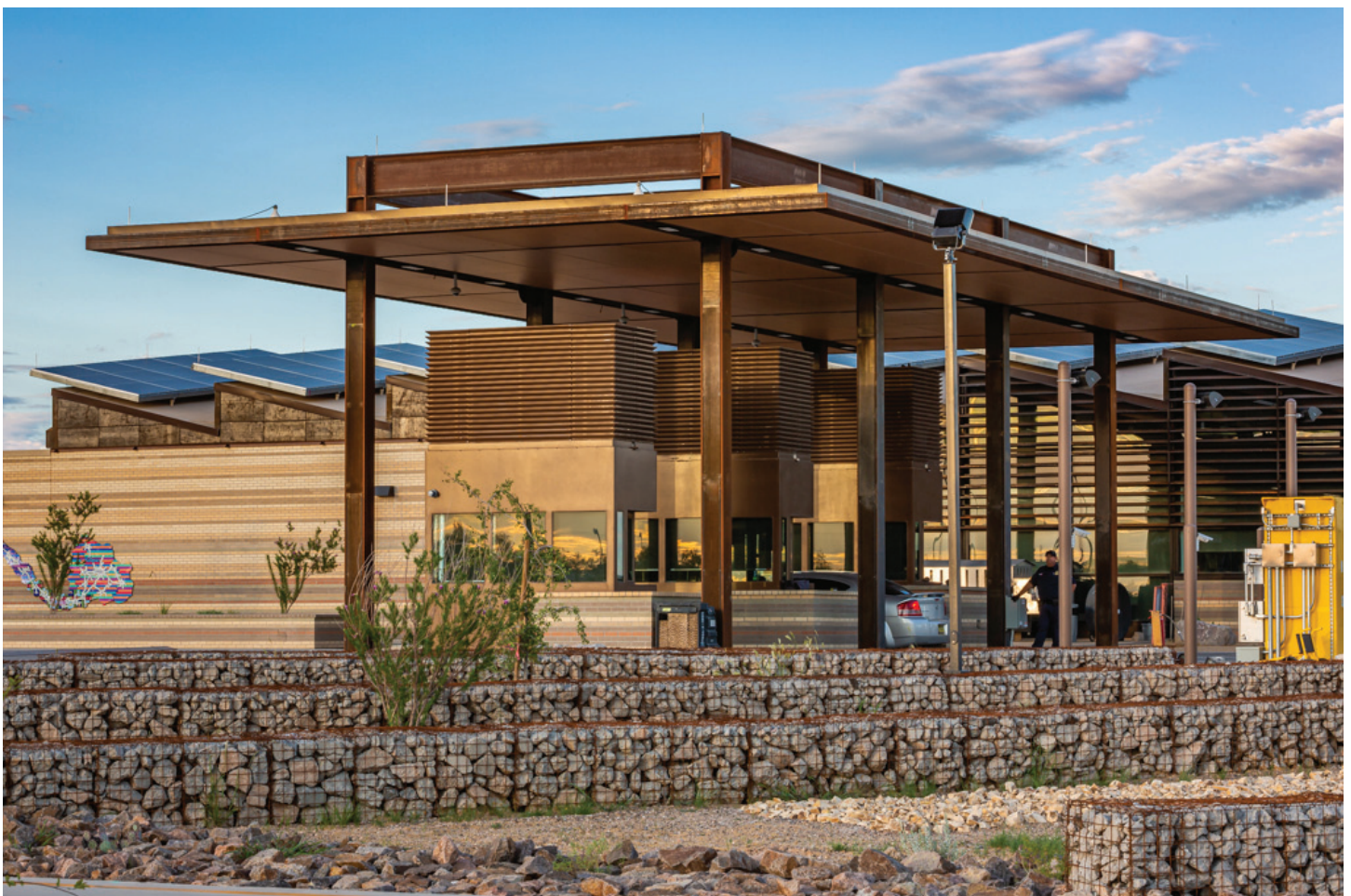
Salvaged concrete reused for gabion fill material. Photo by Robert Reck.
