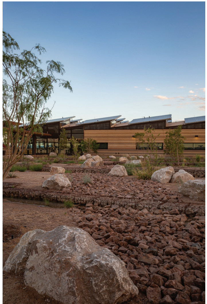
A desert wash carries roof runoff through the landscape. Photo by Robert Reck.
