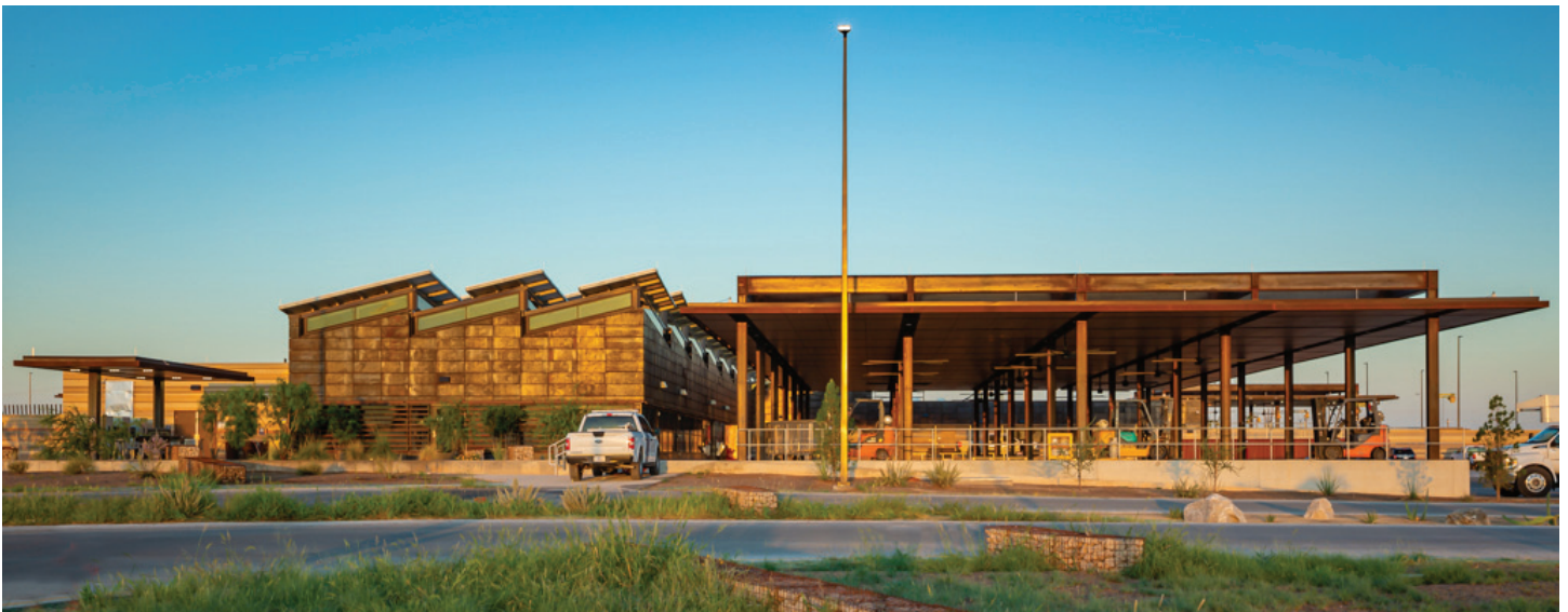
Restored grasslands east of the main building. Photo by Robert Reck.
