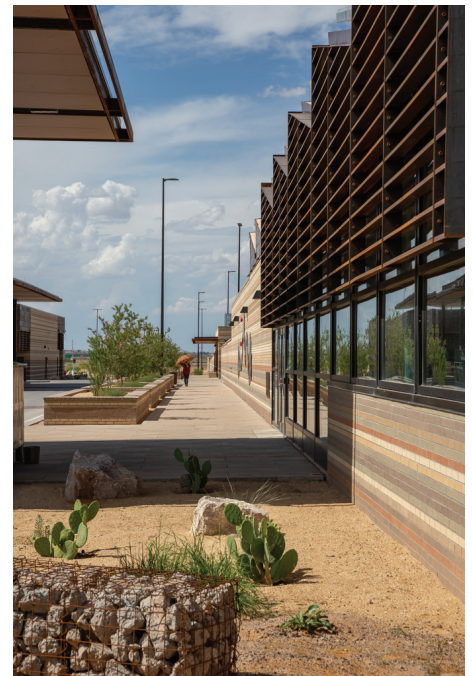
Gabion wall and planters along the west side of the main building. Photo by Robert Reck.
