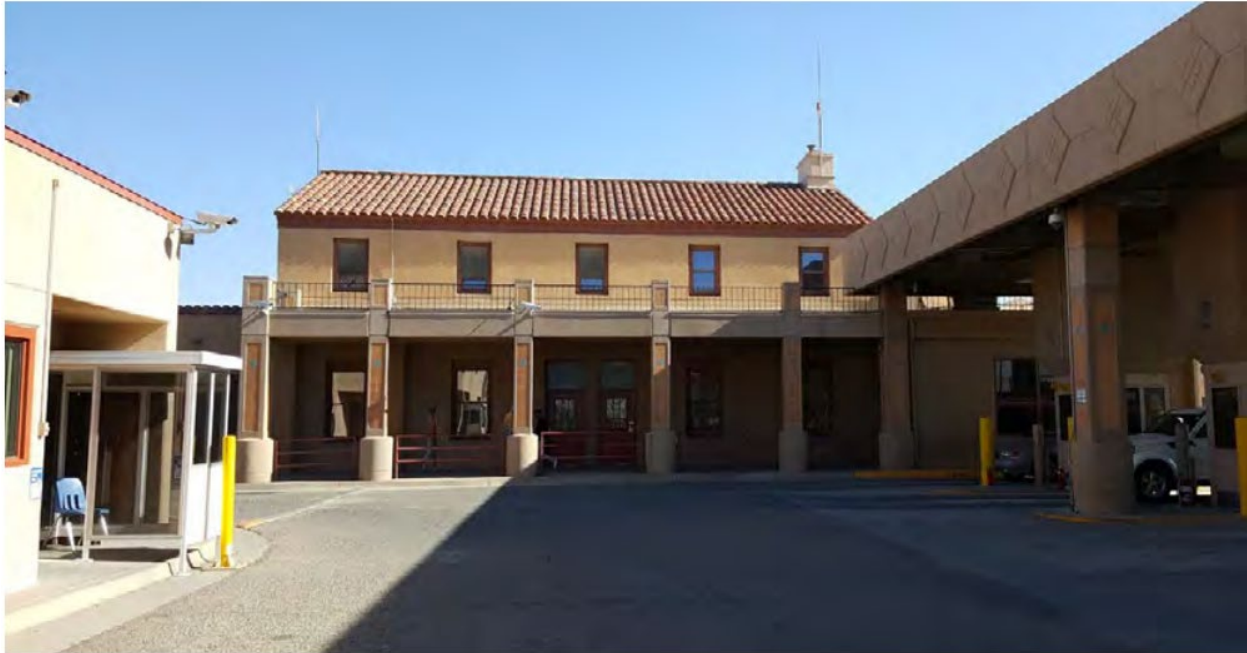
Figure 1-5. Historic Main Building – West Facade
