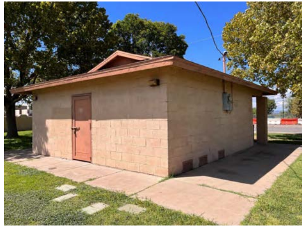
Rear and northern façade
