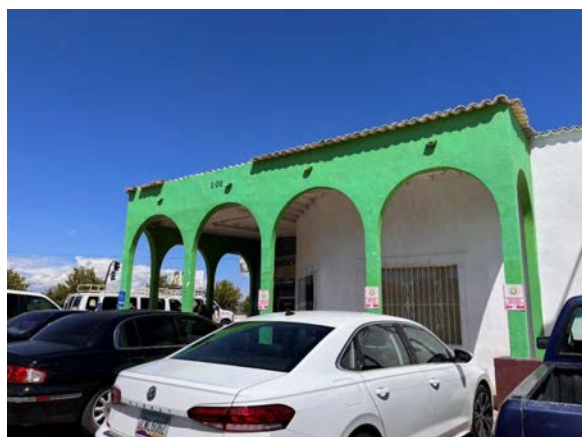
Façade facing parking lot
