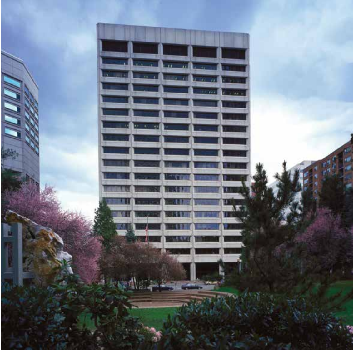
View of building before renovation
