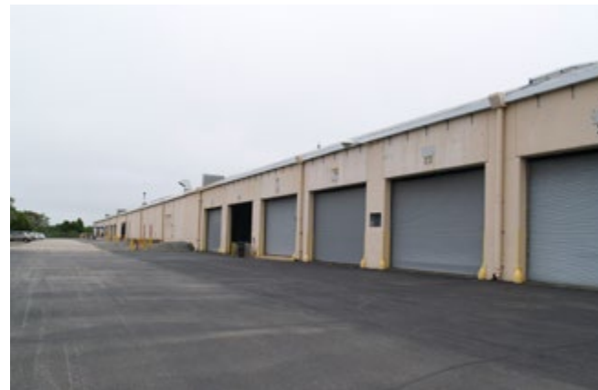
GSA Franconia Warehouse Complex - Building A
