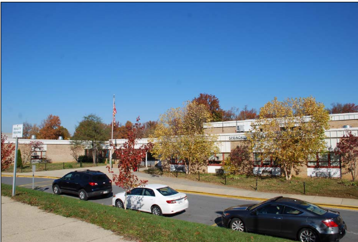
Figure 8. Greenbelt Site, Springhill Elementary School
