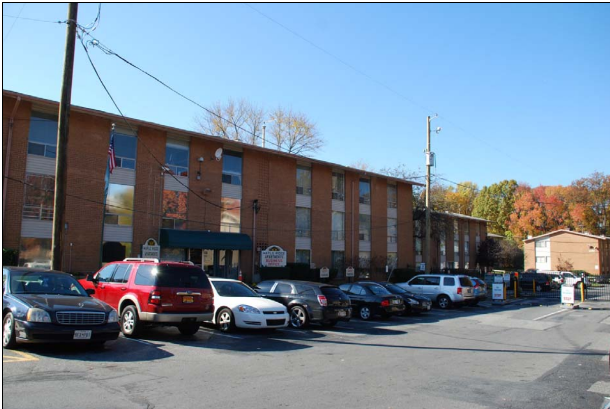
Figure 2. Landover Site, Maple Ridge Apartments (formerly Village in the Woods)
